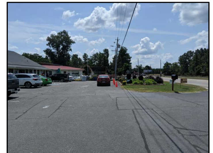
View of Survey Area (Facing Approximately South)
