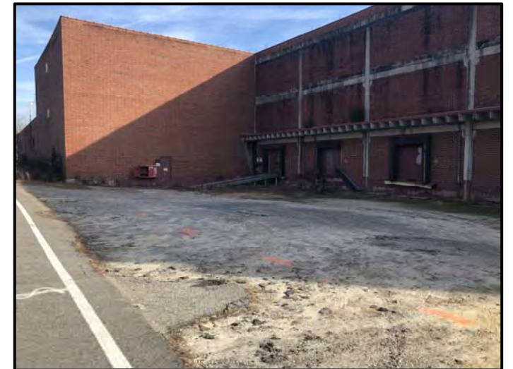
View of Northwest Survey Area (Facing Approximately Southwest)
