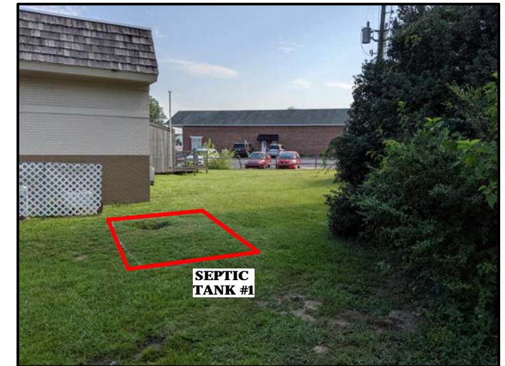
View of One Septic Tank Facing Approximately North
