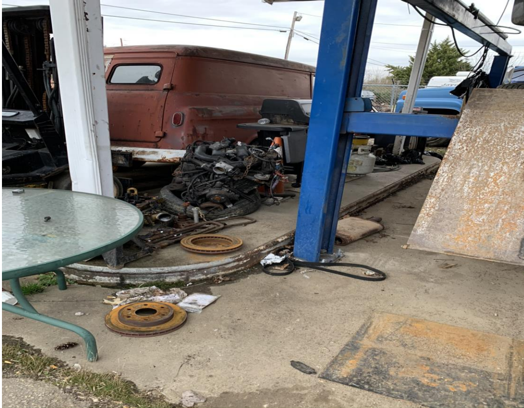
Former UST dispenser area 1
