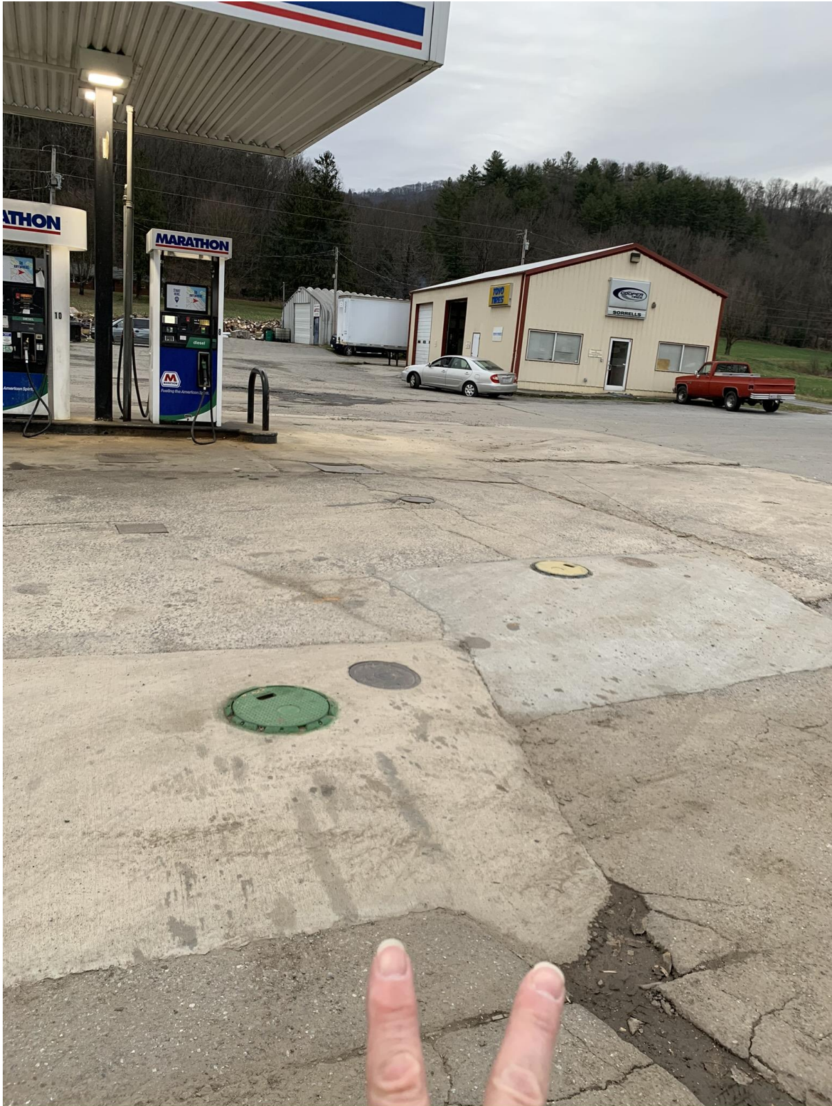
UST area 2. Noted the remediation wells (the square metal covers) in the area.
