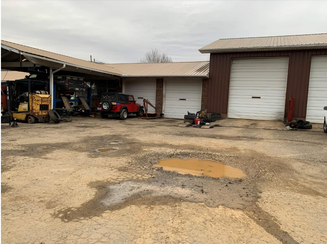
Possible former UST area.
