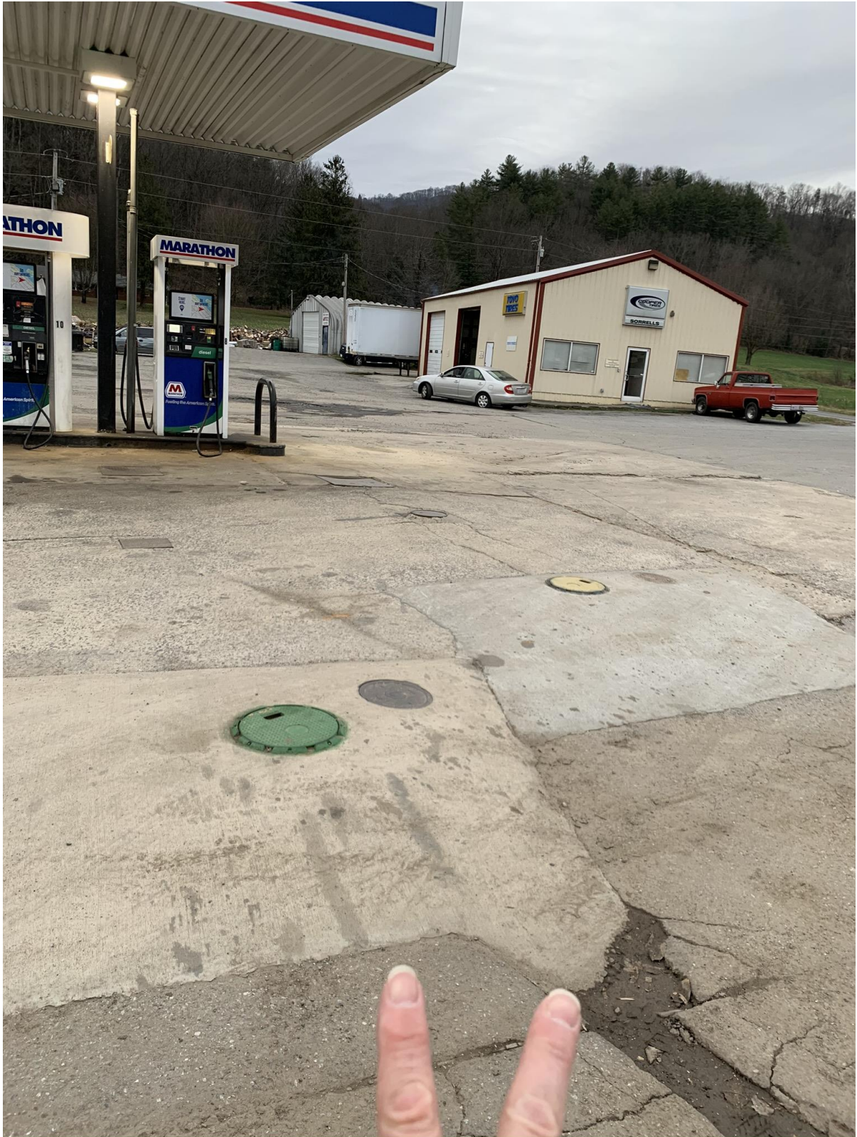
UST area 2. Noted the remediation wells (the square metal covers) in the area.
