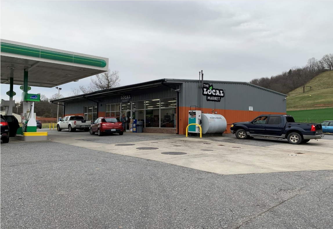
UST area with an AST at the corner of the building
