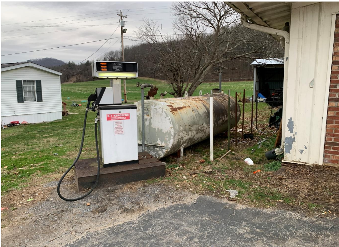
AST at the corner of the building.
