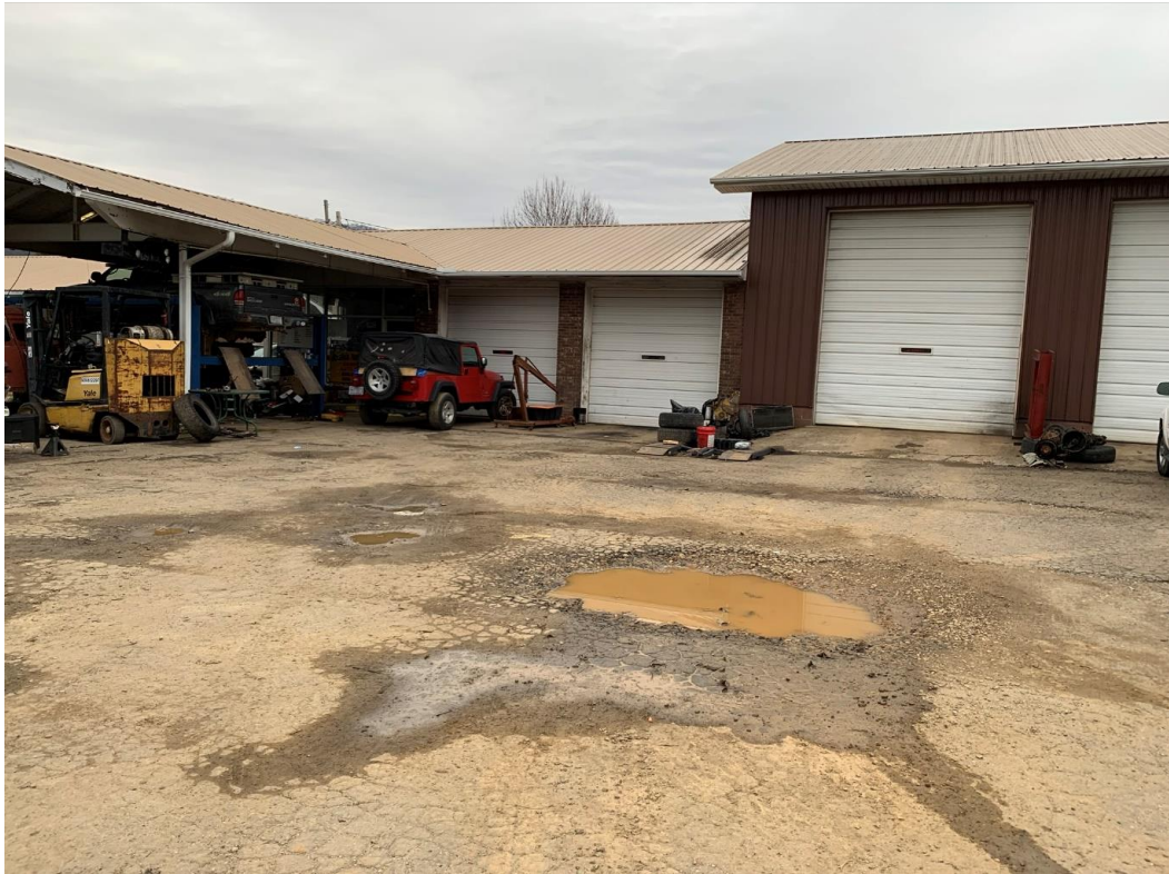
Possible former UST area.
