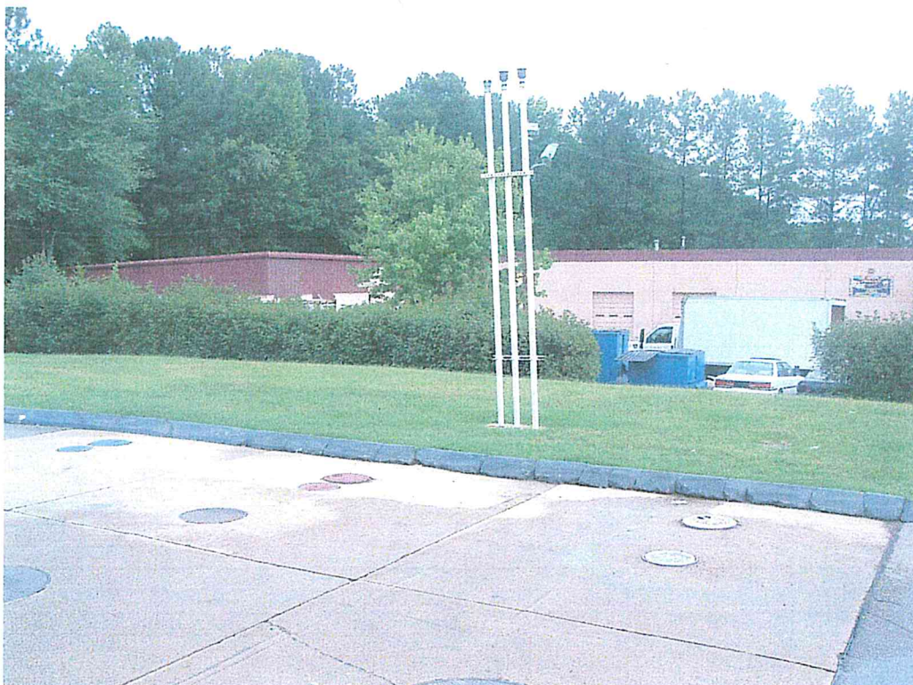
Underground Storage Tanks and Vent Pipes at Adjacent Quality Mart
