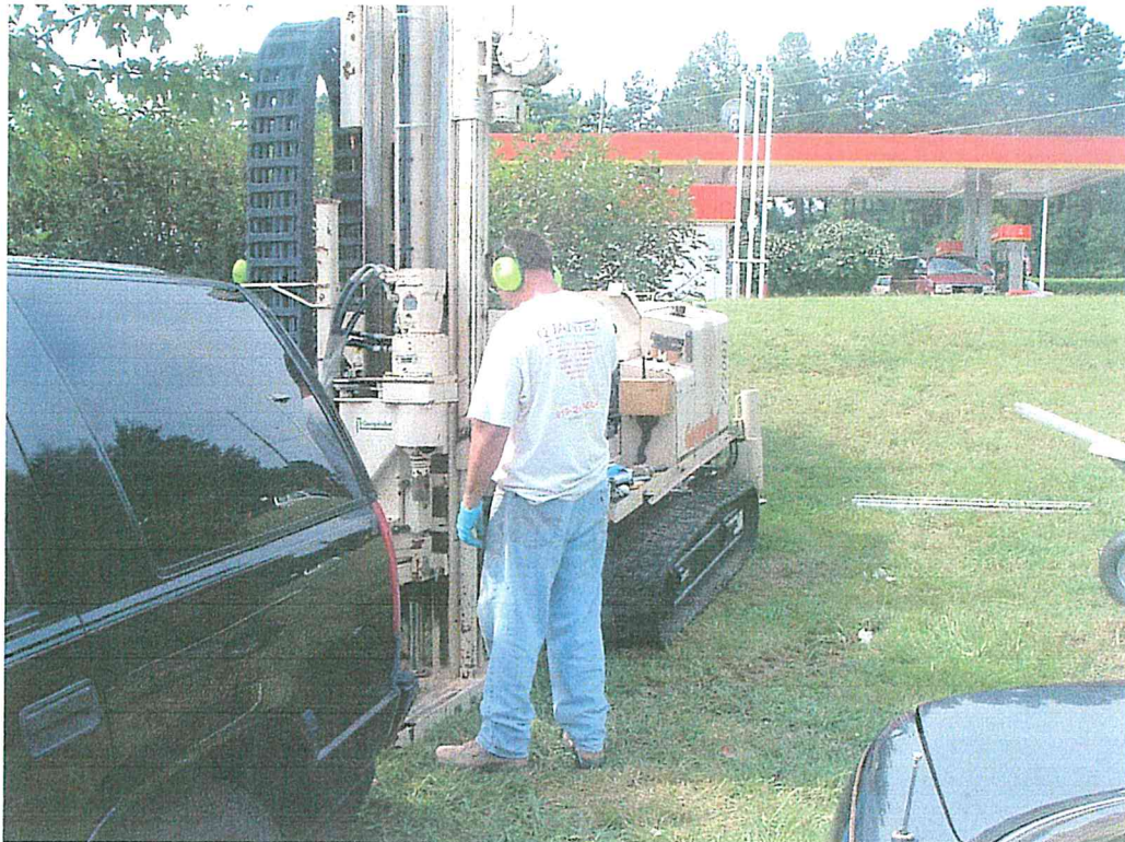
Location of Samples Nos. GW-3 and S-3 (Gas Station UST Vent Pipes in Background)
