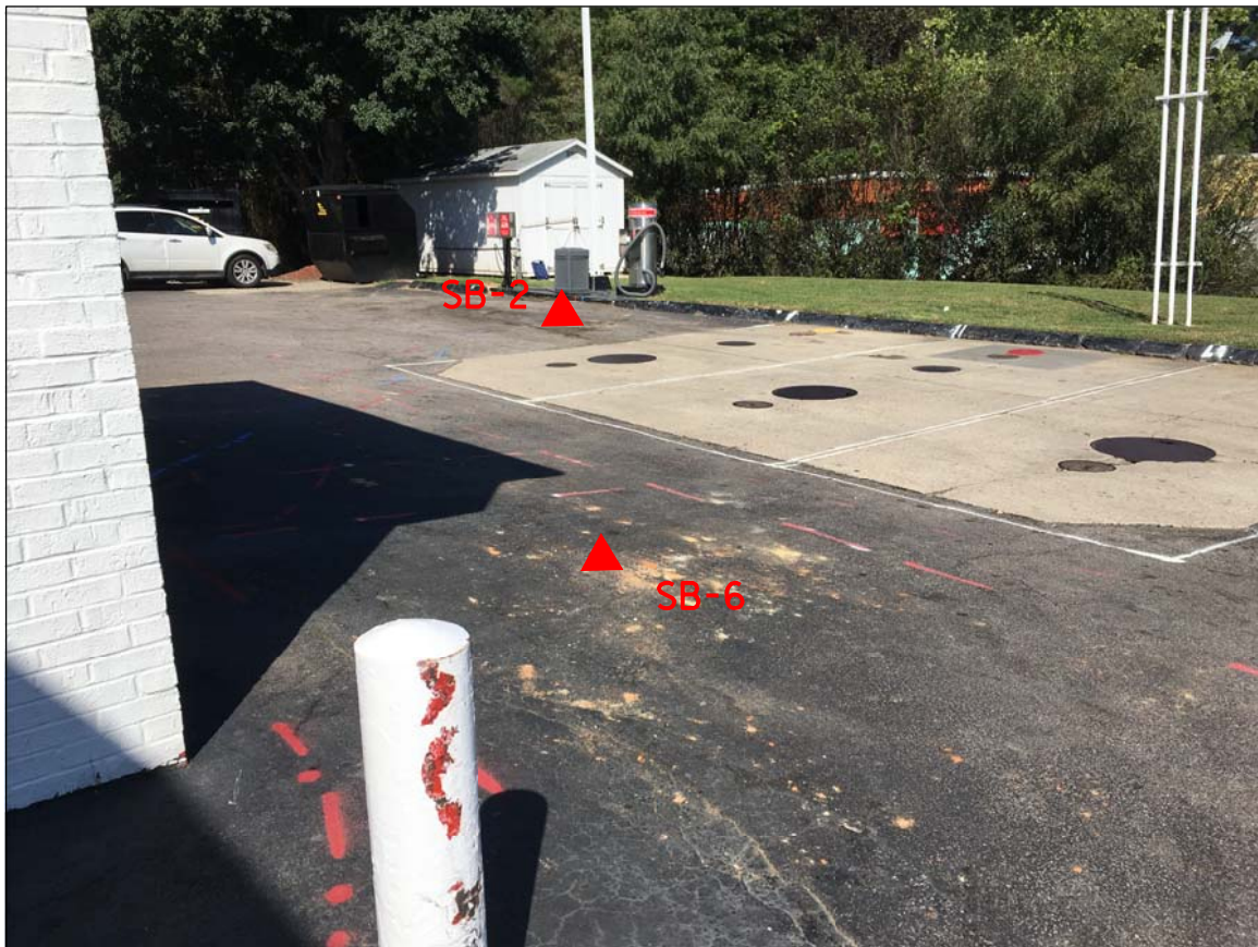
PHOTO 6 - VIEW OF SOIL BORING LOOKING NORTHWEST
