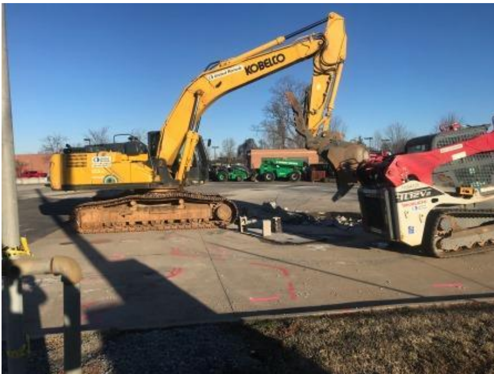
Photograph 2: CCI removing concrete over USTs.
