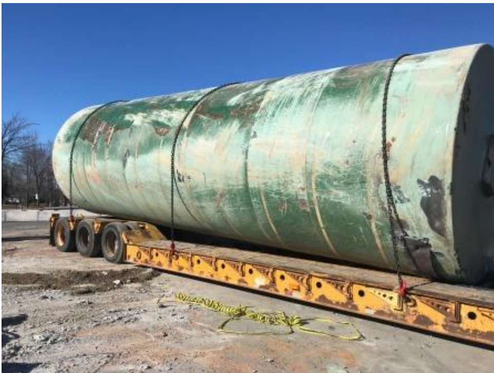
Photograph 6: UST-1 removed from UST basin.
