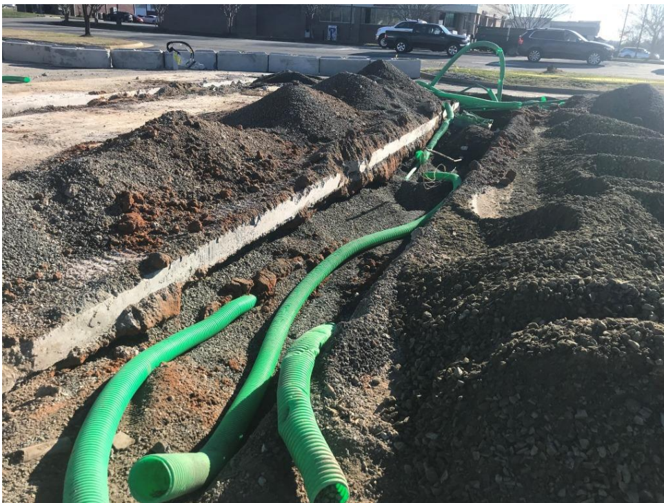
Photograph 16: Product line trench exposed.
