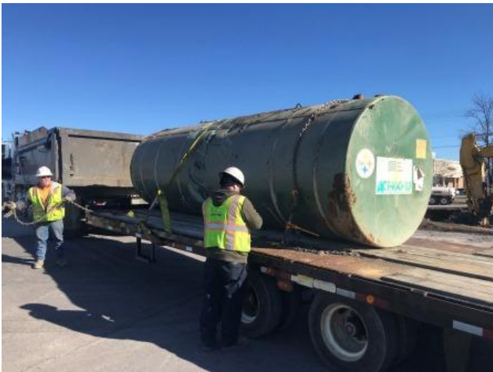
Photograph 4: UST-3 removed from UST basin.
