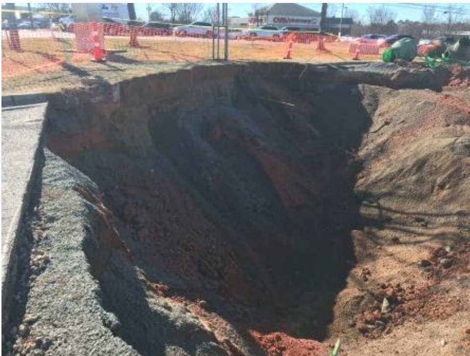
Photograph 8: Open excavation after UST removal.
