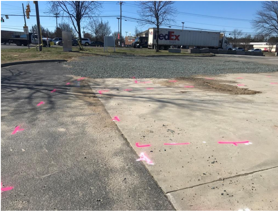
Photograph 11: Product line trenches outlined by private utility locator.
