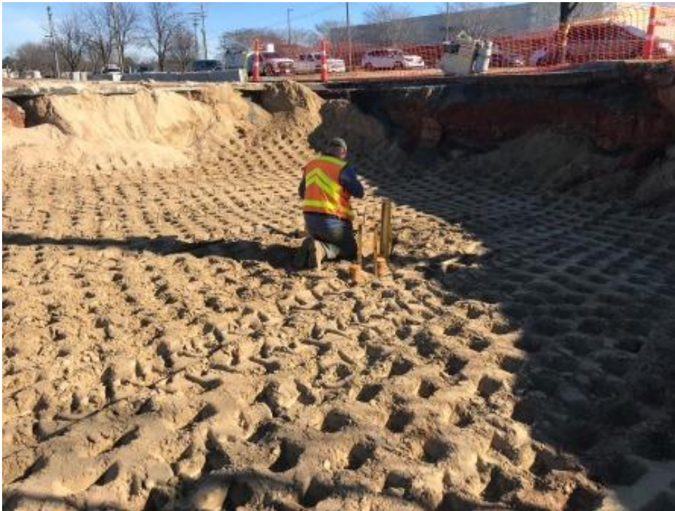
Photograph 9: NCDOT performing compaction testing.
