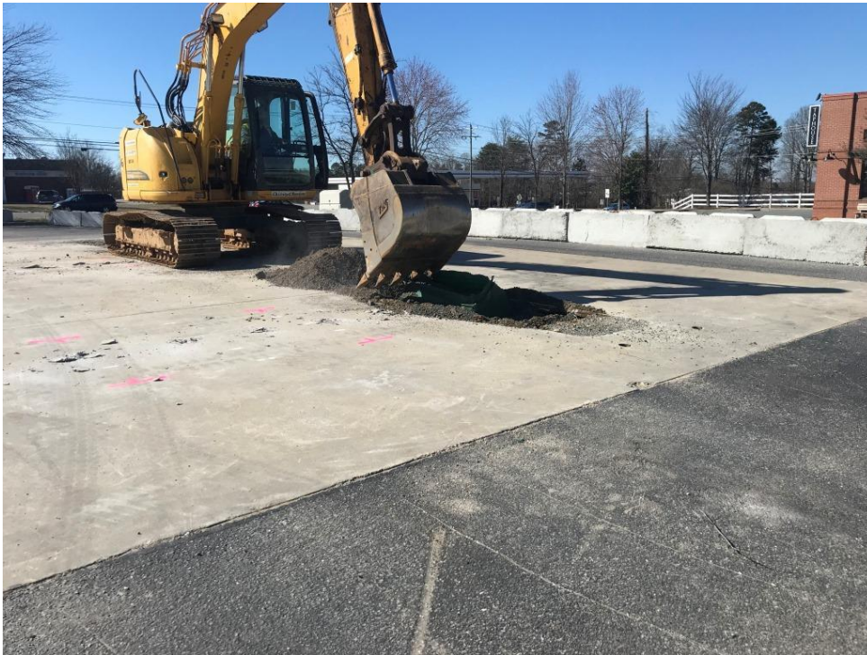
Photograph 13: CCI removing a spill bucket.
