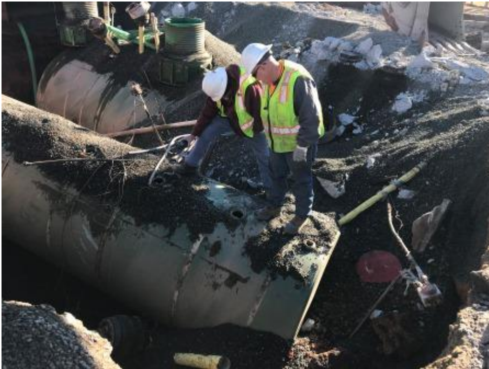
Photograph 3: CCI using a LEL meter to check gas levels before removing.
