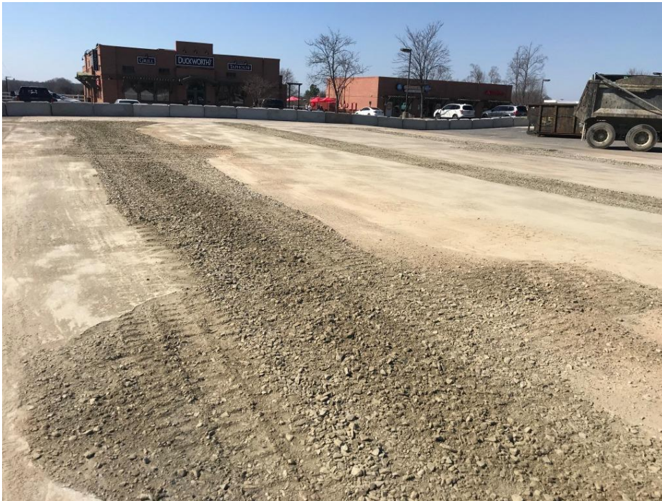
Photograph 17: Product line trenches backfilled and covered with ABC stone.
