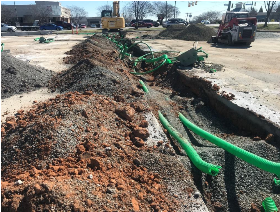
Photograph 15: One product line trench exposed.
