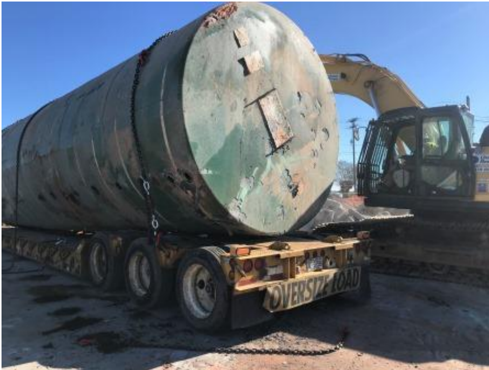
Photograph 7: UST-2 removed from UST basin.
