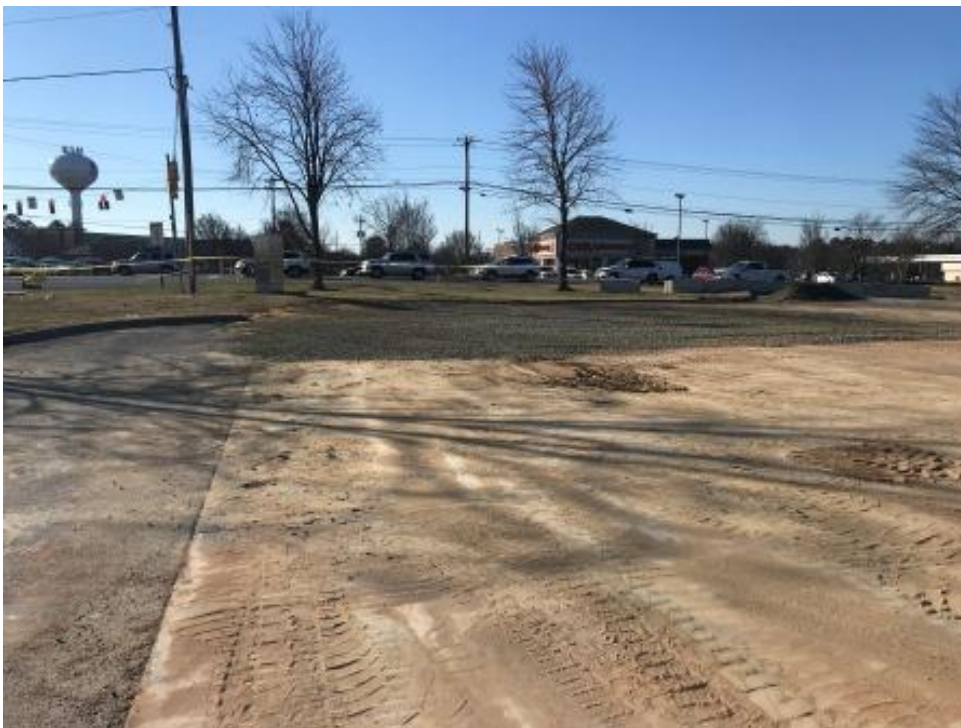
Photograph 10: Excavation backfilled, compacted, and topped with ABC stone.
