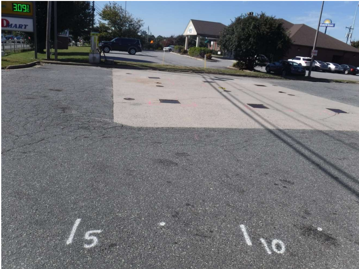
Photo 3: Showing known USTs
