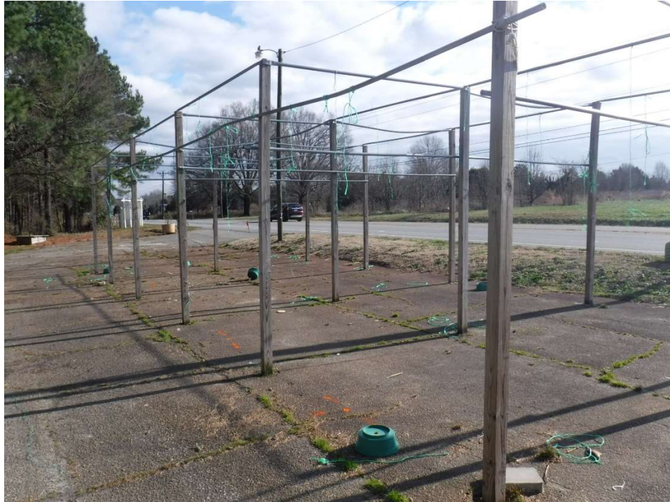
Photo 7: Looking southeast showing “Metal frame with netting”
