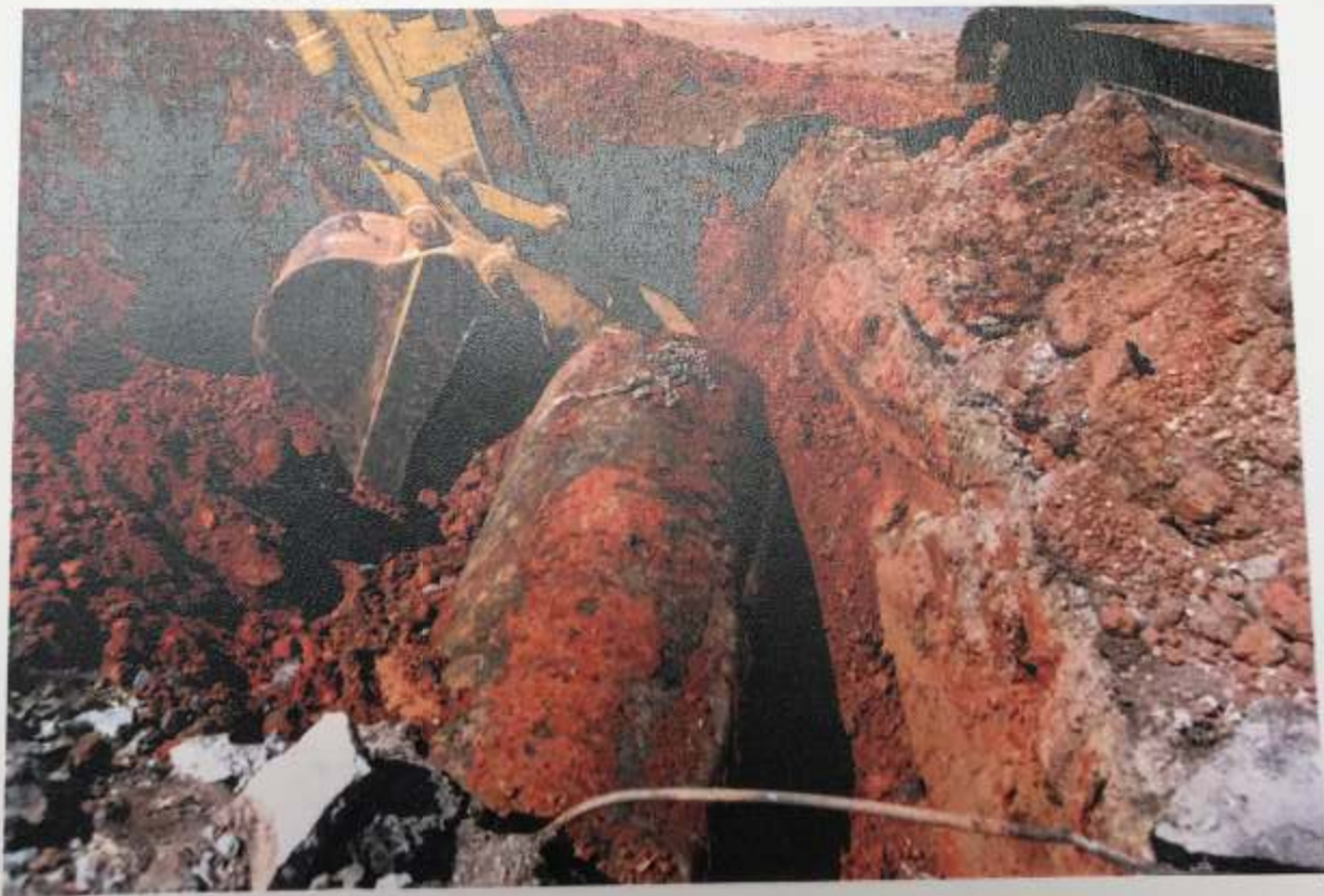
Photograph 7: Tank S-4 (Kerosene) Excavation
