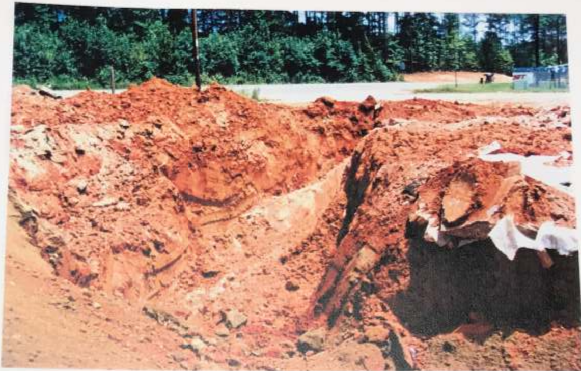
Photograph 6: Product Lines and Dispenser Excavation
