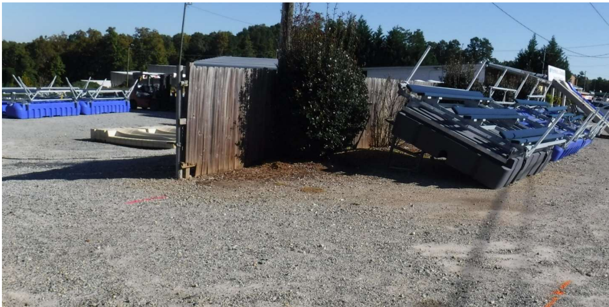
Photo 1: Looking east showing surface metal and obstructions
