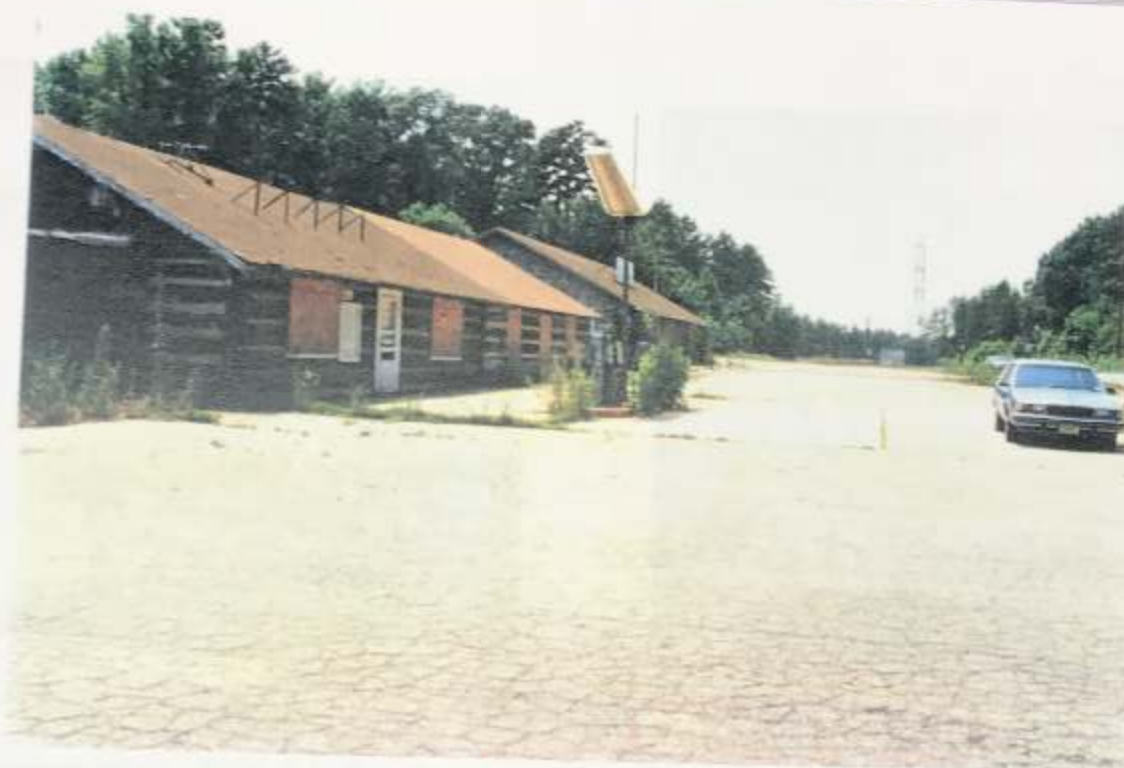
Photograph 1: General Site Conditions Prior to Excavation
