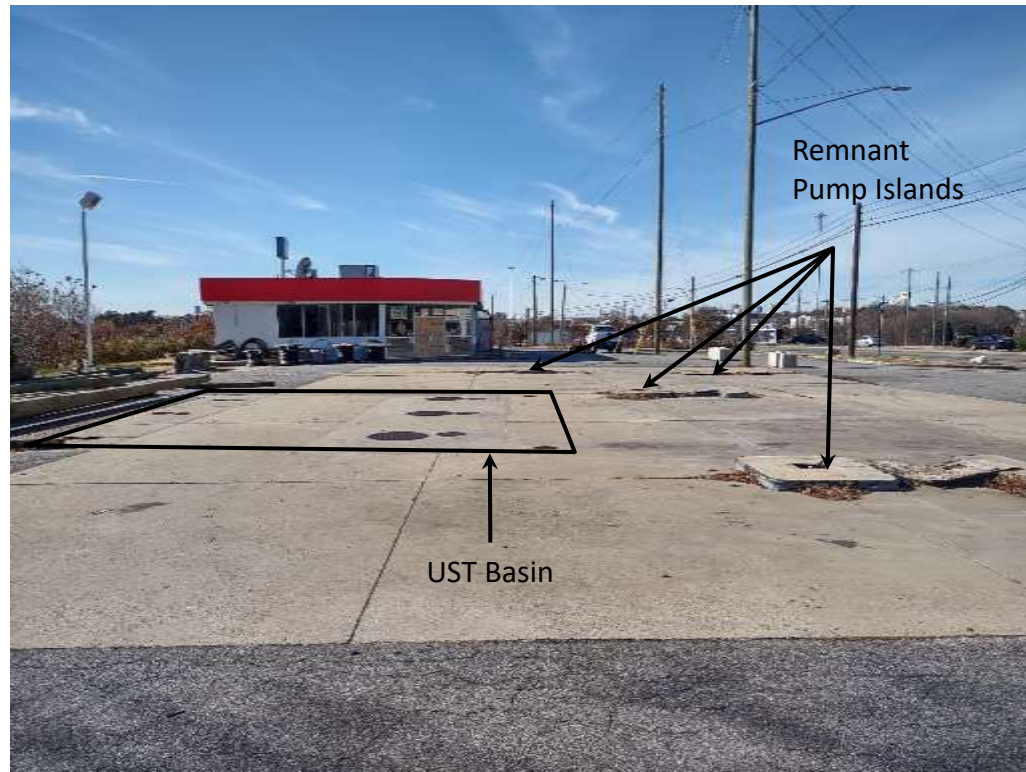
C. Photograph of the east side of site showing UST basin and remnant pump islands, facing west.
