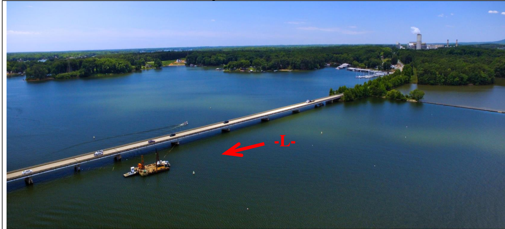
Looking southwest towards End Bent 1
