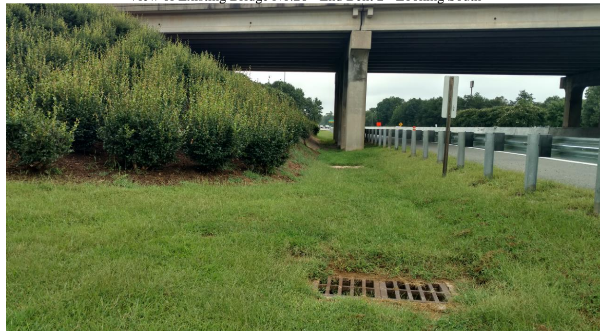
View of Existing Bridge No.26 - End Bent 2 - Looking South
