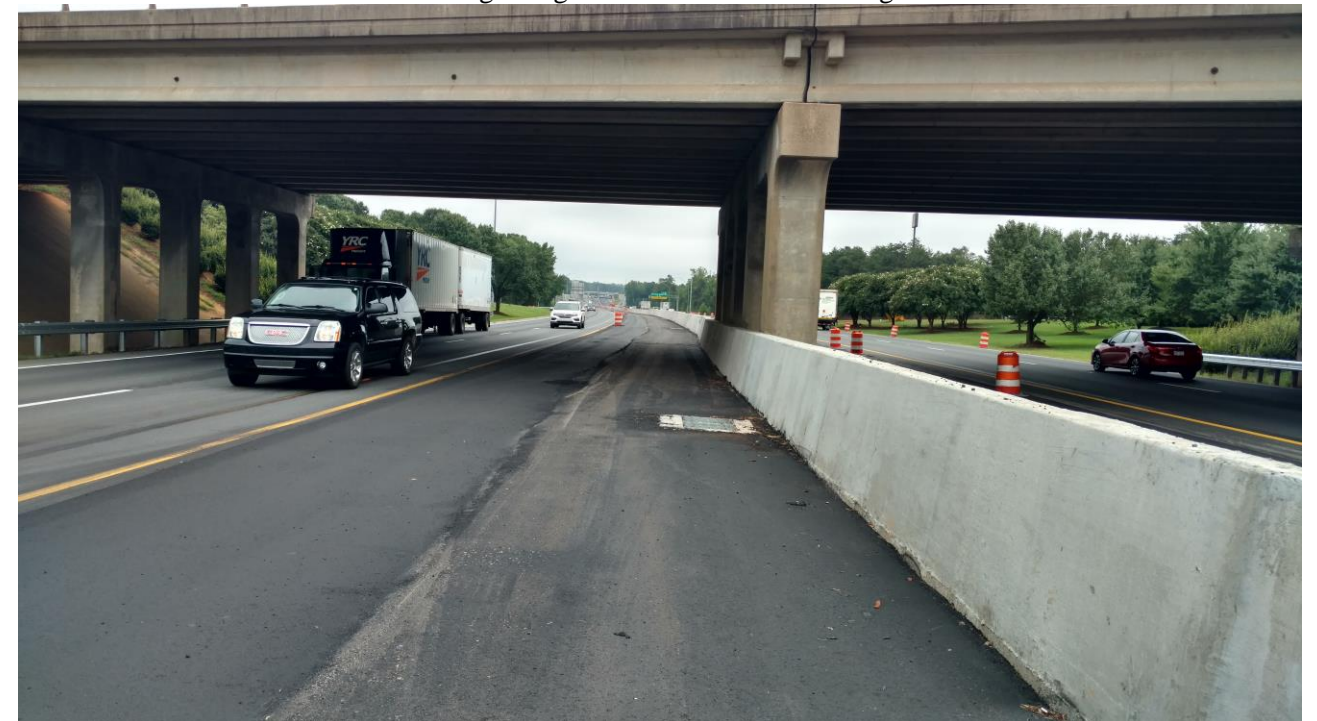
View of Existing Bridge No. 26 - Bent 1 - Looking South
