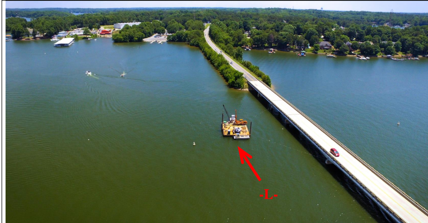
Looking east towards End Bent 2
