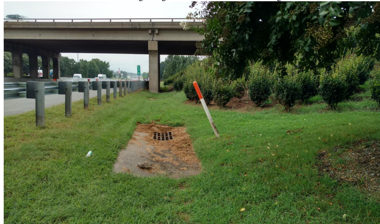
View of Existing Bridge No.26 - End Bent 1 - Looking South
