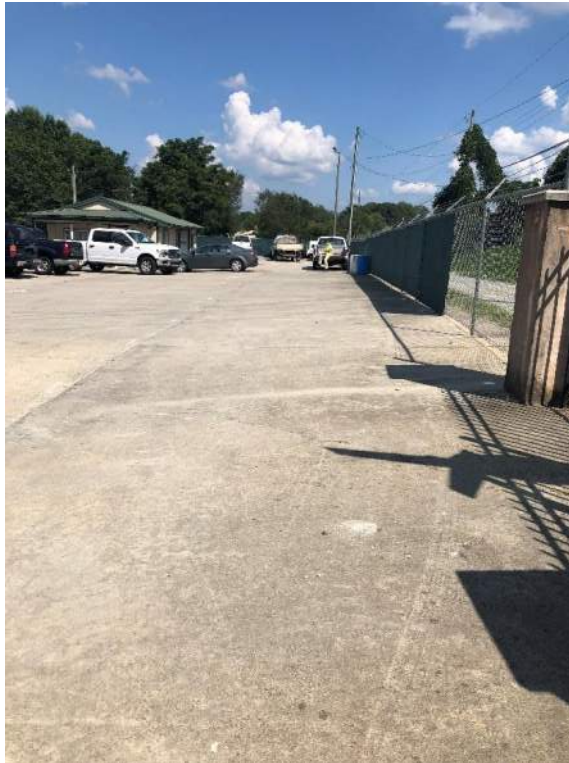
View facing east away from Winston Road on Parcel 50.
