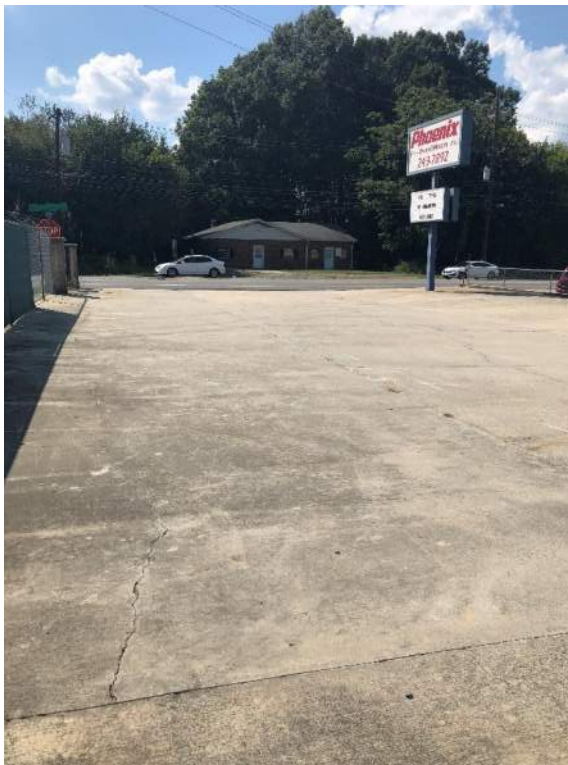
View facing westerly toward Winston Road on Parcel 50.
