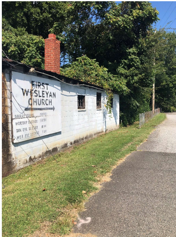
View facing easterly along the southern boundary of Parcel 46.
