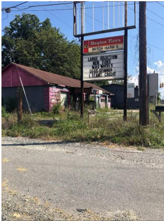
View facing southeast toward the former service station on Parcel 47.
