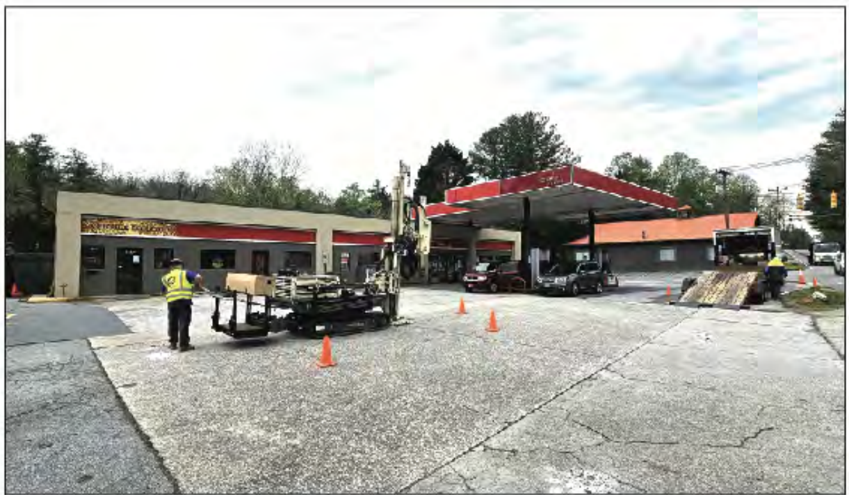
Photo 1. View to the southwest across Parcel #019. Geoprobe is drilling boring B-5.
