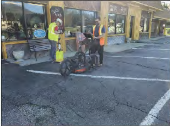
Photo 2. Collecting GPR data at Parcel #019B.
