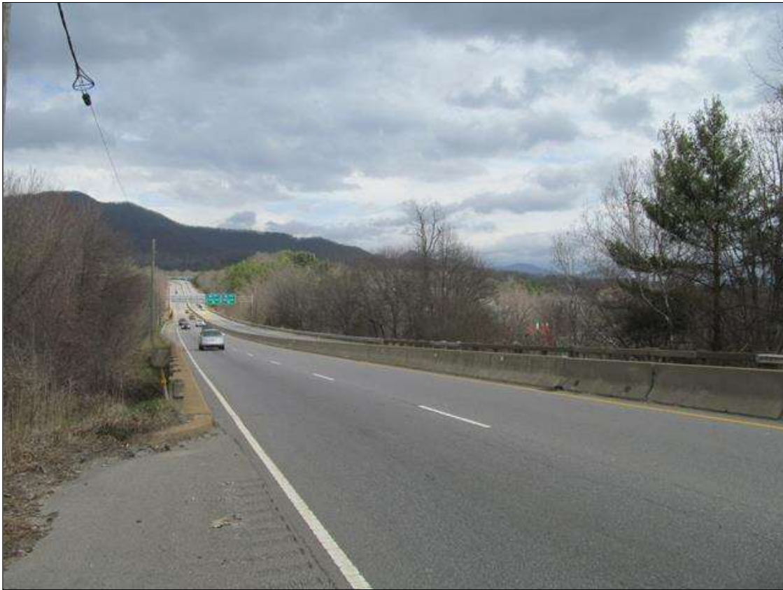
SOUTH APPROACH, SBL
