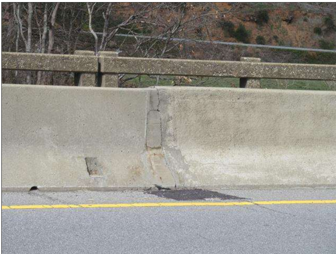
SOUTH APPROACH, TRANSITION FROM RC BARRIER TO RC MEDIAN RAIL. NORTH APPROACH IS SIMILAR.
