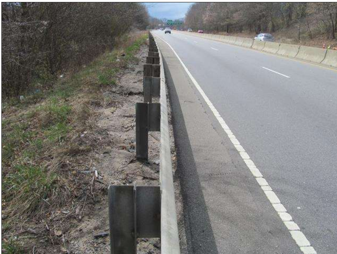
SE CORNER, GR TIED TO EXTENDED RAIL RUN
