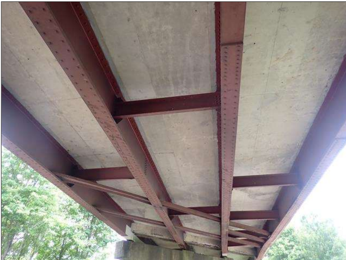
SPAN 2 UNDERDECK, OTHERS SIMILAR
