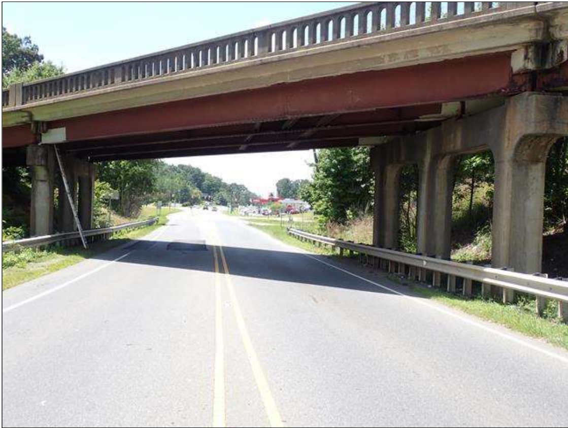
SPAN 2 EAST PROFILE, LOOKING WEST
