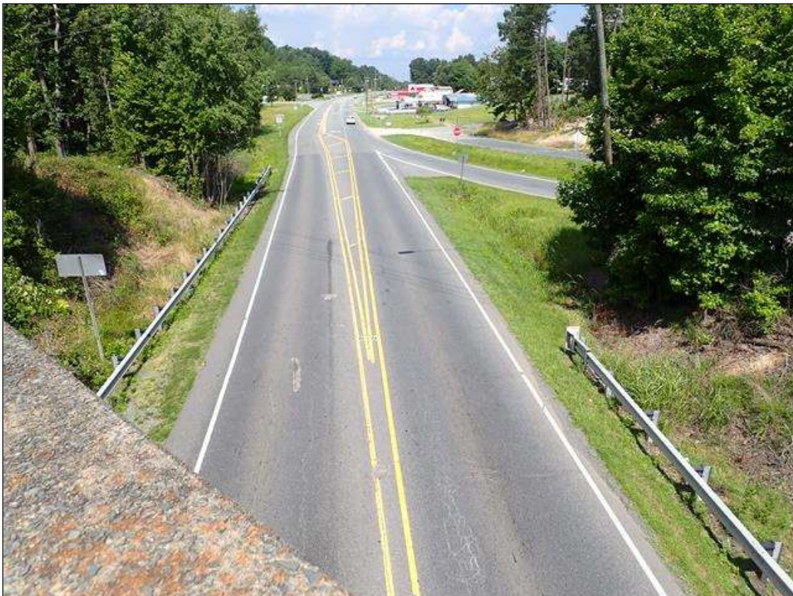
LOOKING WEST FROM SPAN 2
