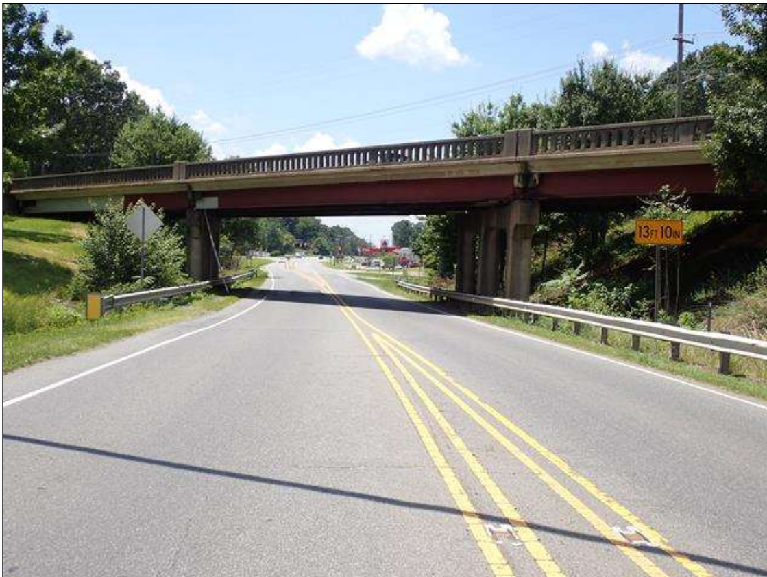
EAST PROFILE, LOOKING WEST
