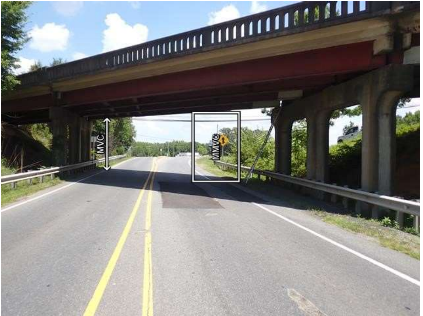
SPAN 2 WEST PROFILE, LOOKING EAST
