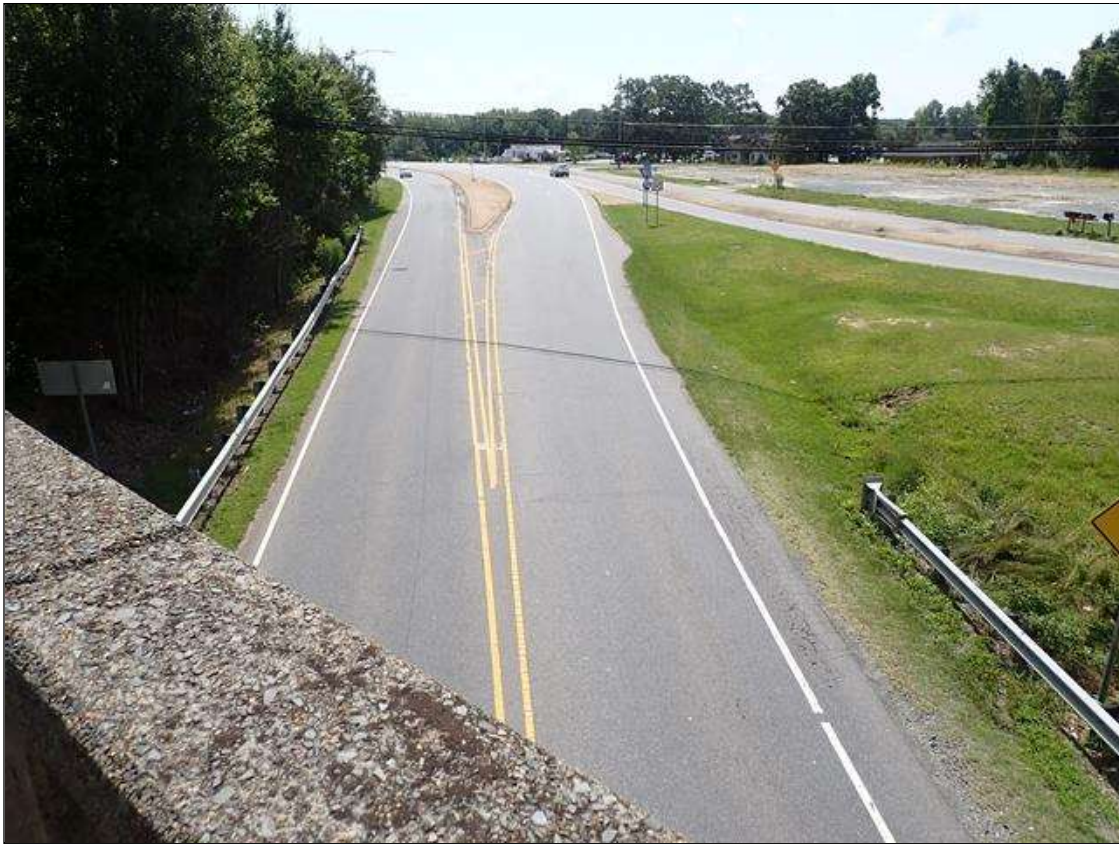
LOOKING EAST FROM SPAN 2
