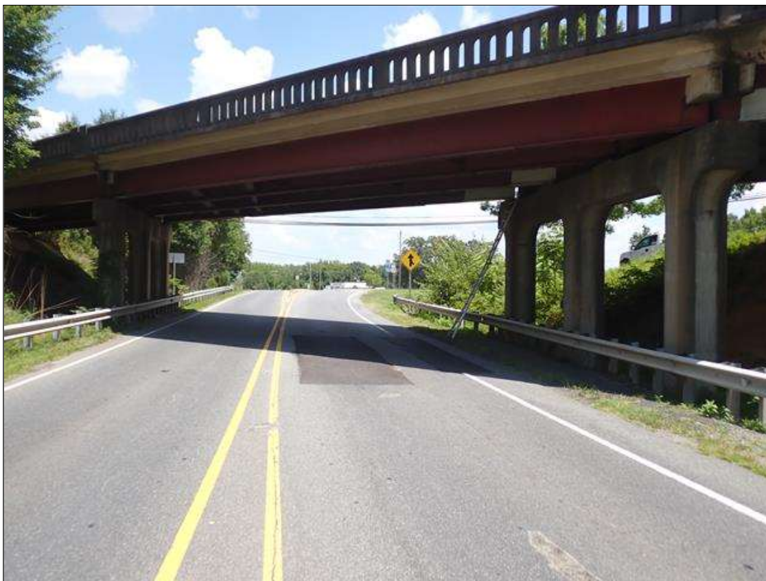
SPAN 2 WEST PROFILE, LOOKING EAST
