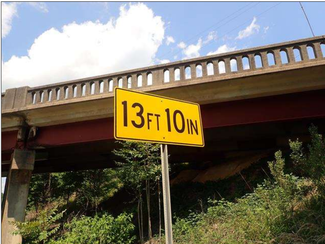
CLEARANCE SIGN, APPROXIMATELY 25 FEET EAST OF BENT 2
