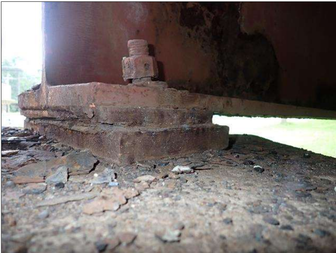
SPAN 1 BEAM 4 BEARING AT BENT 1, OTHERS SIMILAR AT BENTS
