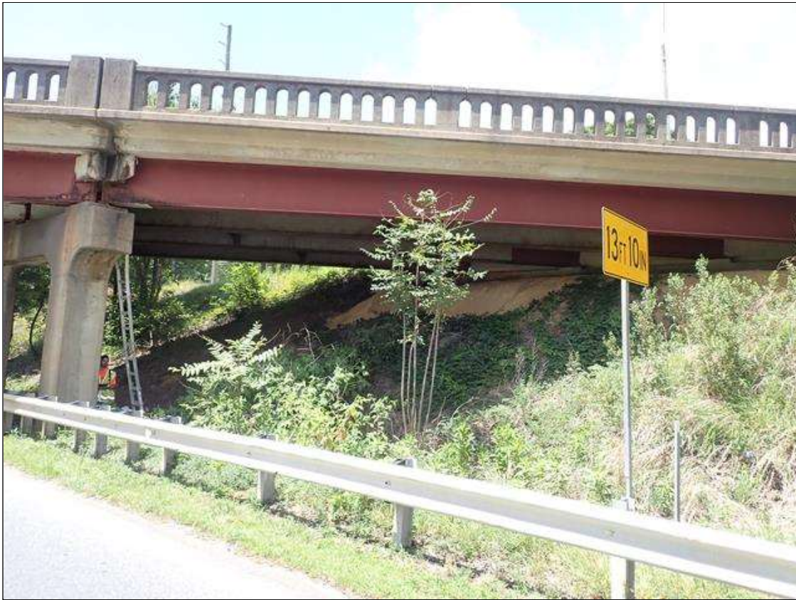
SPAN 3 EAST PROFILE, LOOKING NORTHWEST
