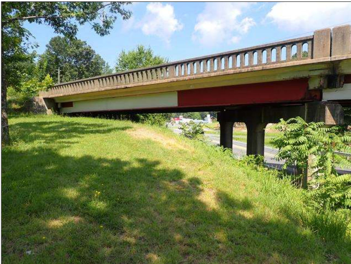
SPAN 1 EAST PROFILE, LOOKING WEST
