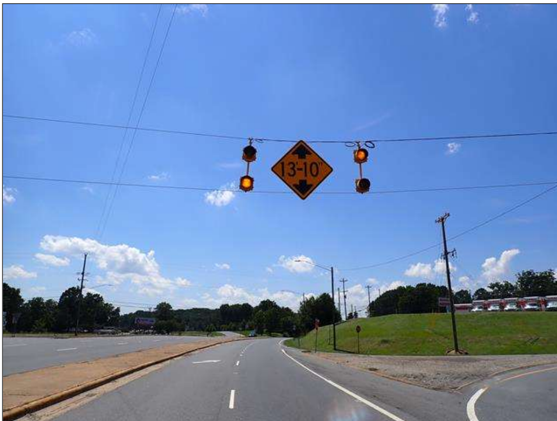
CLEARANCE SIGN OVER WESTBOUND LANES, APPROXIMATELY 1000 FOOT EAST OF BRIDGE
