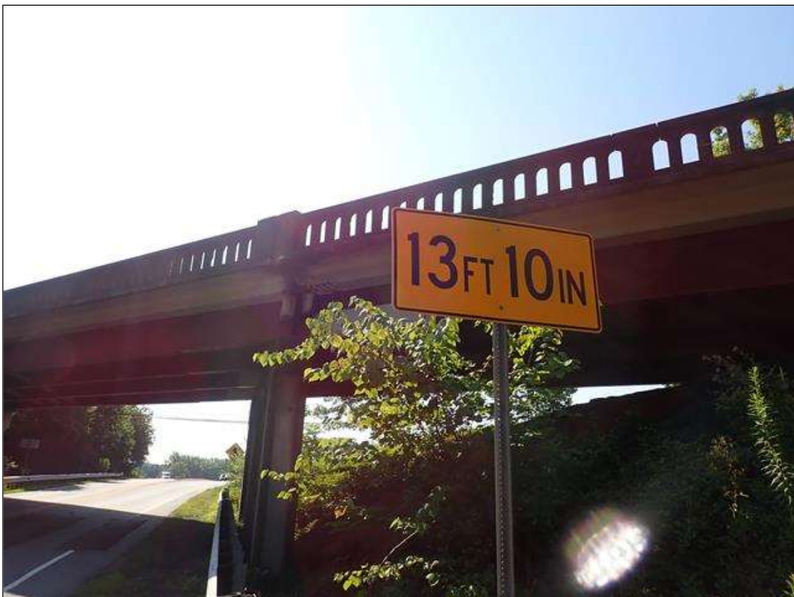
CLEARANCE SIGN, APPROXIMATELY 25 FEET WEST OF BENT 1
