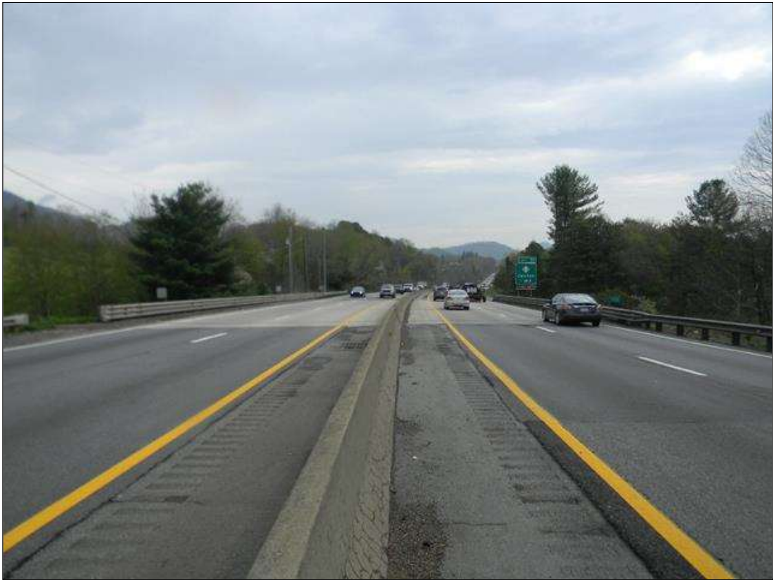
WEST APPROACH LOOKING EAST
