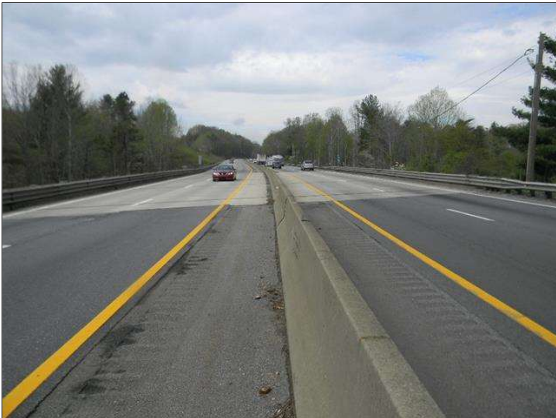
EAST APPROACH LOOKING WEST
