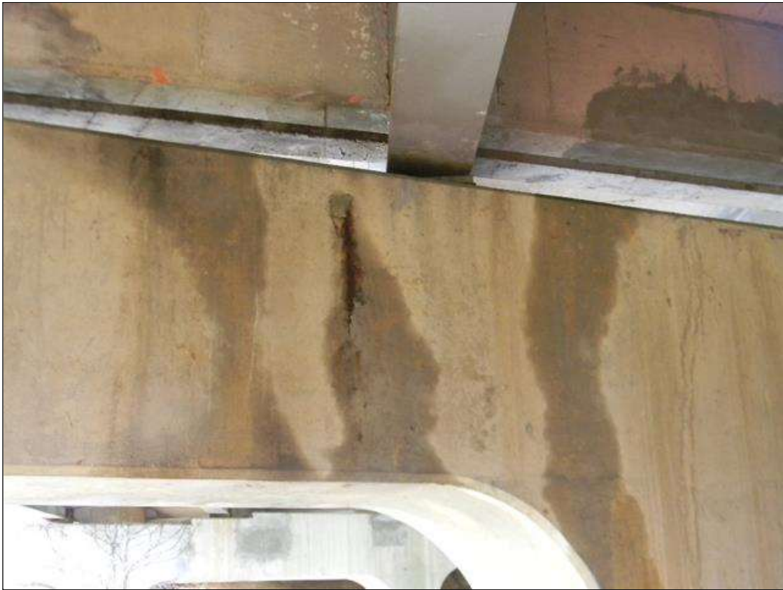
Bent 2 Cap 1: EAST FACE OF THE CAP HAS A 12" LONG EXPOSED REBAR UNDER BEAM 8.
