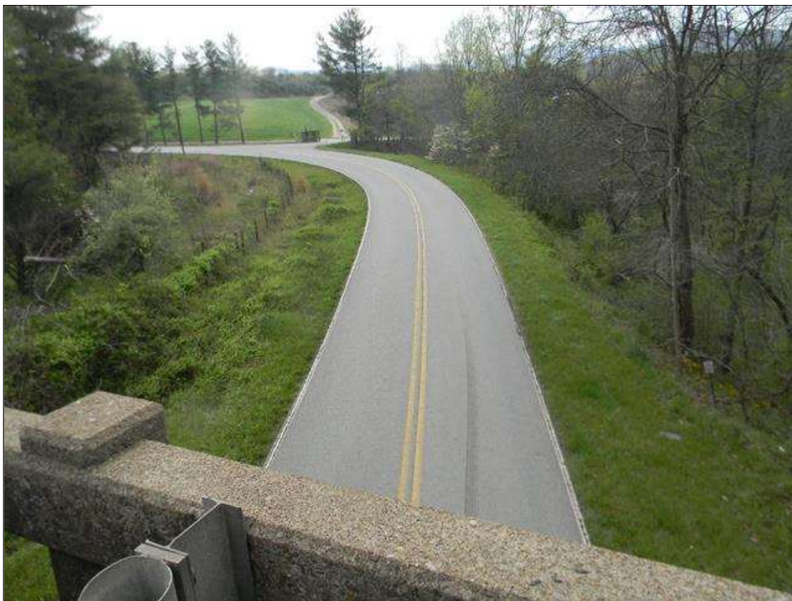
LOOKING SOUTH FROM THE STRUCTURE
