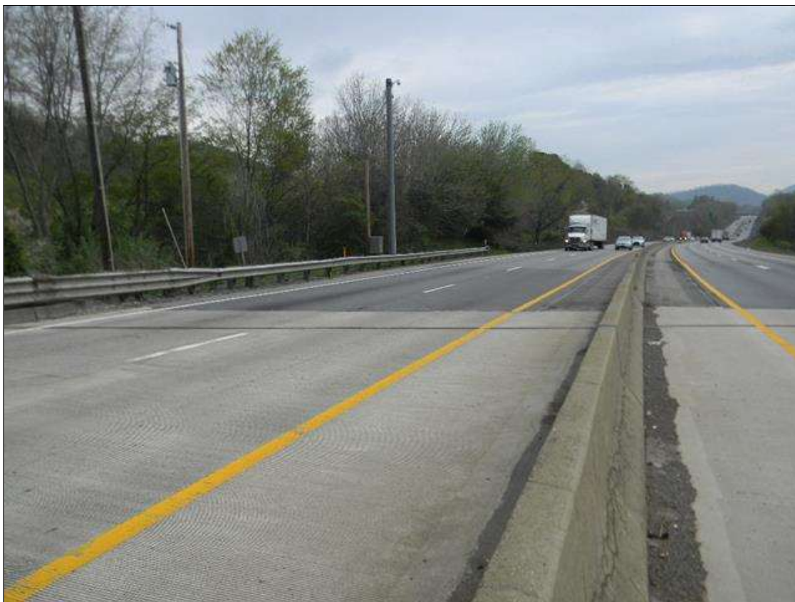
GUARDRAIL LOOKING EAST
