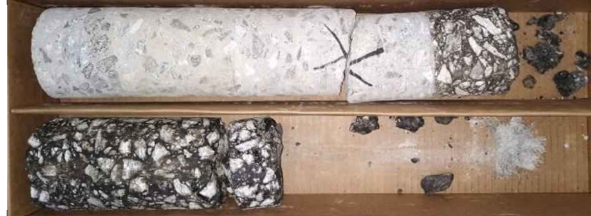
C-33 Y Sta. 30+94 EB OSL (continued)
