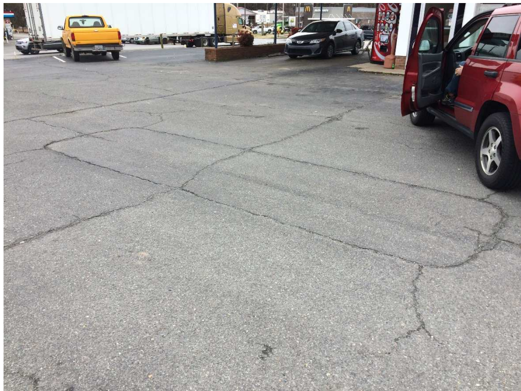
C. Photo of possible former pump island location, center of site.
