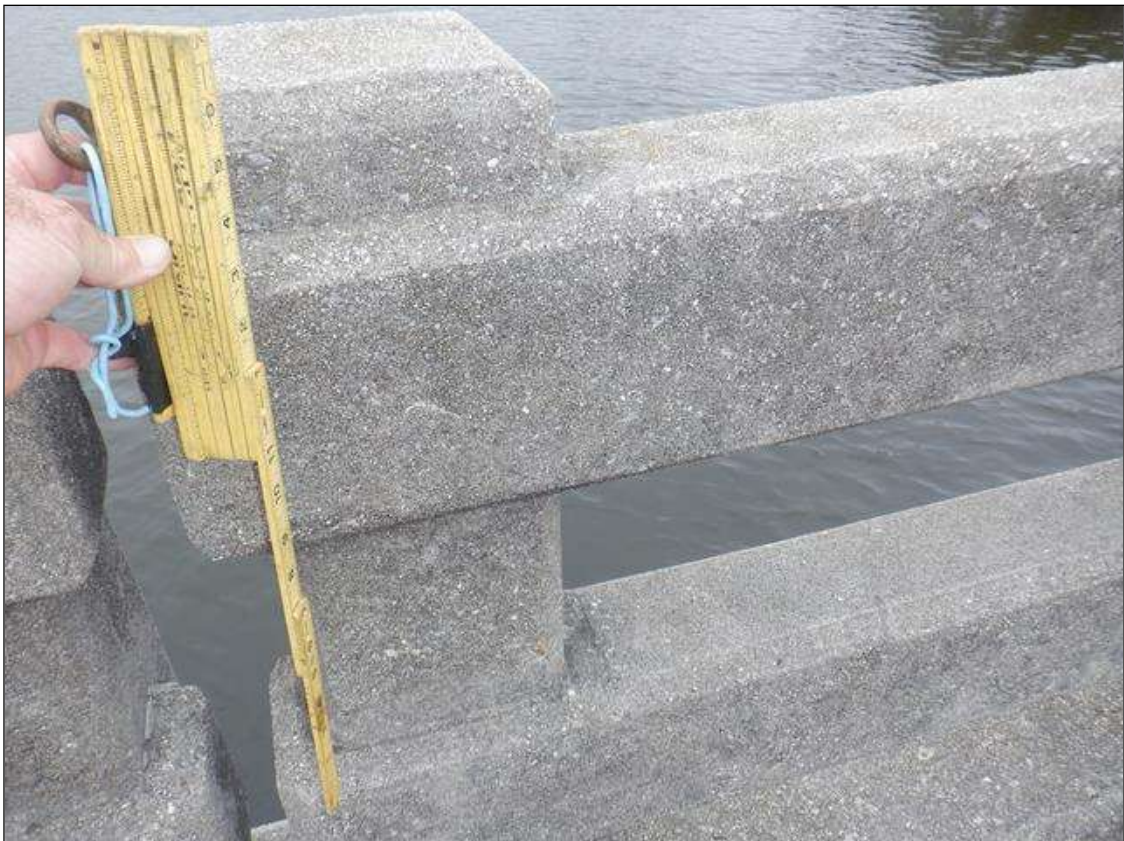
SCALING TO .125 INCH ON RAILS
