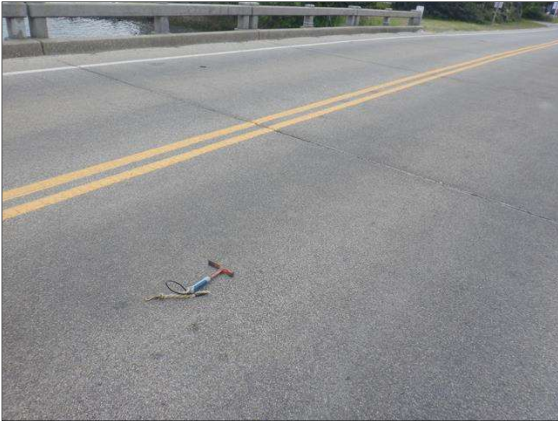
EPOXY WEARING SURFACE OVERVIEW
