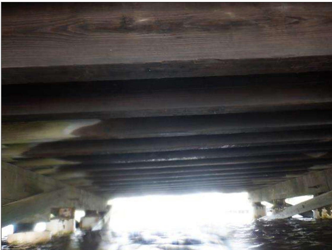
BOTTOM OF DECK SPAN 3
