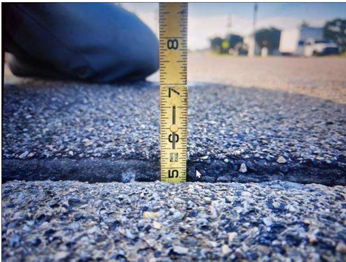
EPOXY WEARING SURFACE IS .375 INCH THICK
