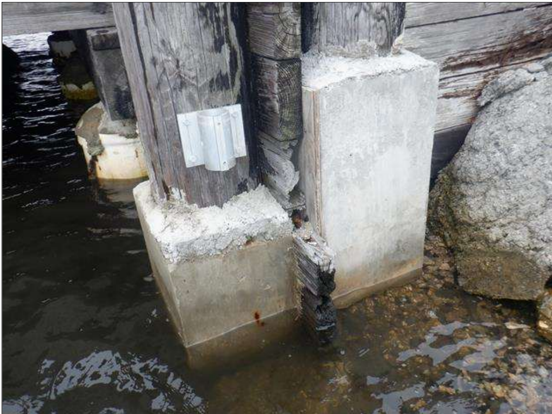
PREVIOUS PAR ADDRESSED. ALL RETAINING PILES HAVE BEEN ENCASED IN CONCRETE.
