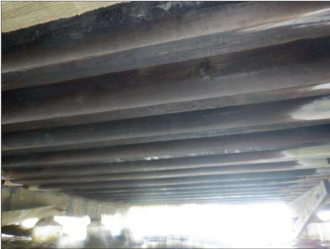
BOTTOM OF DECK SPAN 2
