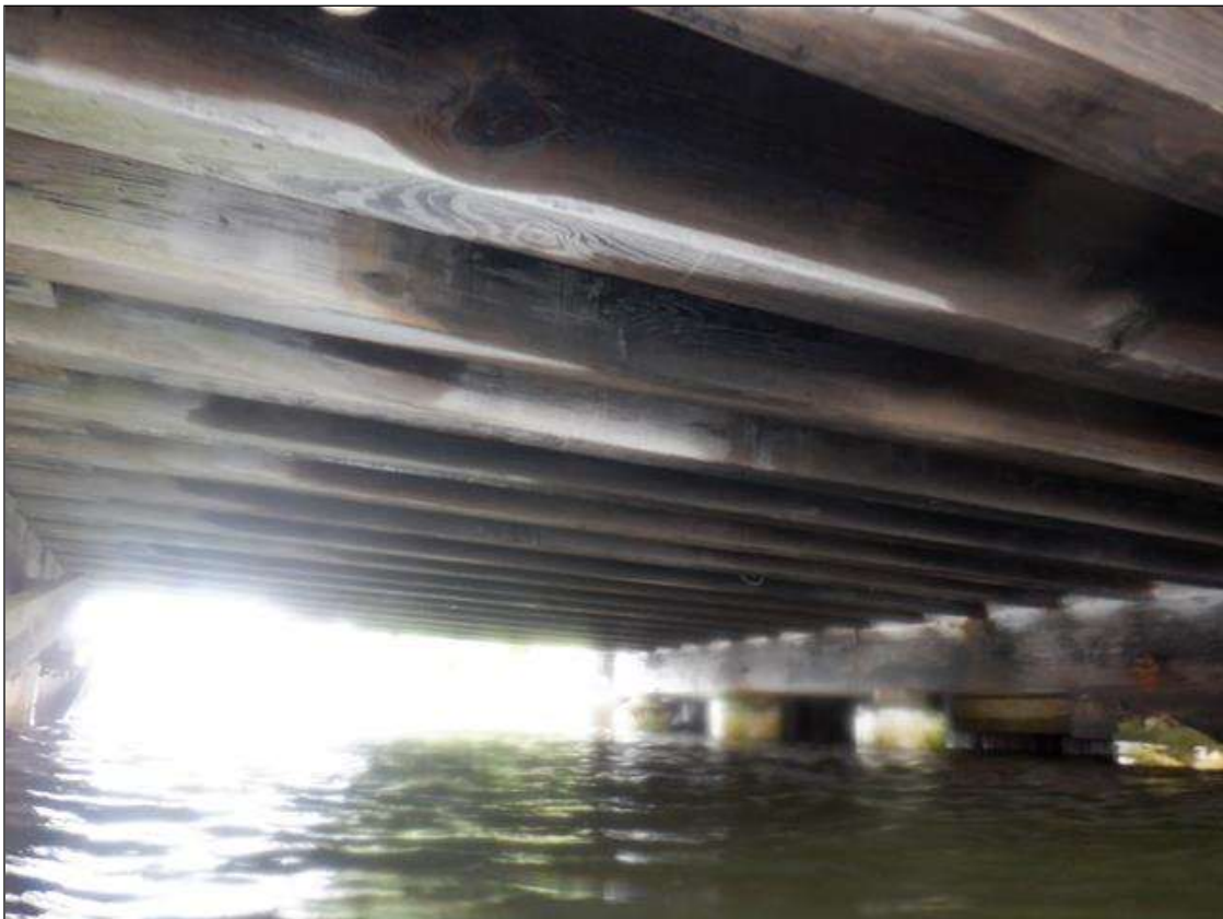
BOTTOM OF DECK SPAN 5
