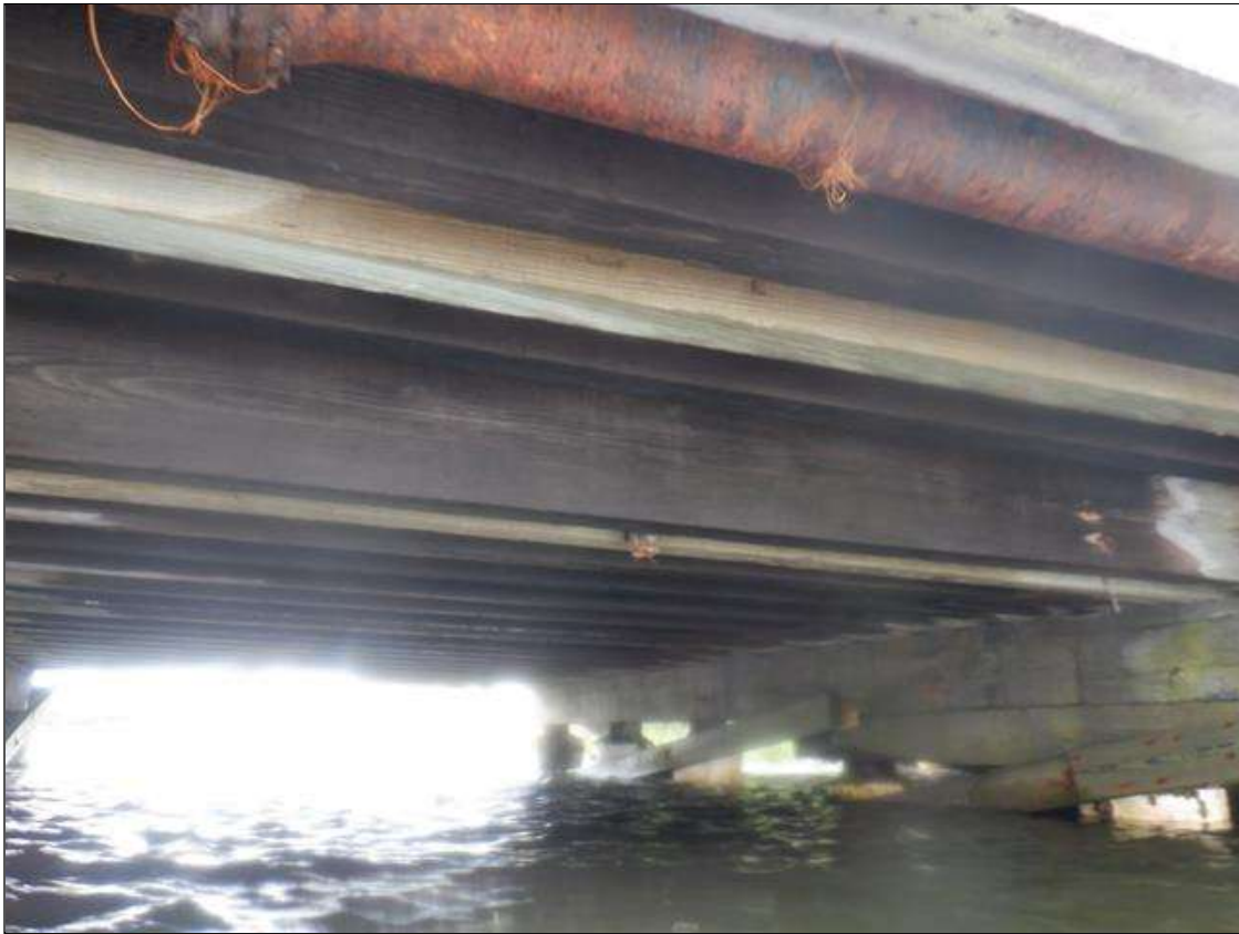
BOTTOM OF DECK SPAN 4
