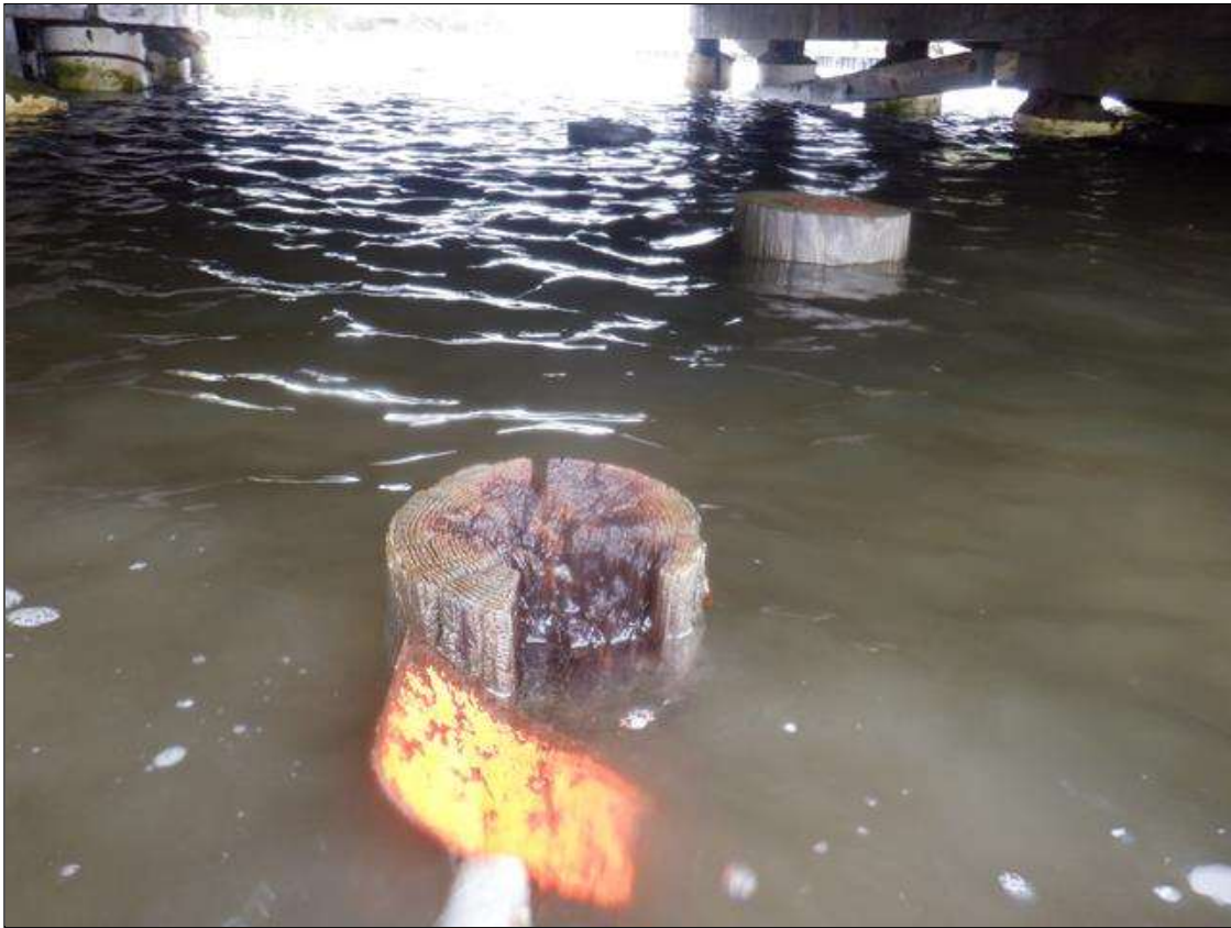
OLD SUBSTRUCTURE IN WATERWAY
