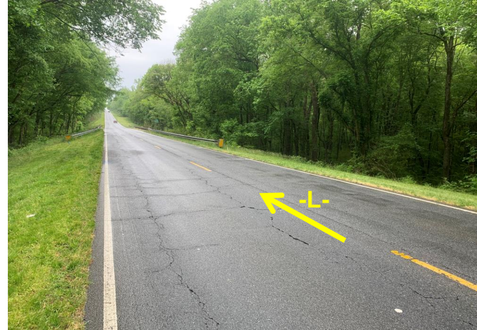
View of US 52 looking northwest.
