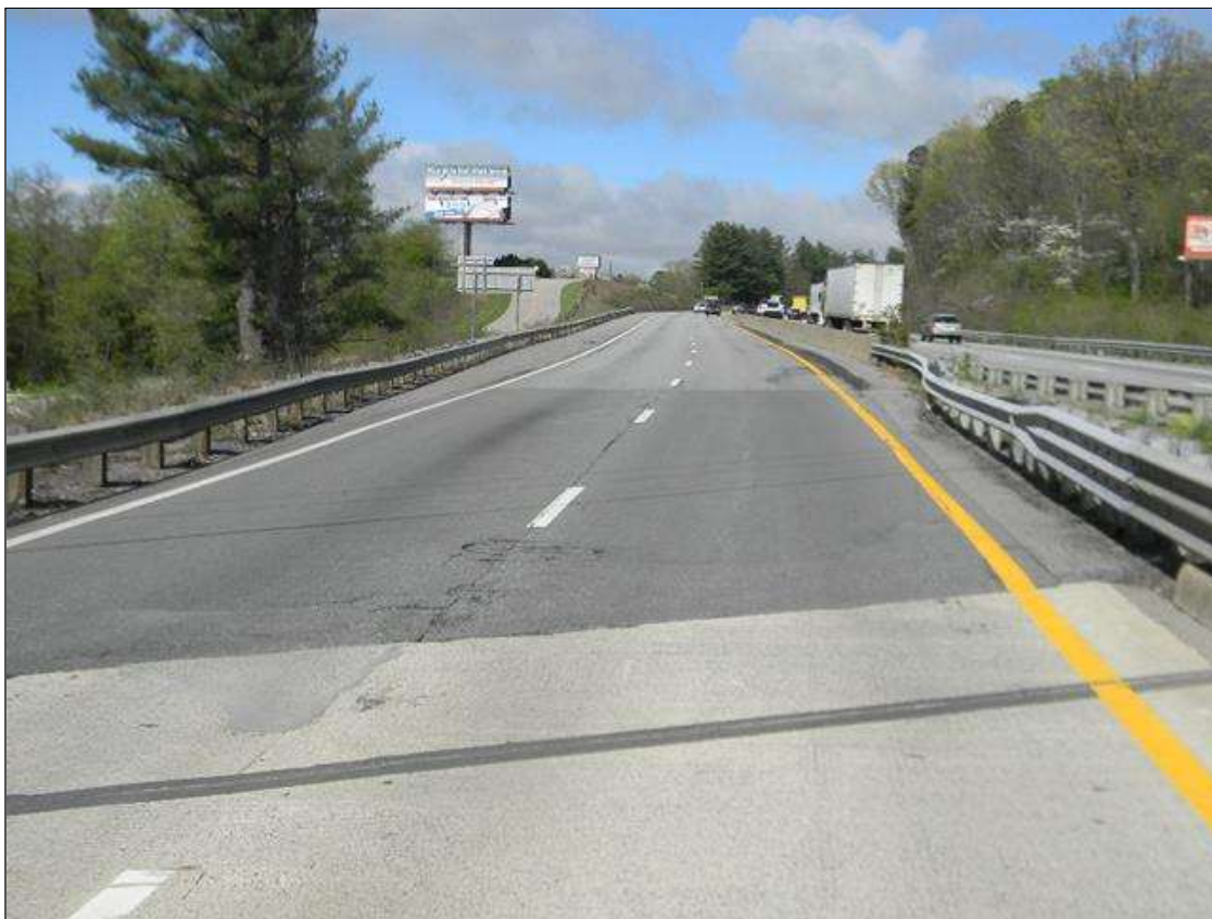
GUARDRAIL LOOKING WEST
