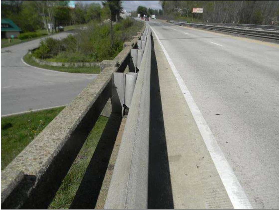
TRI-BEAM RAIL WAS INSTALLED INSIDE OF THE ORIGINAL CONCRETE RAIL.
