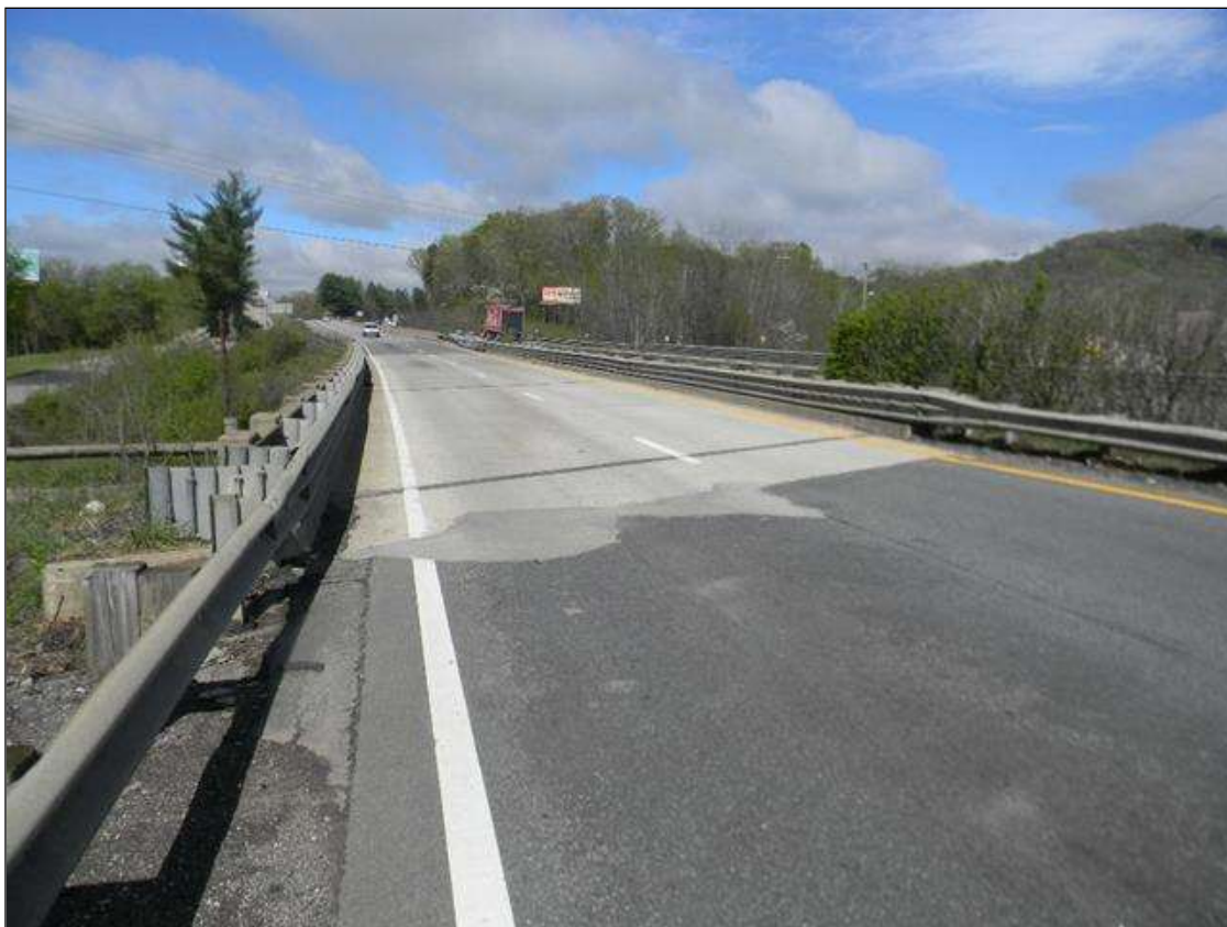
EAST APPROACH LOOKING WEST
