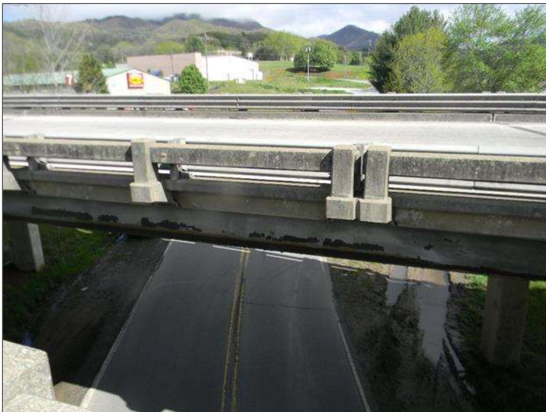
LOOKING NORTH FROM THE STRUCTURE
