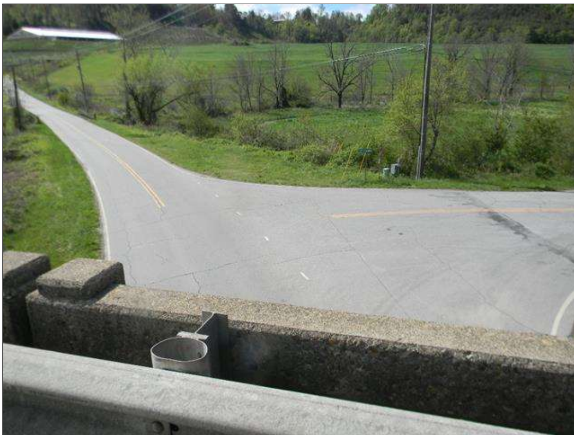
LOOKING SOUTH FROM THE STRUCTURE
