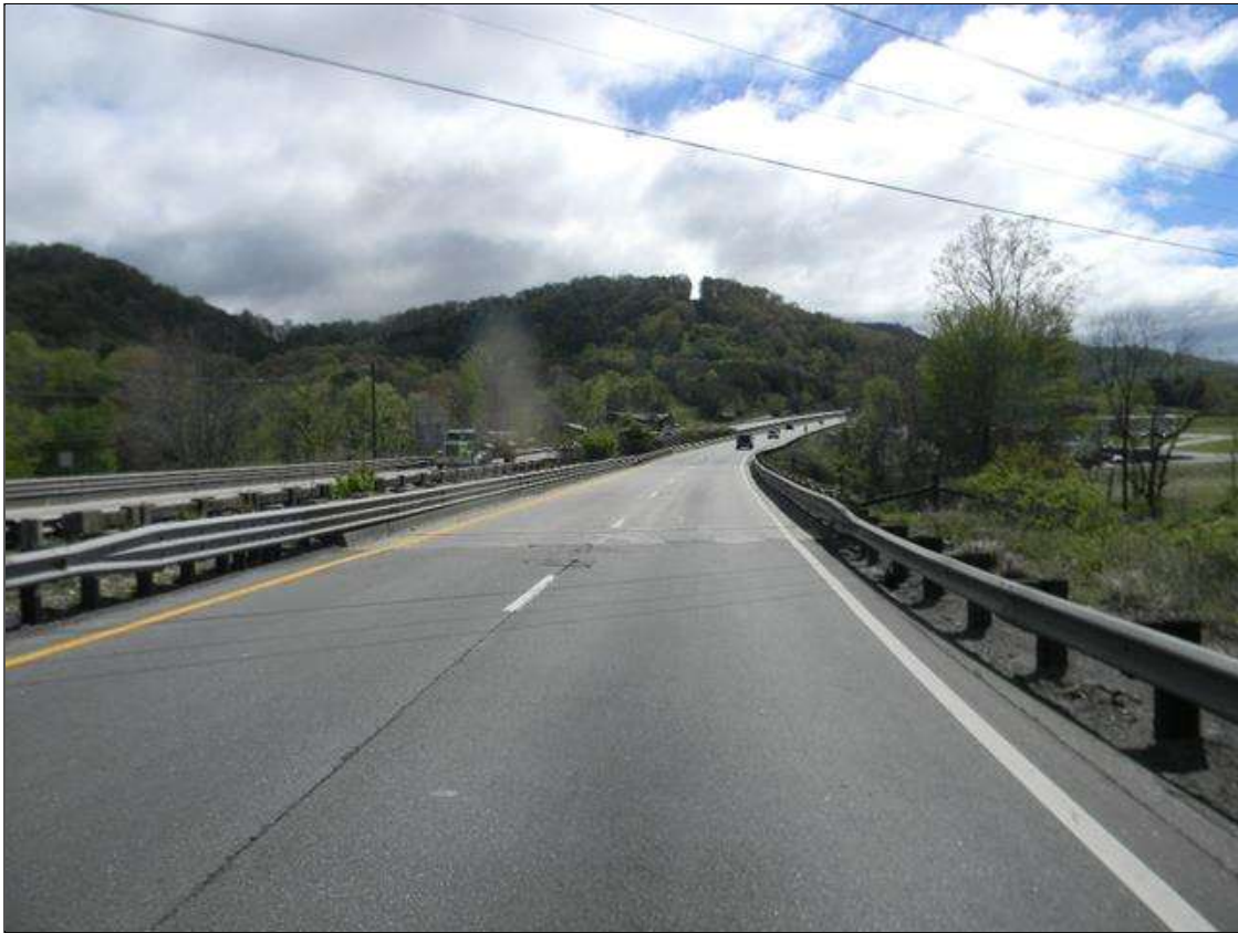
WEST APPROACH LOOKING EAST
