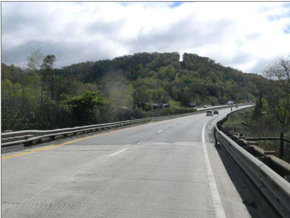
GUARDRAIL LOOKING EAST
