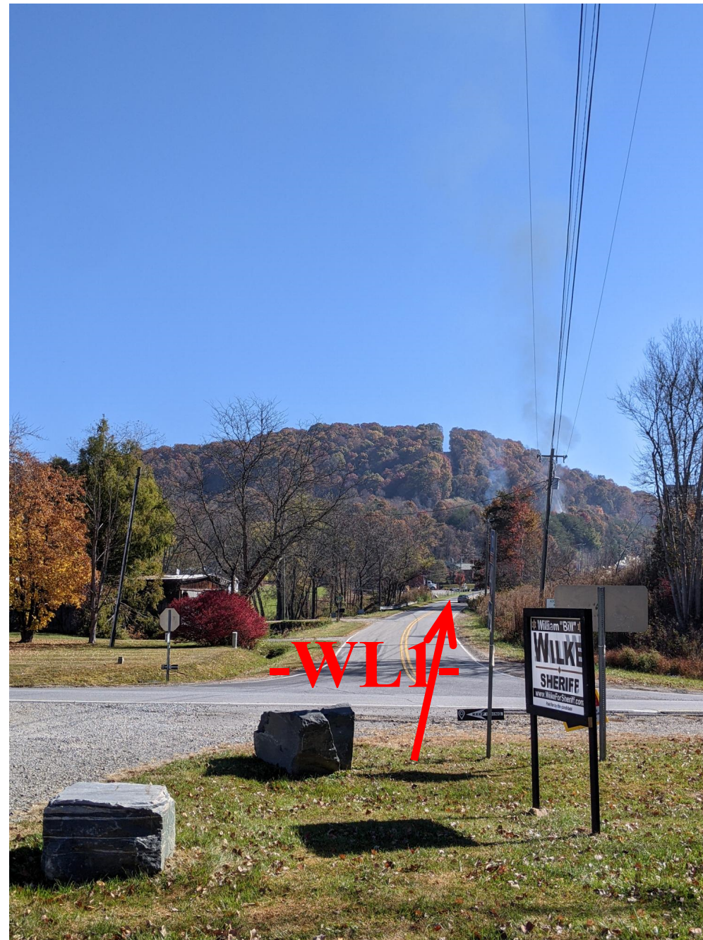
Looking East from West End of Retaining Wall along -WL1-
