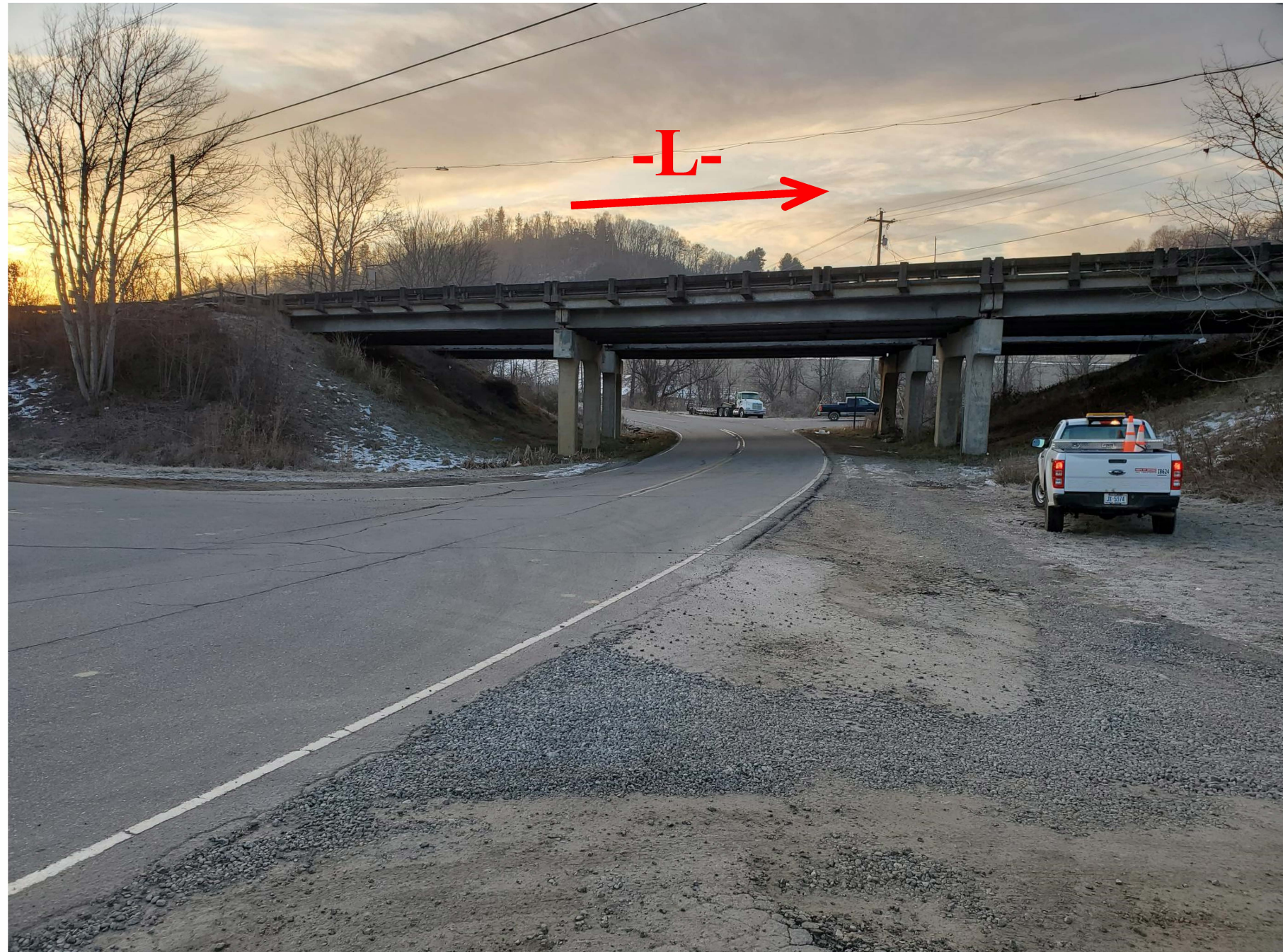
Looking South Along SR 1613
