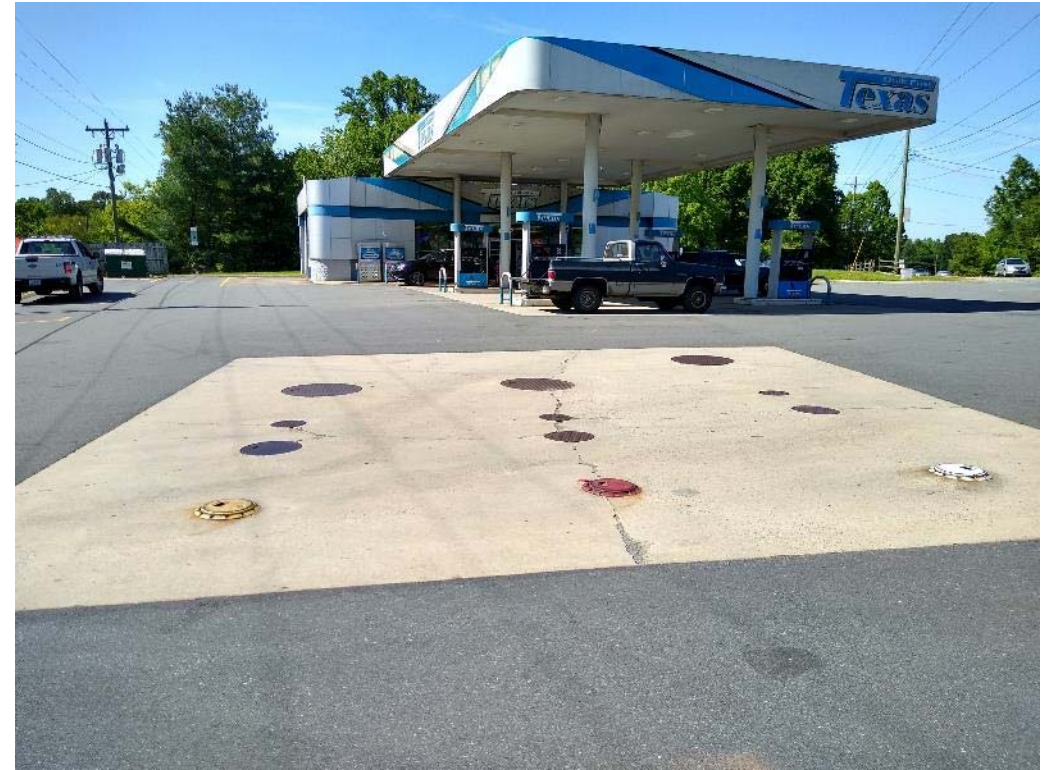
D. Photograph of tank bed, looking south.
