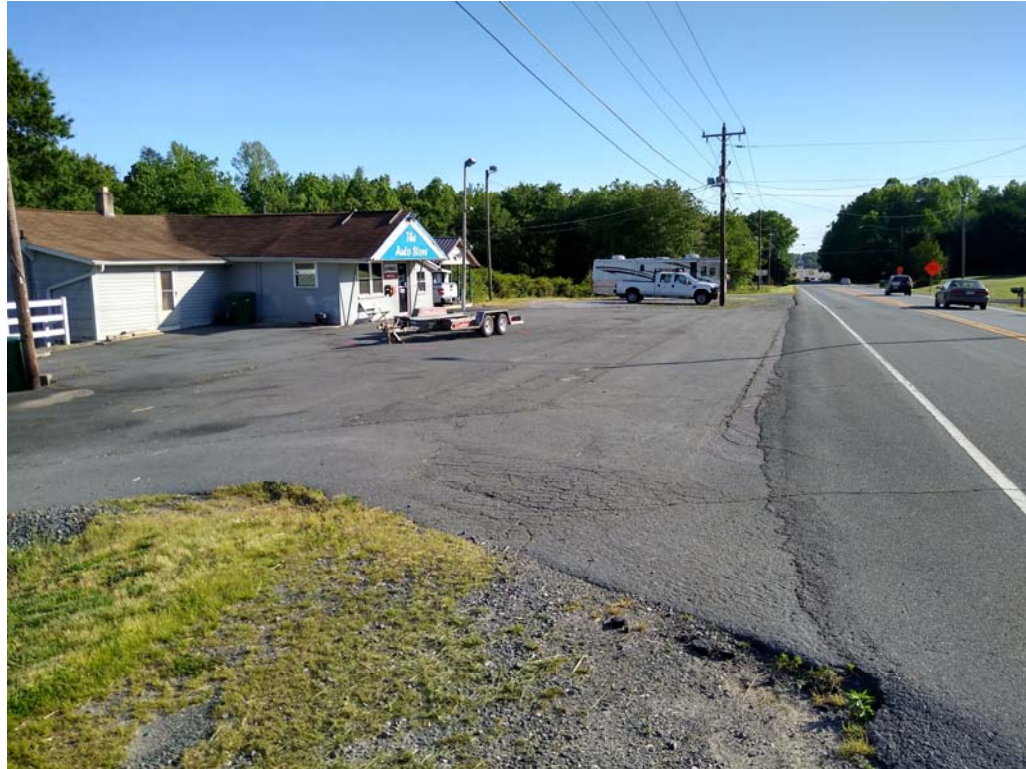
A. Photograph from northeast end, looking southwest.
