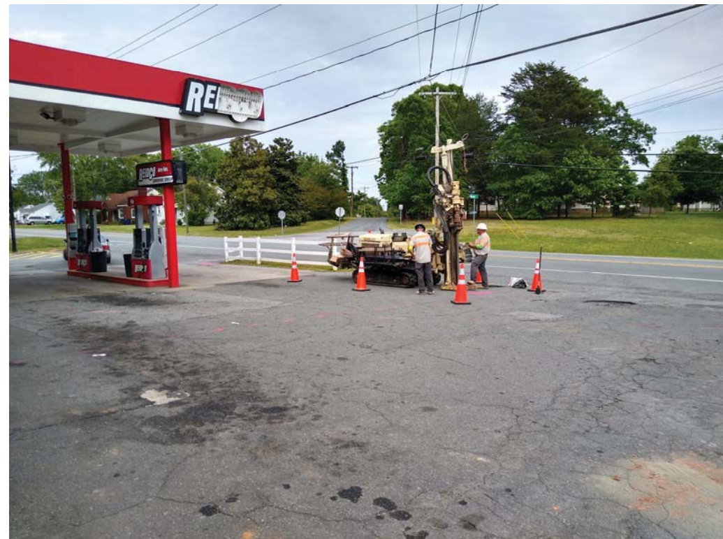
D. Photograph of drilling operations, looking northeast.
