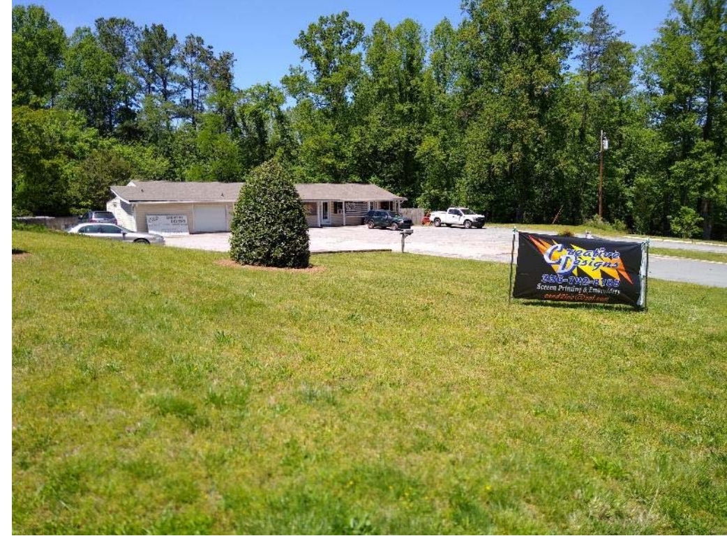
B. Photograph from south end, looking north.
