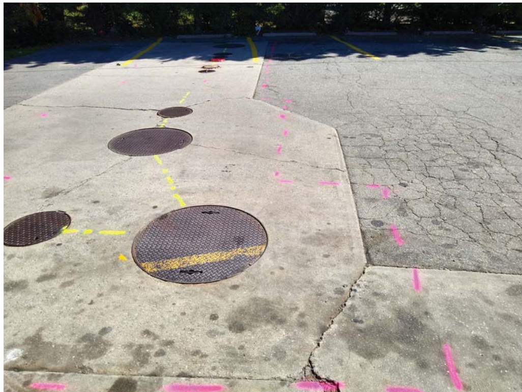
C. Photograph of tank bed area, looking northeast. Magenta lines are approximate edges of USTs, as indicated by GPR images.
