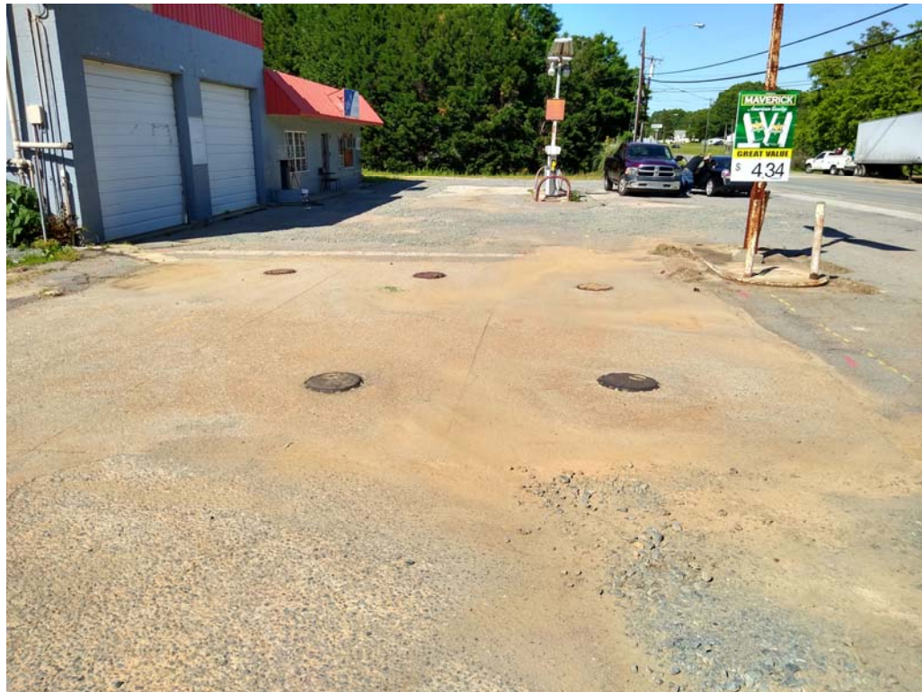
C. Photograph of tank bed area, looking northeast.
