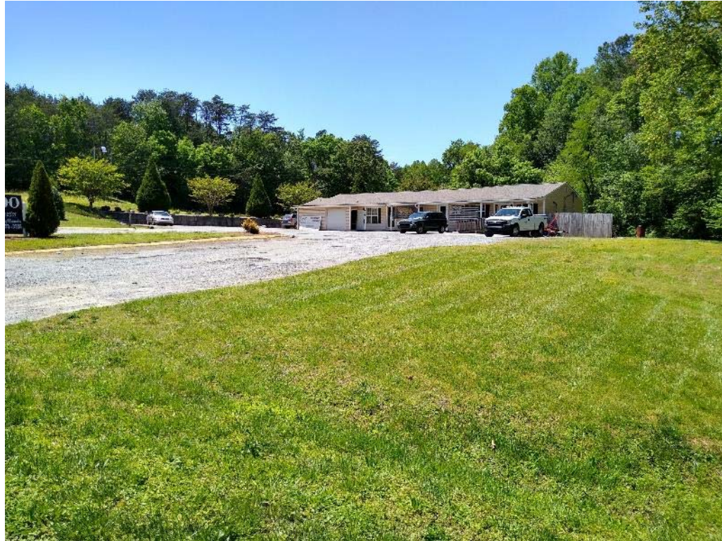
A. Photograph from northeast corner, looking southwest.
