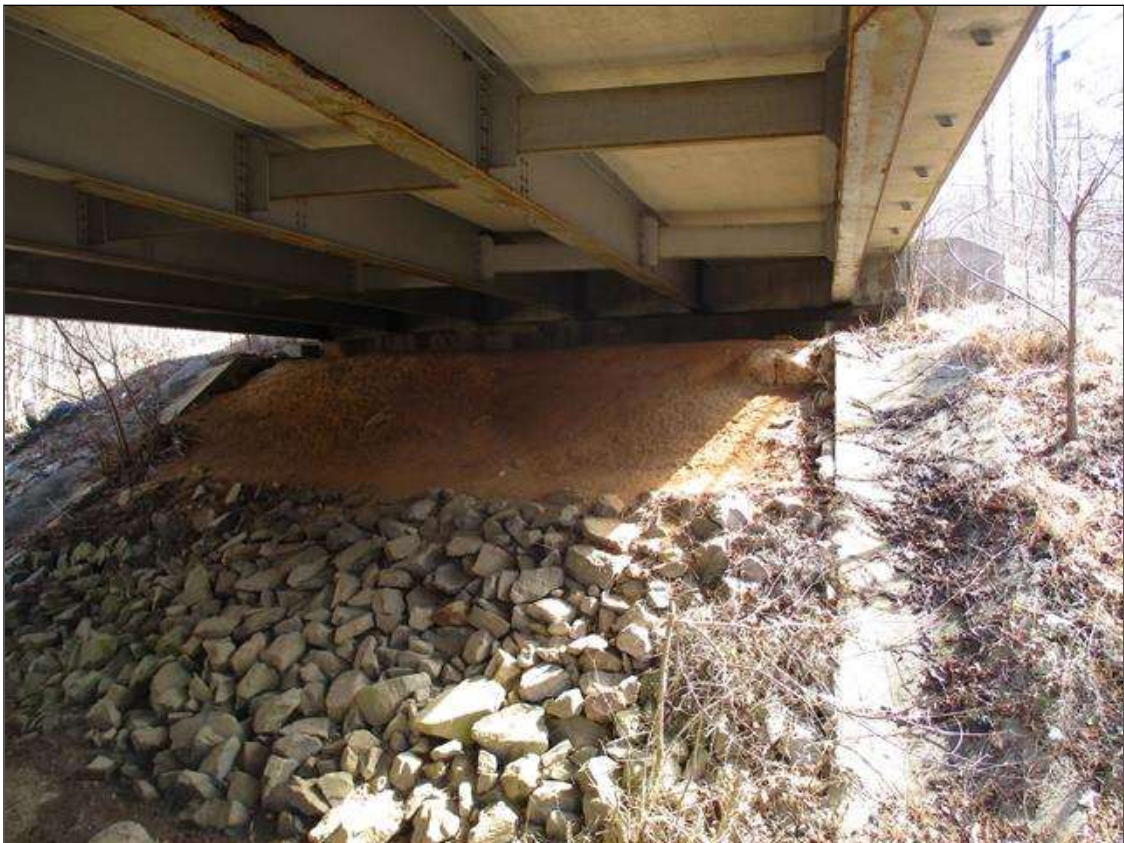
SLOPE @ END BENT 2
