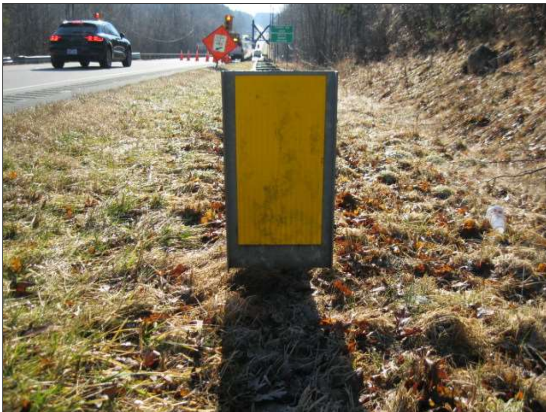
TYPICAL GUARDRAIL TERMINAL END
