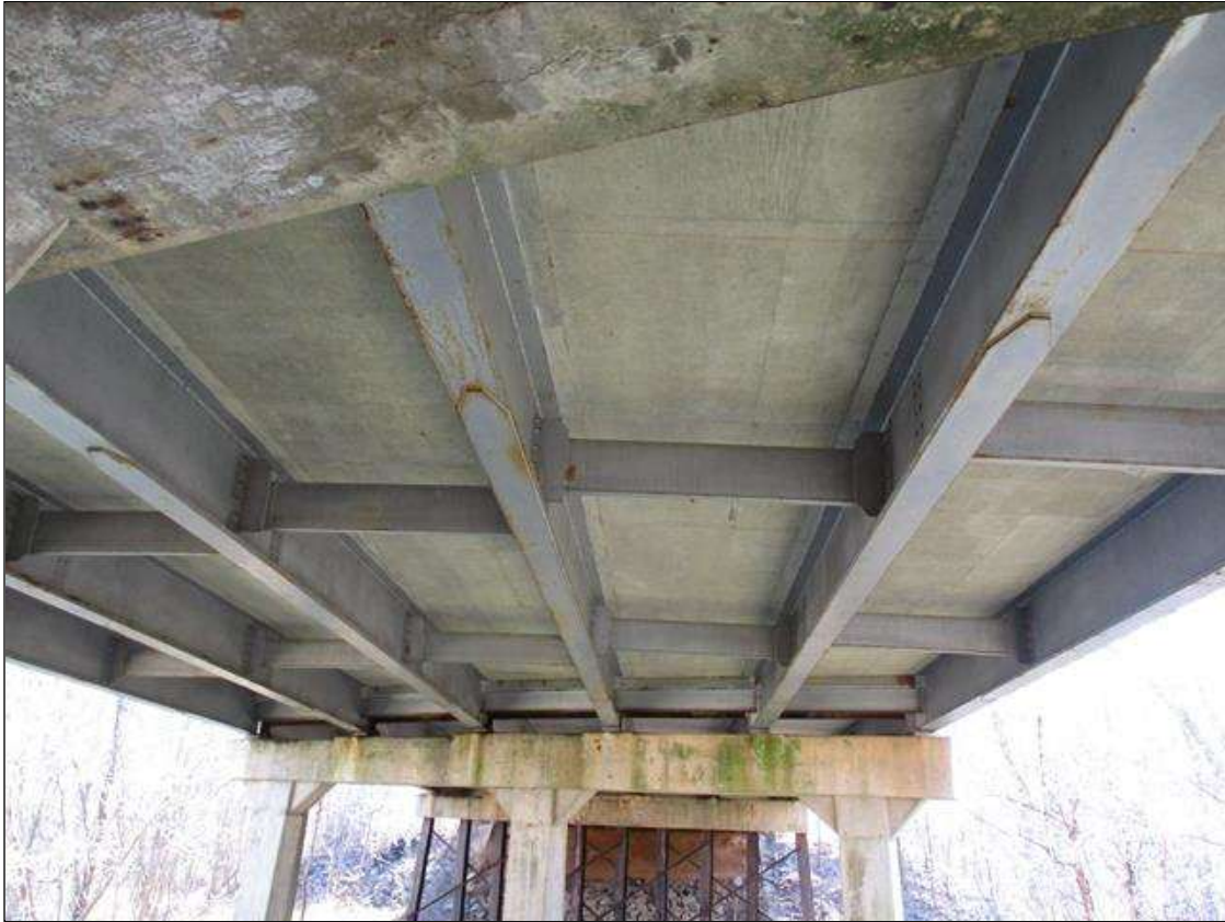
TYPICAL UNDERSIDE (SPAN 2 SHOWN)
