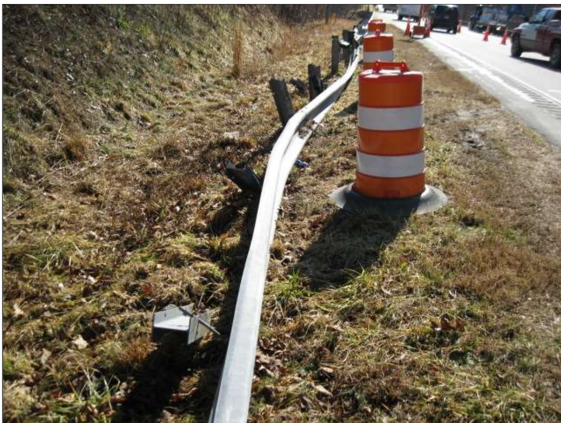
(PAR) GUARDRAIL DAMAGE AT NEAR LEFT APPROACH ADJACENT TO END TERMINATION, 50' SECTION IMPACTED
