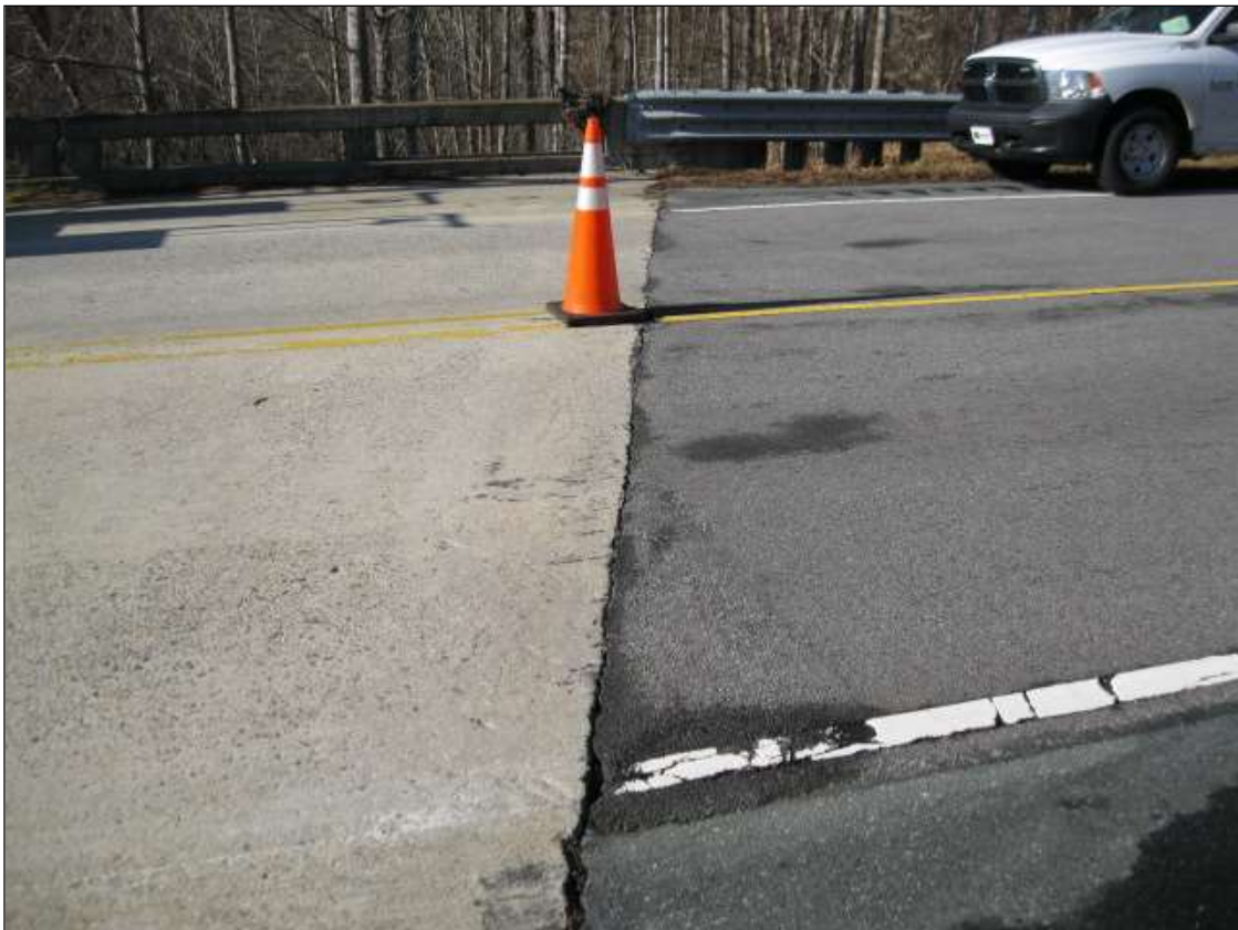
TYPICAL END BENT EXPANSION JOINT
