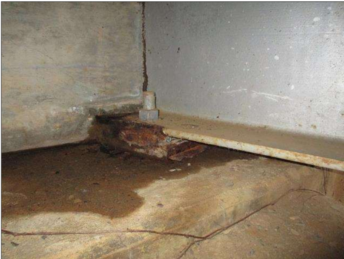
TYPICAL END BENT BEARING (END BENT 1 SHOWN)
