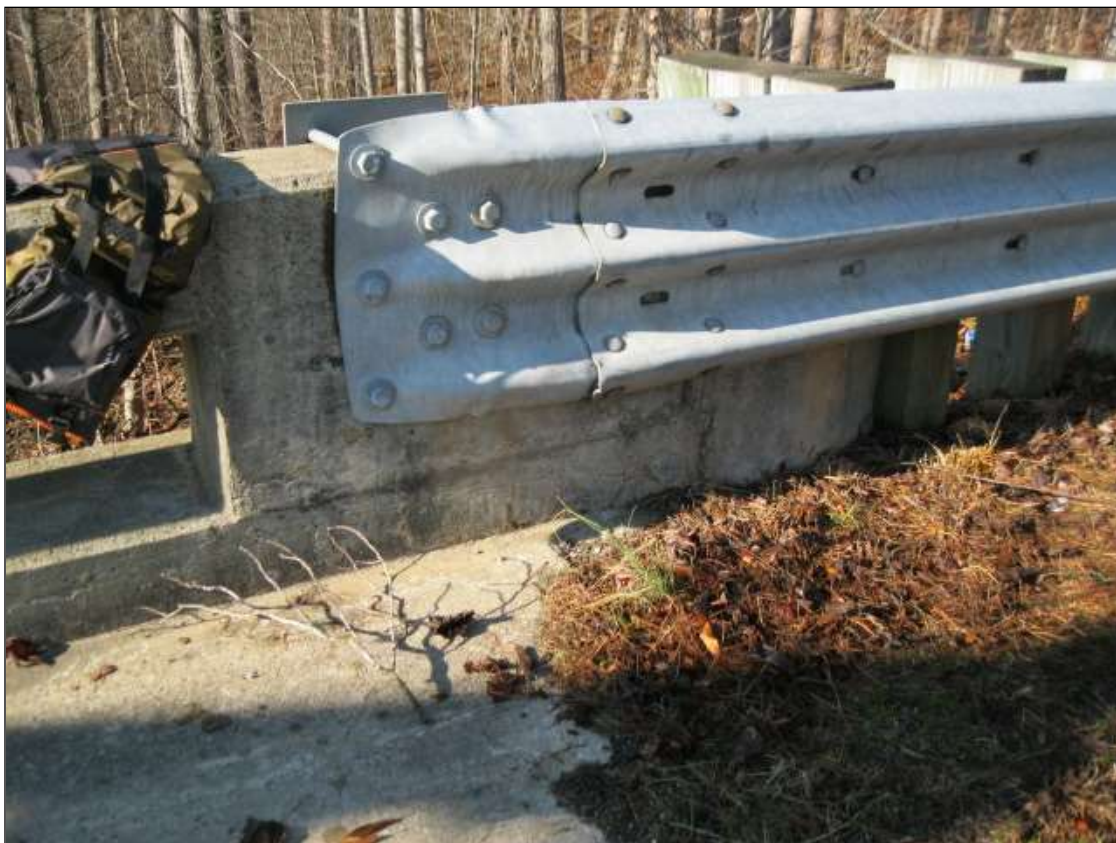
BRIDGE RAIL TO GUARDRAIL CONNECTION
