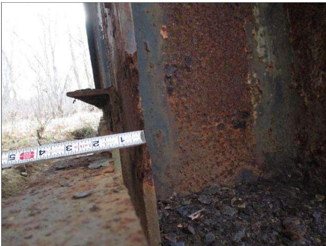
Bent 3 Pile 4: (PAR) FAR FLANGE DOWN TO KNIFE EDGE
