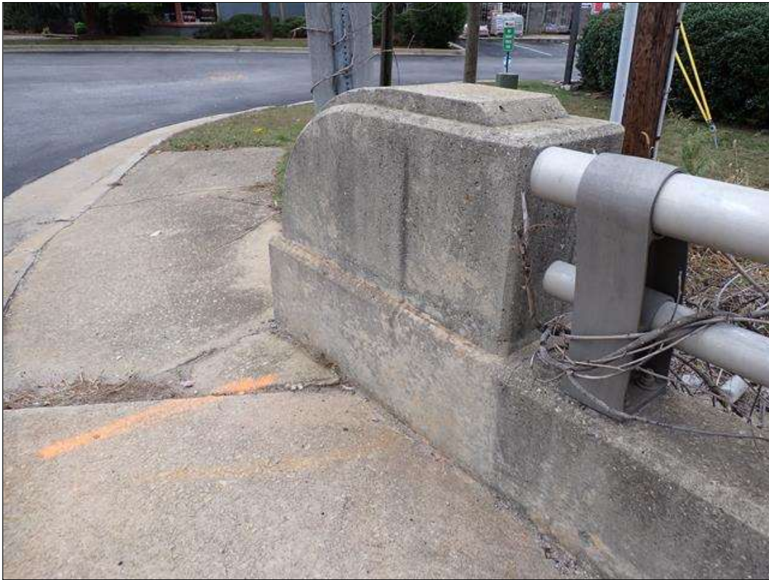
RIGHT RAIL END POST AT NORTHEAST CORNER
