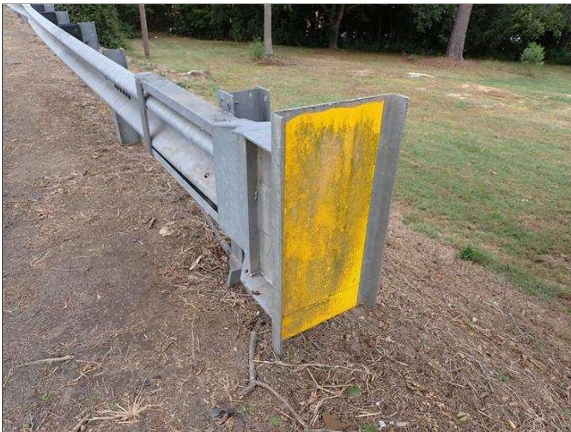
GUARDRAIL END TREATMENT AT NORTHWEST CORNER, SOUTHWEST SIMILAR
