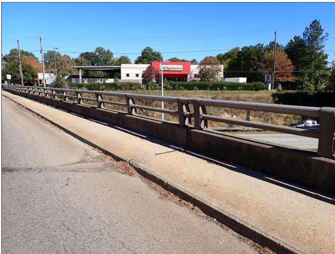
RIGHT RAIL, LEFT RAIL SIMILAR
