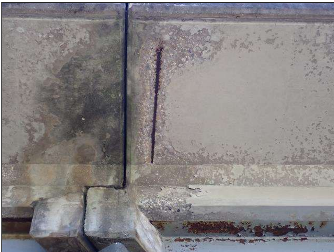
Span 2 Deck: 6 INCH X 36 INCH X 1 INCH DEEP SPALL WITH EXPOSED REINFORCING, EAST OVERHANG AT BENT 1.
