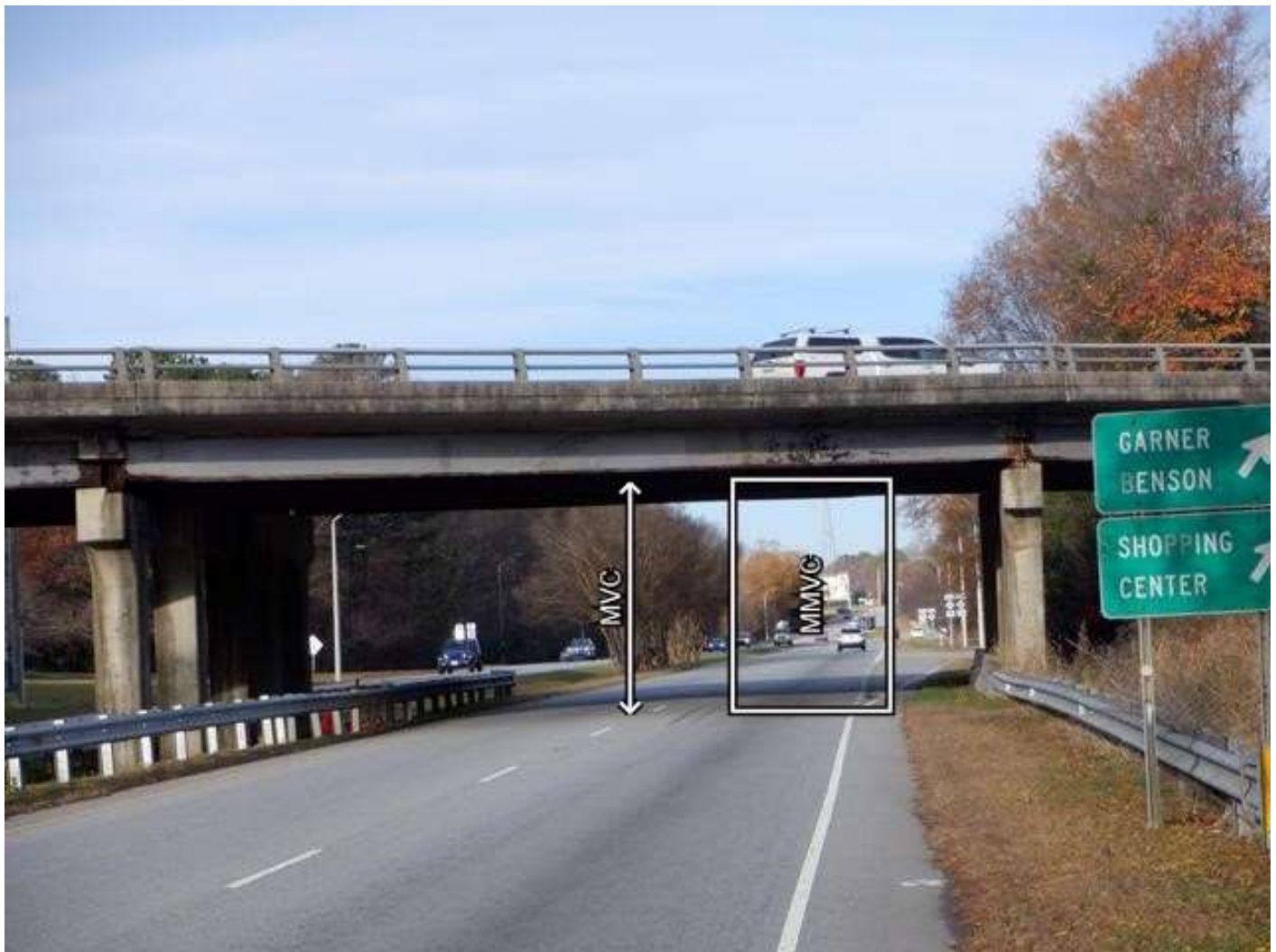
LOOKING WEST AT SPAN 3.
