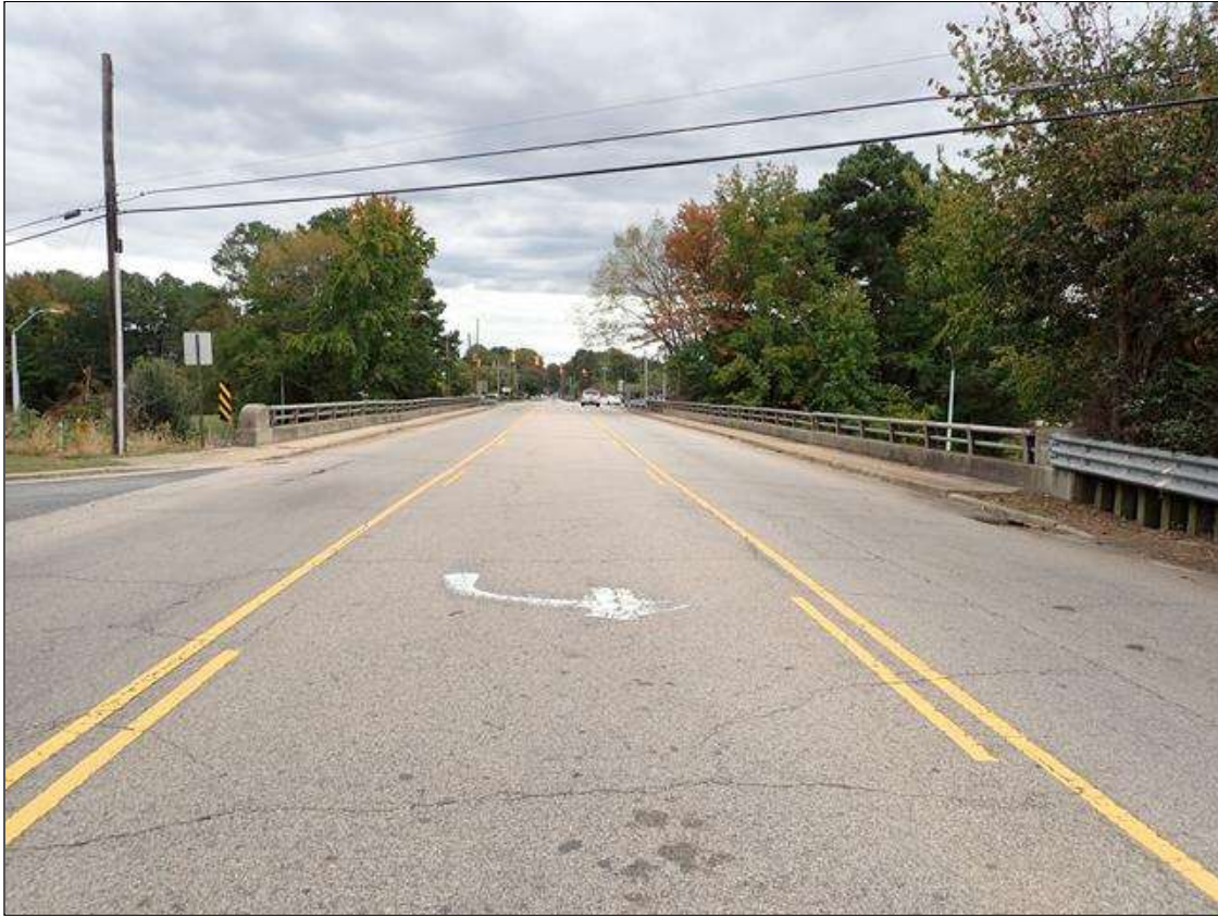
NORTH APPROACH, LOOKING SOUTH
