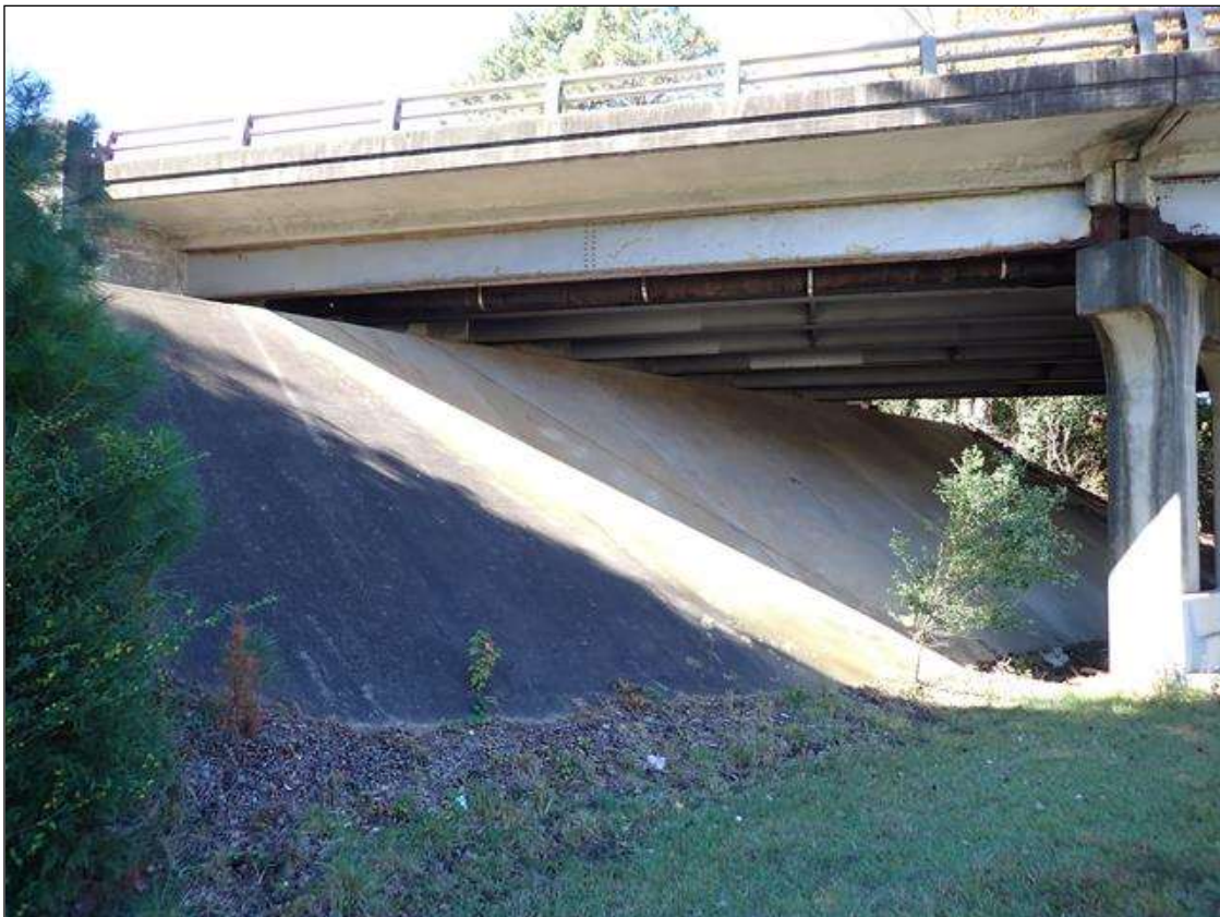
SPAN 1 EAST PROFILE, LOOKING SOUTHWEST
