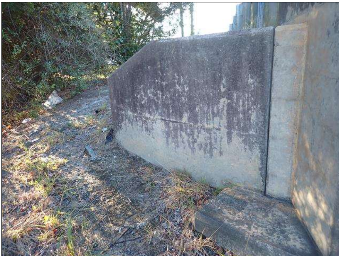
SOUTHEAST WINGWALL, OTHERS SIMILAR
