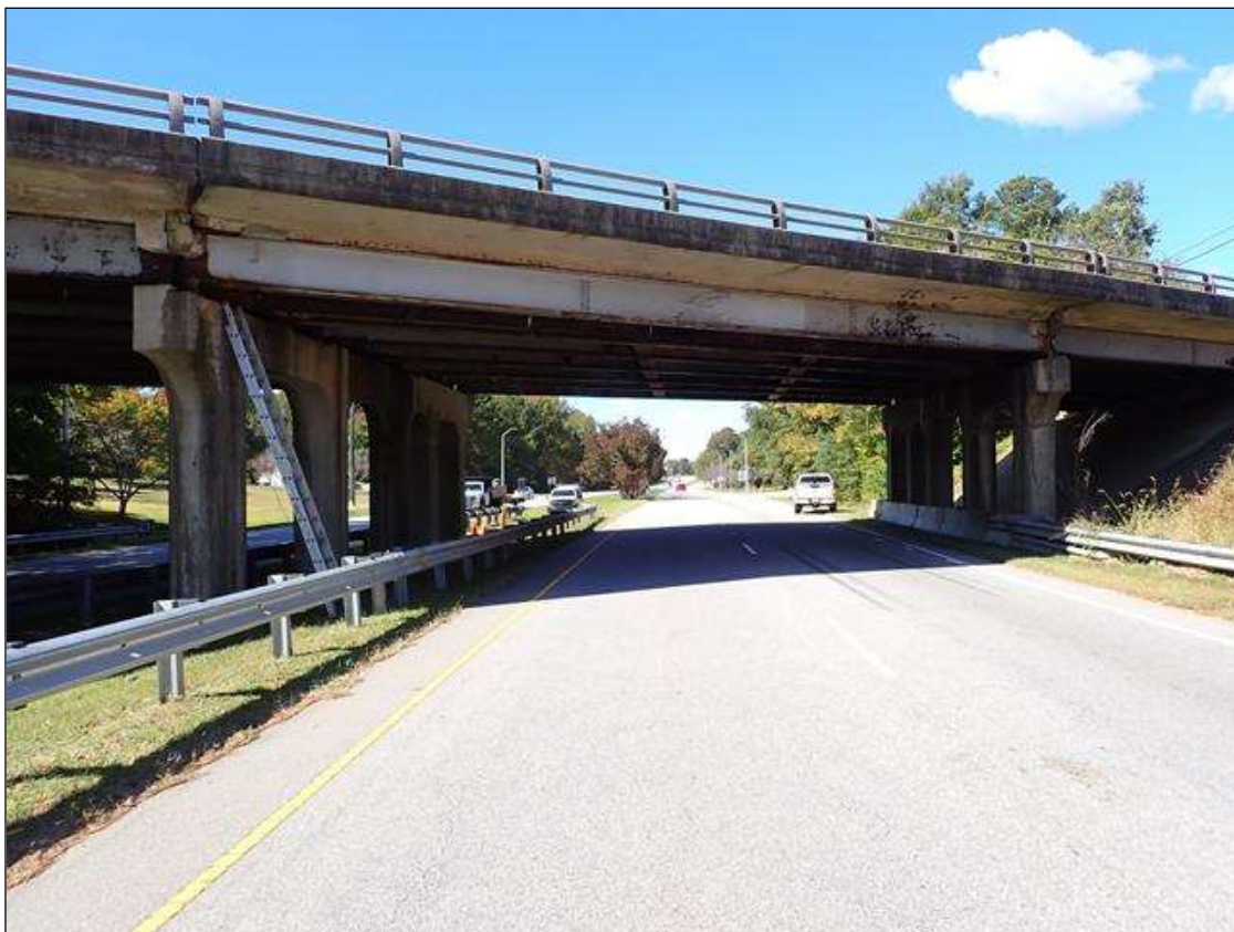
SPAN 3 EAST PROFILE, LOOKING WEST
