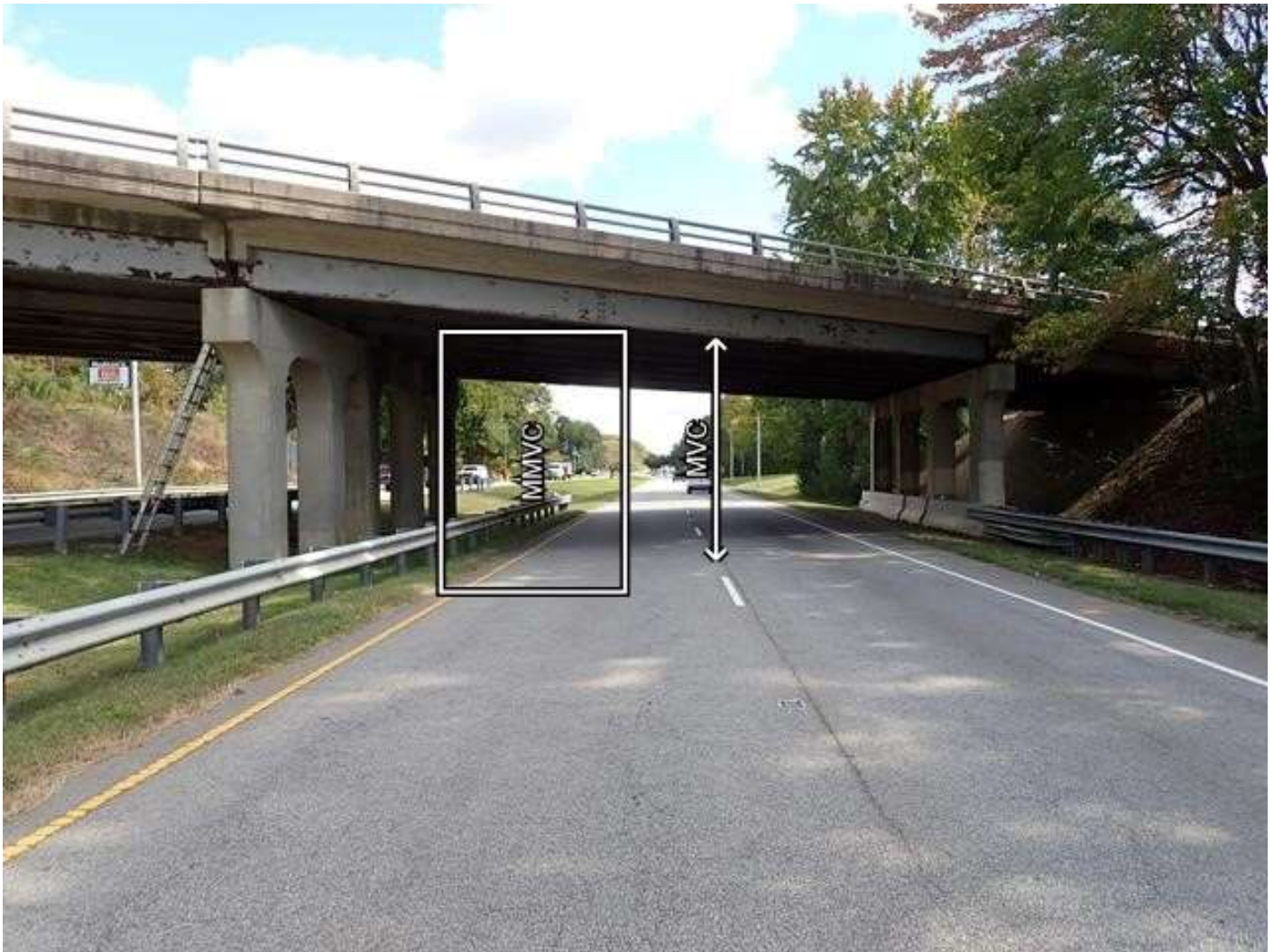
SPAN 2 WEST PROFILE, LOOKING EAST - LIDAR
