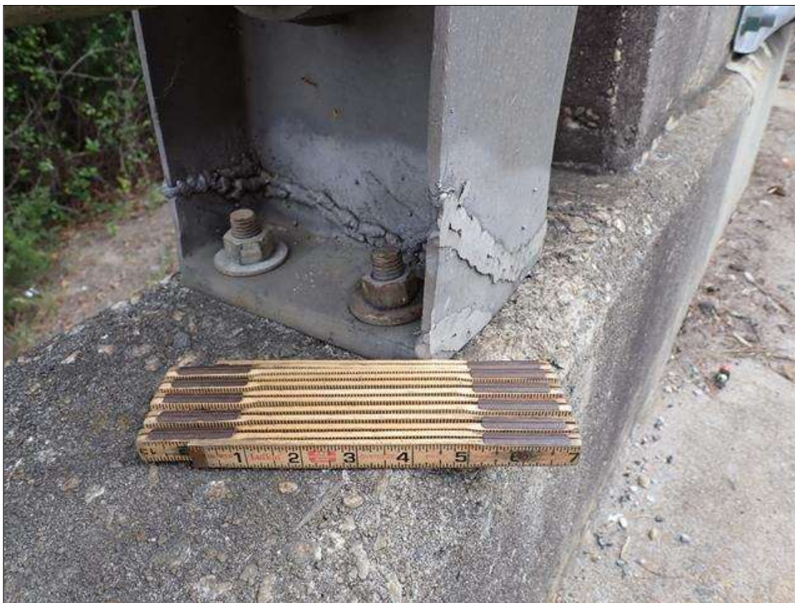
Span 1 Right Bridge Rail: WELDED REPAIR TO BOTTOM OF ALUMINUM POST 1
