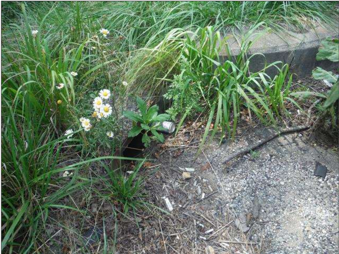
near left drainage structure
