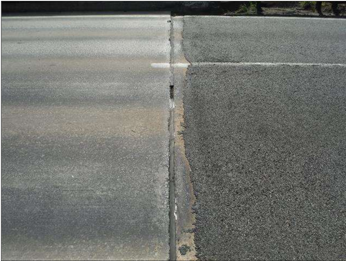
end bent 2 joint
