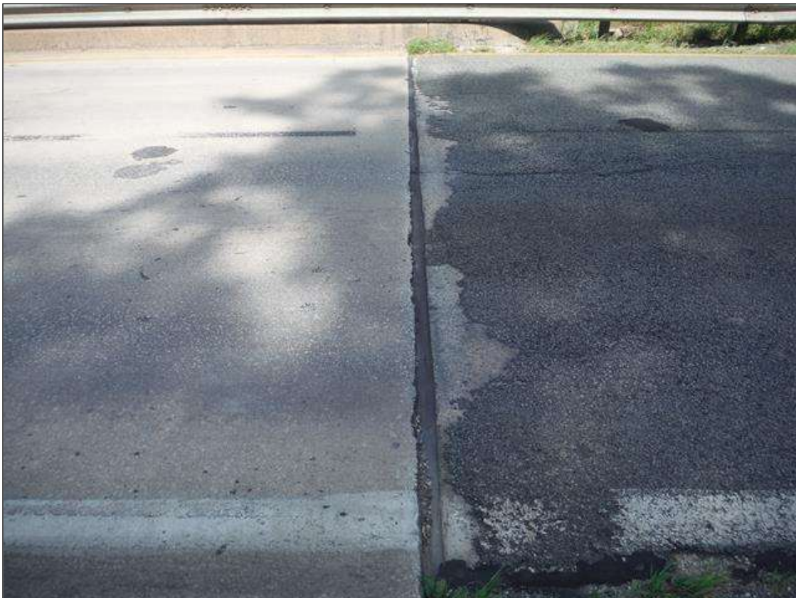
end bent 1 expansion joint
