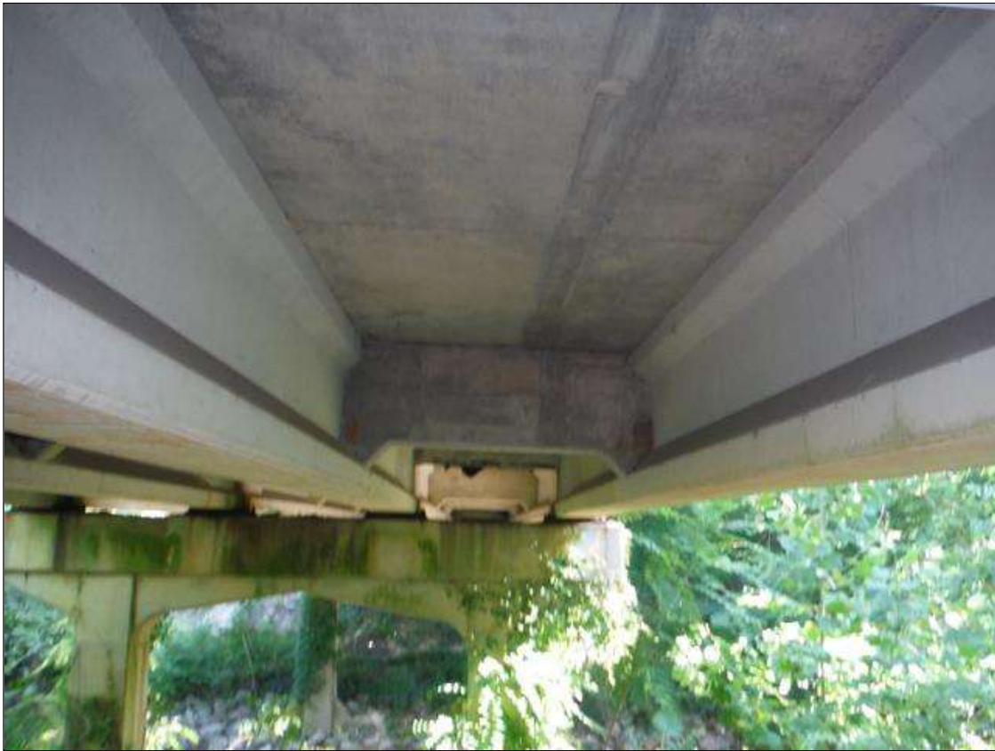
span 1 bay 3 intermediate diaphragm
