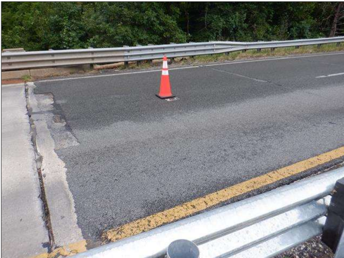
South approach asphalt
