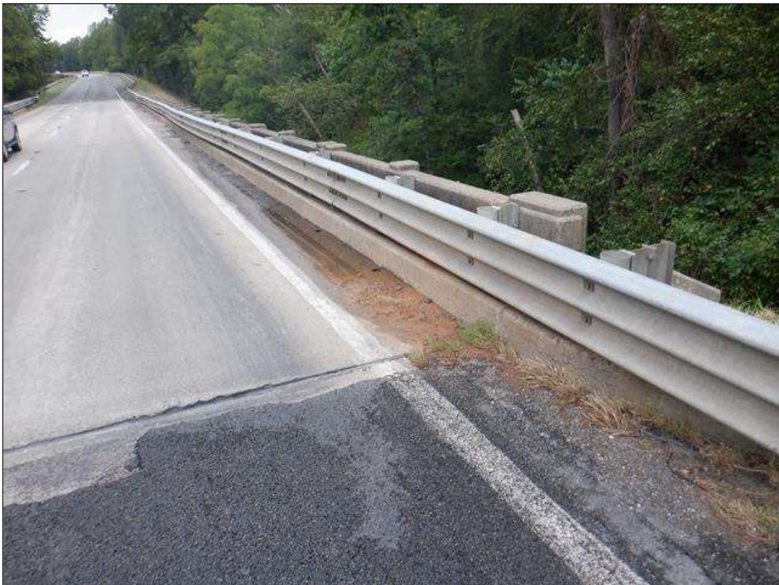
right bridge rail
