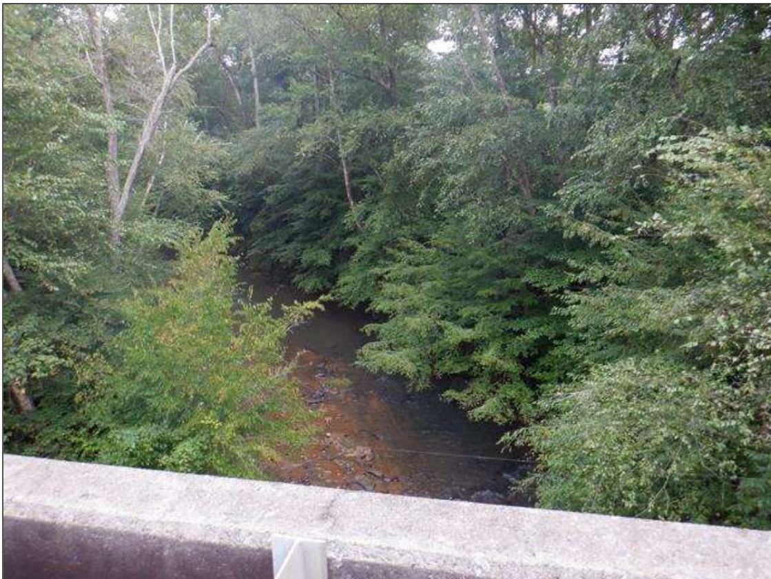
looking upstream [East] from bridge
