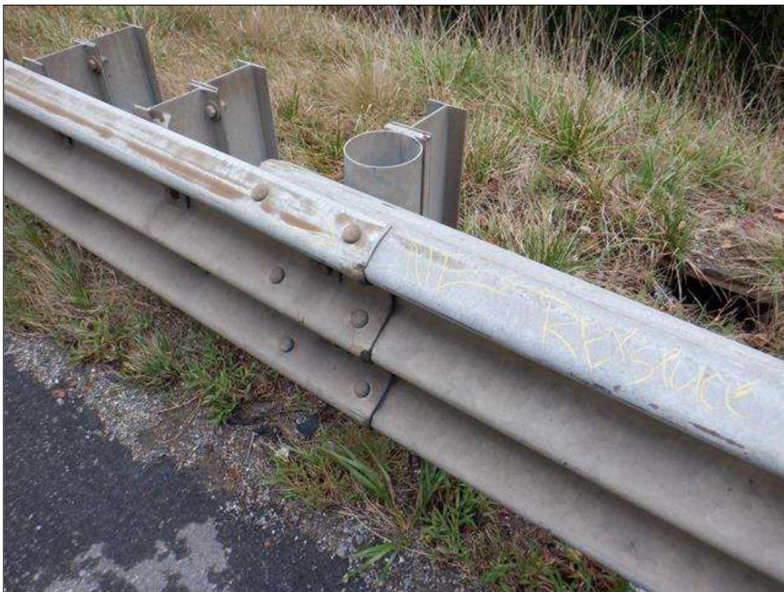
[PAR] splices at North approach slab, reversed and facing traffic
