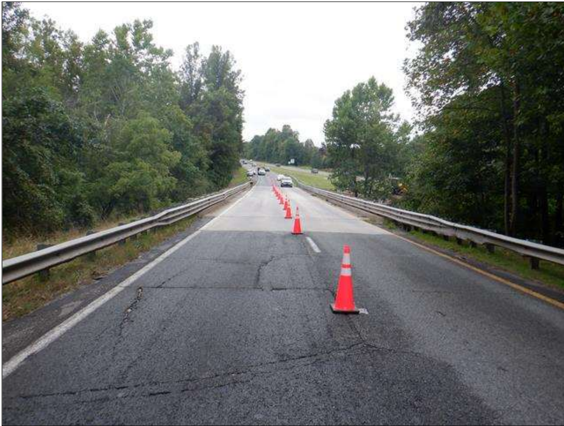
North approach looking South
