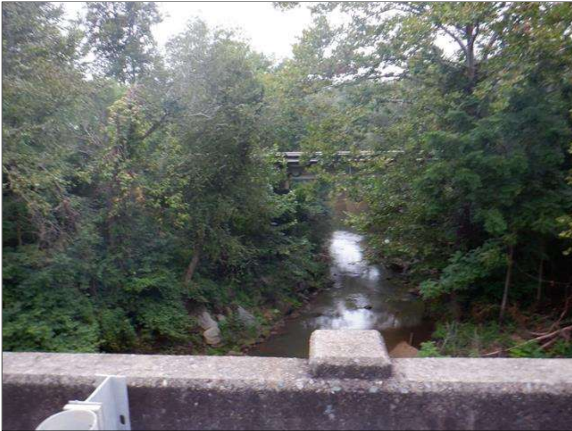
looking downstream [West] from bridge
