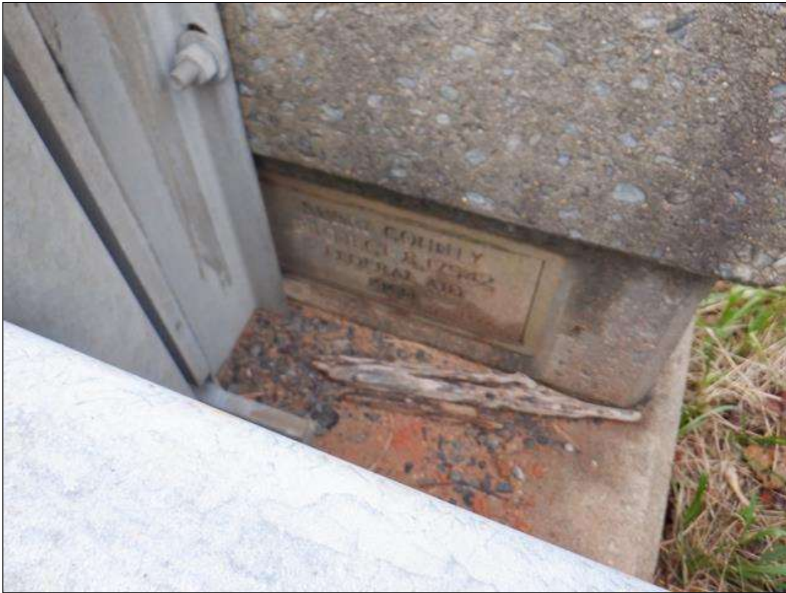
bridge plaque at Southeast corner
