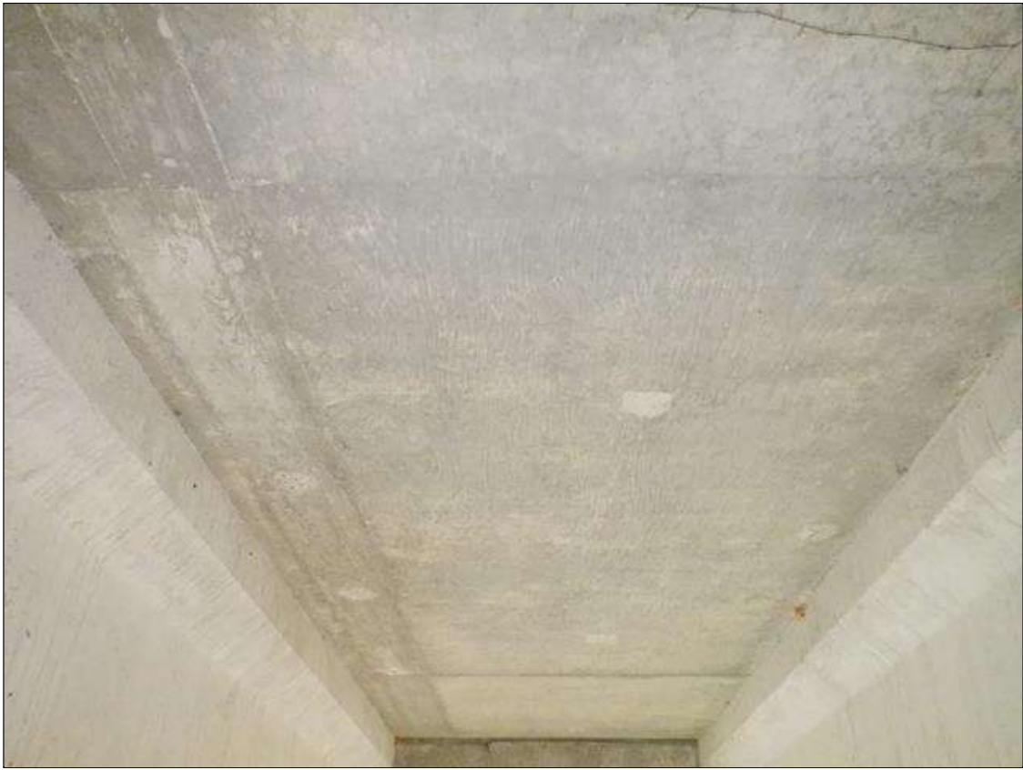
typical underside of deck
