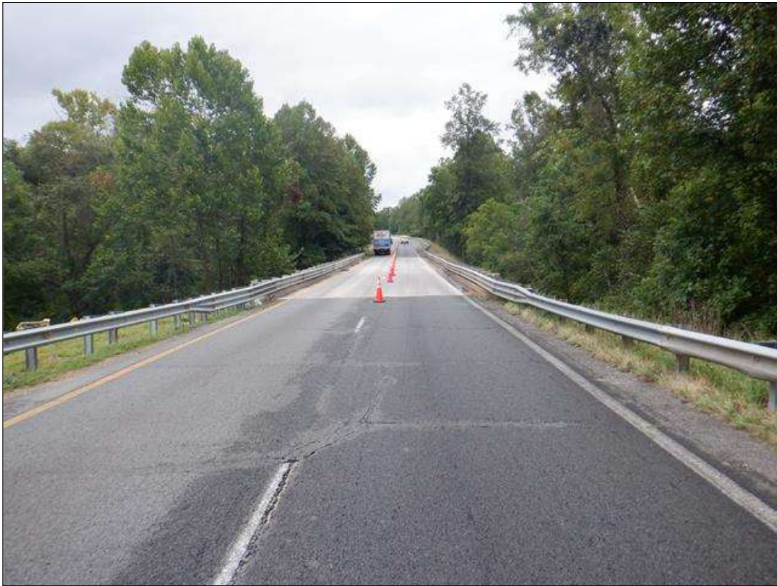
South approach looking North
