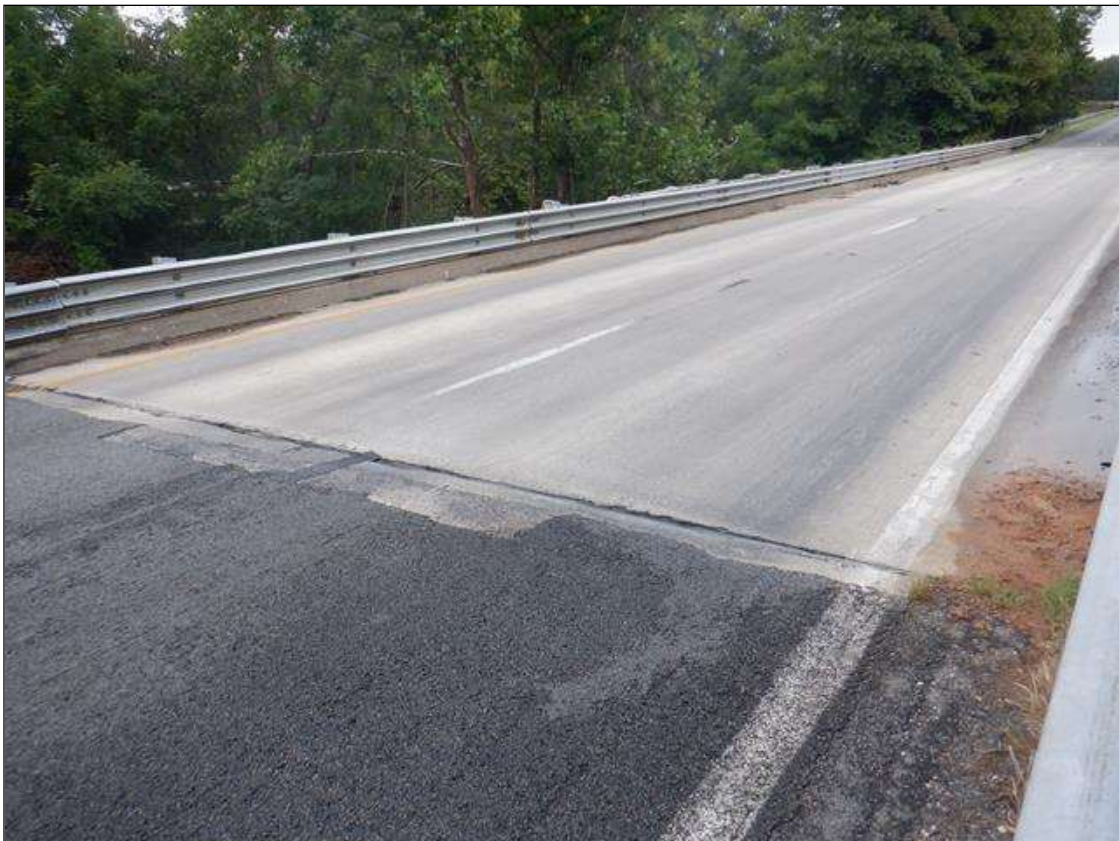
left bridge rail
