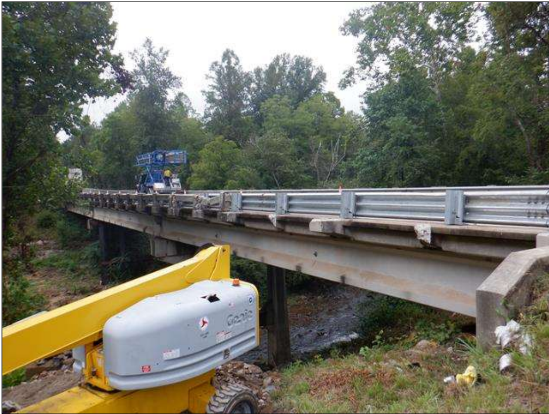
West profile looking East
