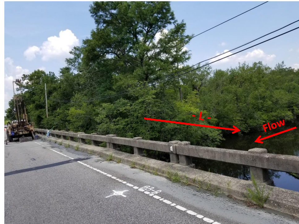
Photograph No. 1: View at existing Bent 3 looking northwest, drilling B2-B
