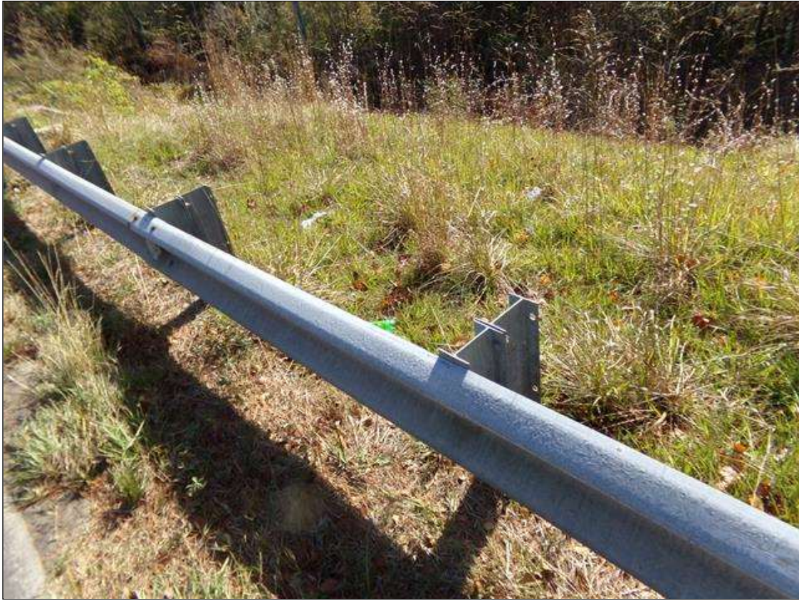
SOUTHWEST GUARDRAIL POST SPACING (SOUTHEAST CORNER SIMILAR)
