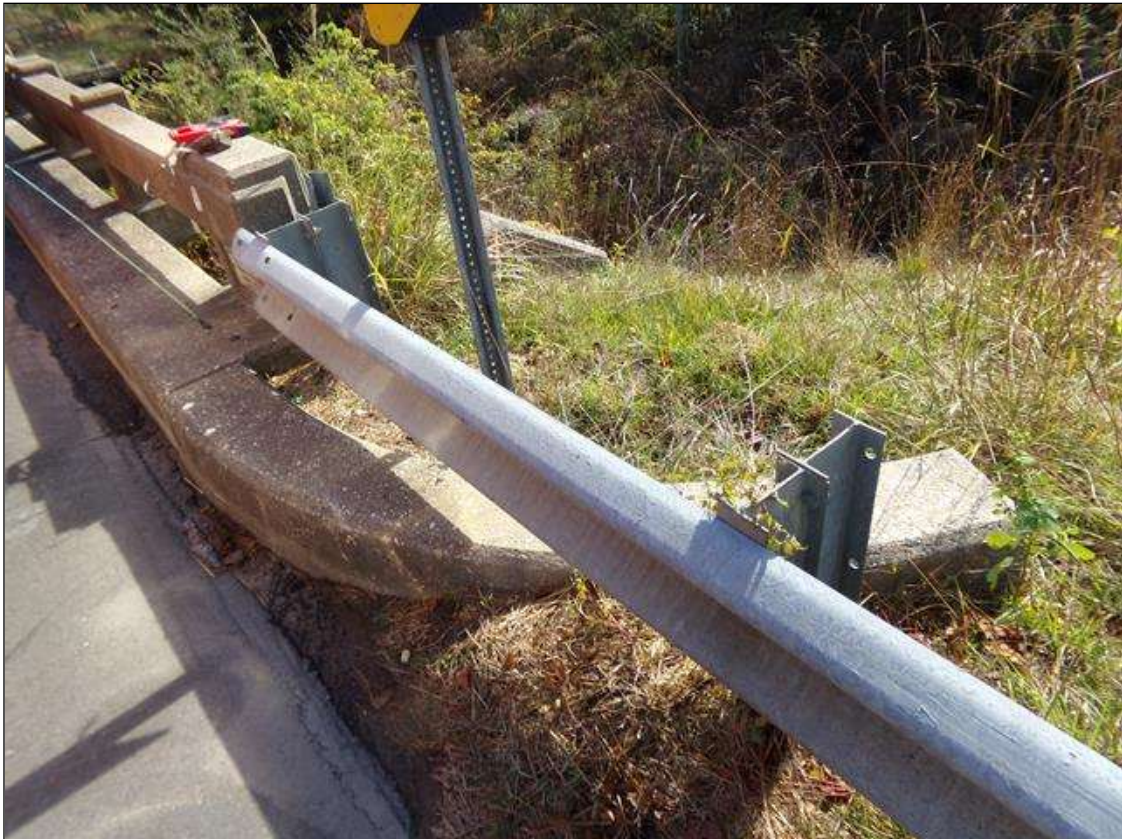
SOUTHWEST GUARDRAIL TRANSITION (SOUTHEAST CORNER SIMILAR)
