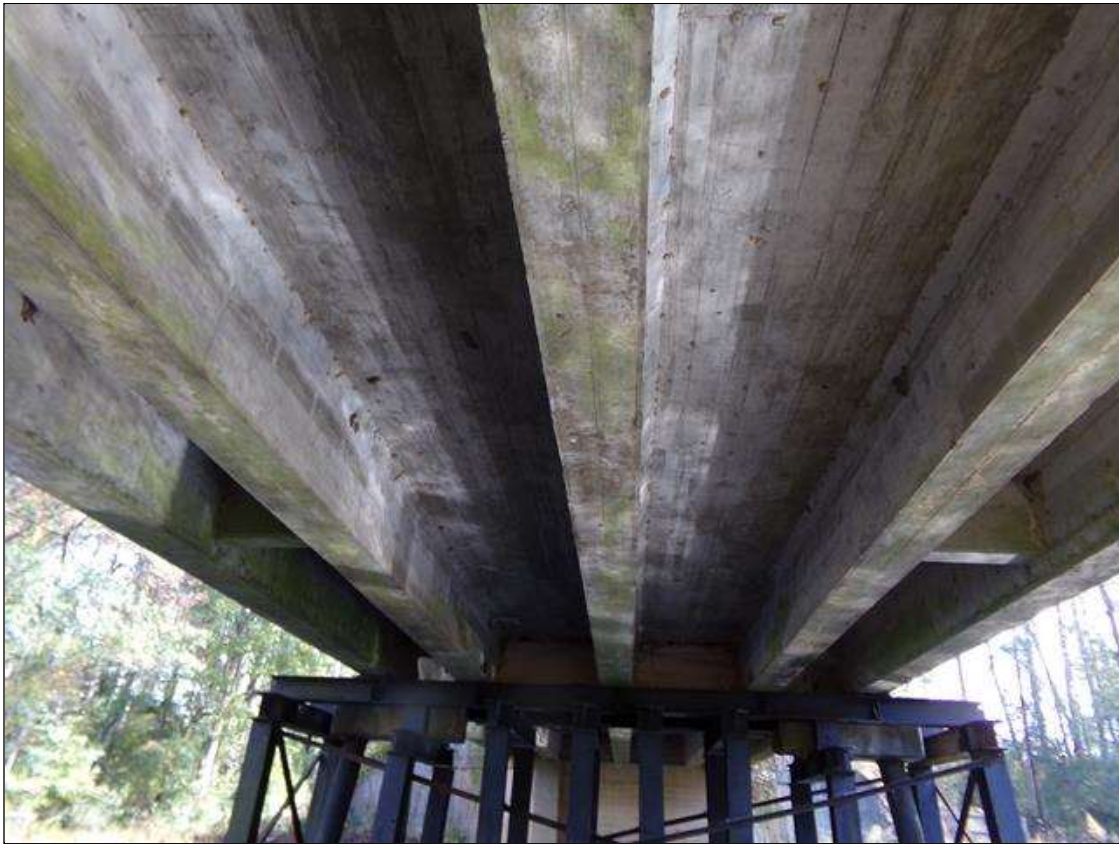
UNDERSIDE OF SUPERSTRUCTURE (SPAN 3 SHOWN)
