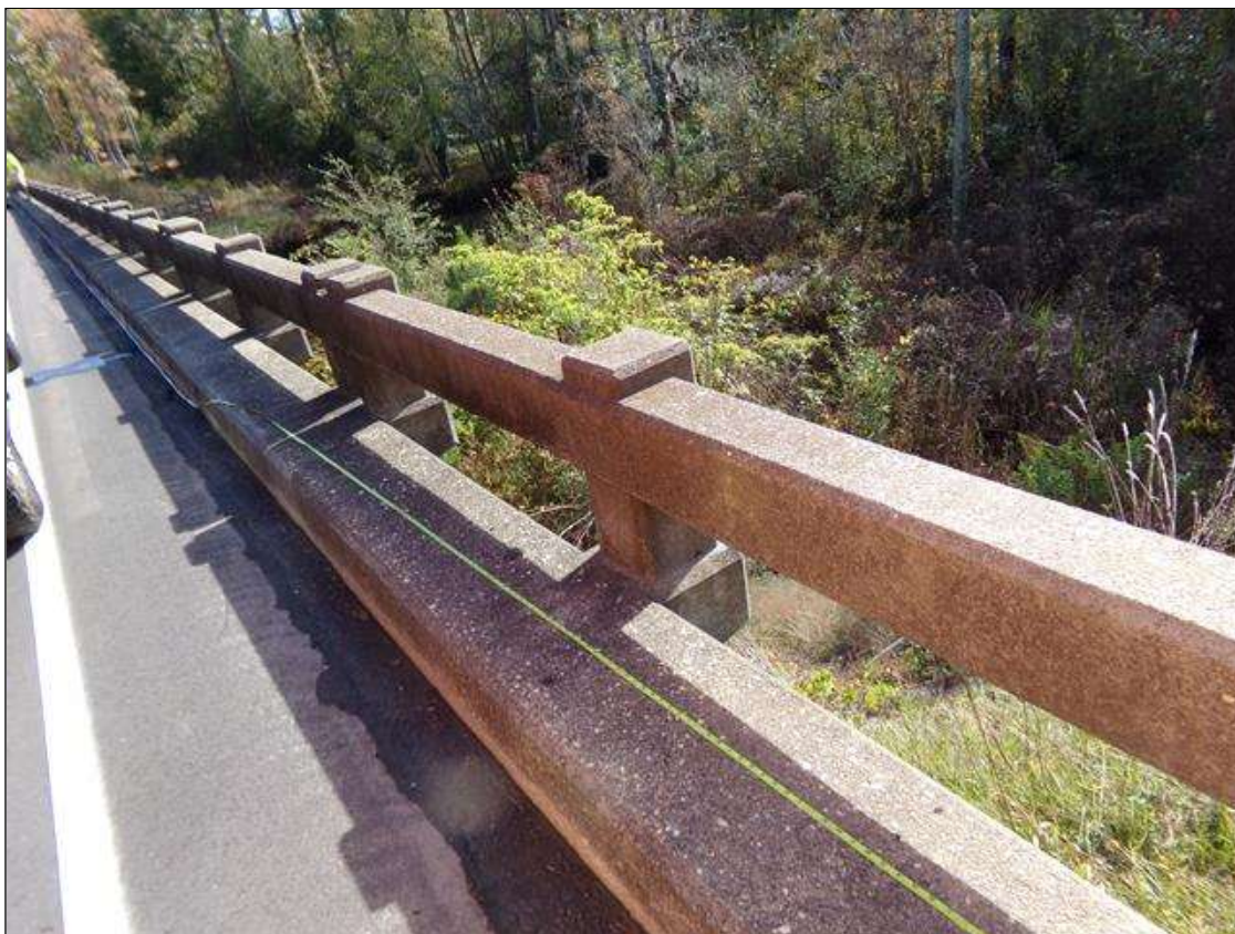
SOUTH BRIDGE RAIL (NORTH BRIDGE RAIL SIMILAR)
