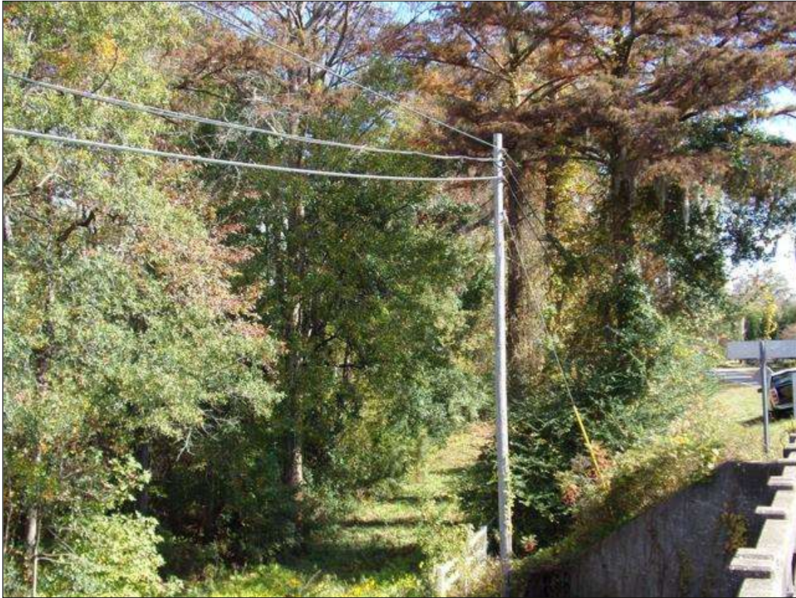
OVERHEAD UTILITIES ON NORTH SIDE OF BRIDGE (SOUTH SIDE SIMILAR)
