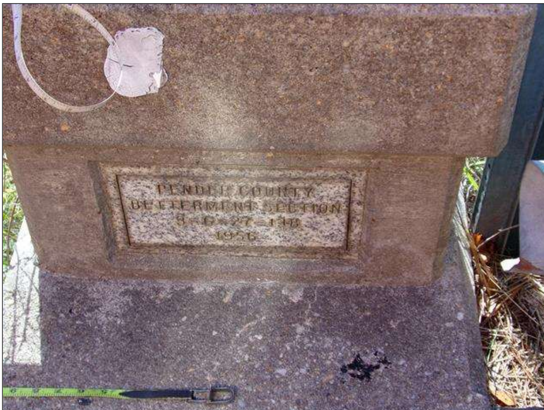
BRIDGE PLAQUE AT SOUTHWEST CORNER (NORTHEAST CORNER SIMILAR)
