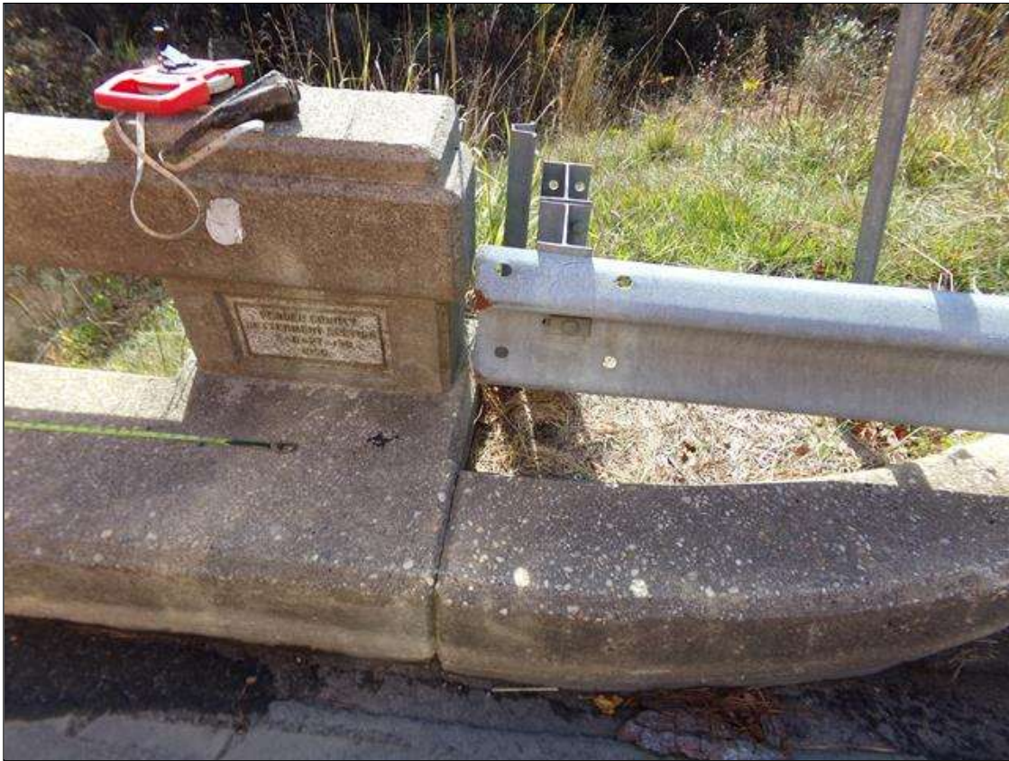
SOUTHWEST GUARDRAIL ATTACHMENT (SOUTHEAST CORNER SIMILAR)
