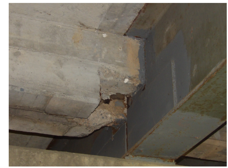
TYP. INTERIOR DIAPHRAGM REPAIR SITE
