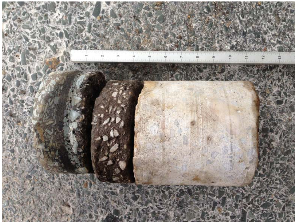
Exhibit A-22: Photograph of pavement core HA-05
