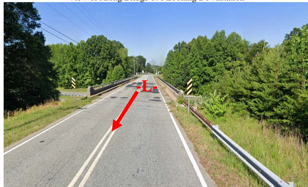
View of Along Bridge 170 Looking Downstation
