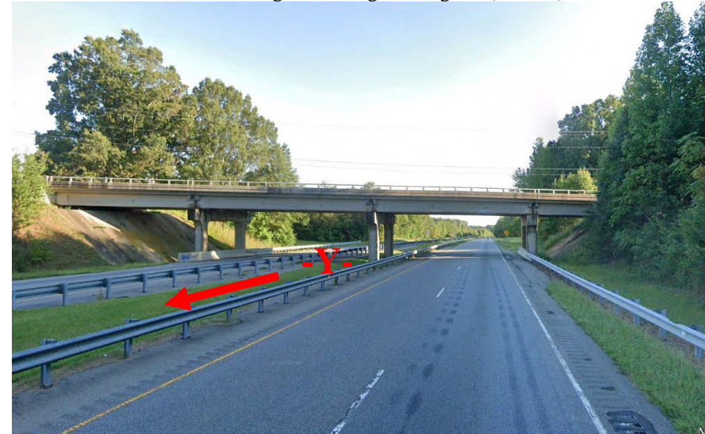
View Looking Left to Right Along -Y- (US 220)
