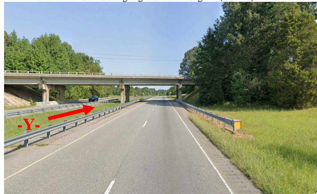
View Looking Right to Left Along -Y- (US 220)
