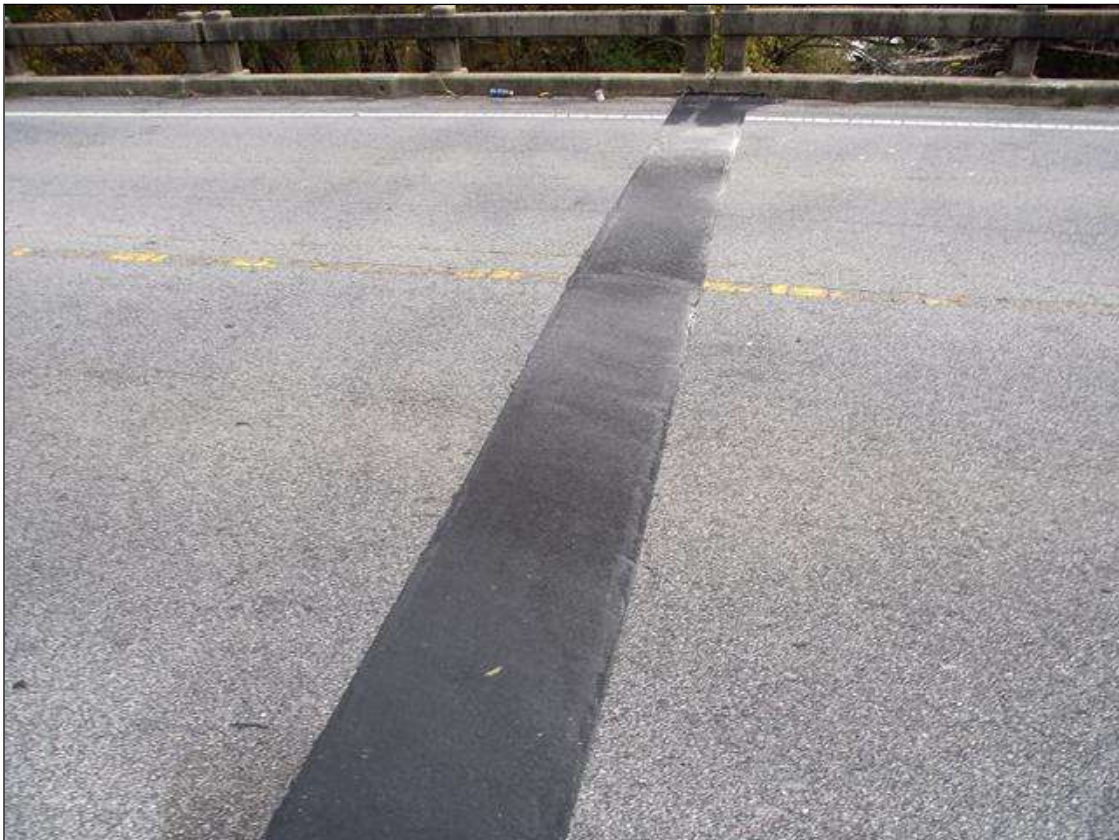
JOINT AT BENT 2
