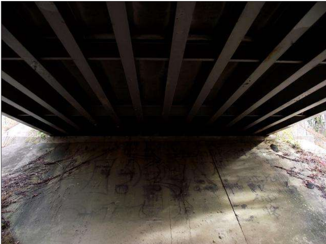
END BENT 2 OVERVIEW
