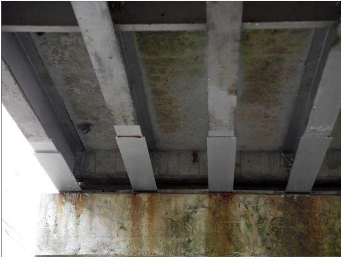
PLATE REPAIRS AT THE ENDS OF BEAMS 1-4 IN SPAN 1 OVER BENT 1
