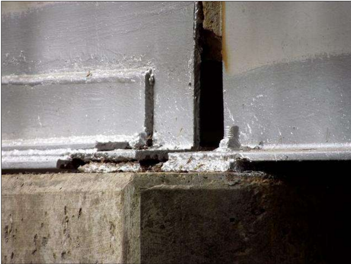
TYPICAL BEARING ASSEMBLY THROUGHOUT STRUCTURE
