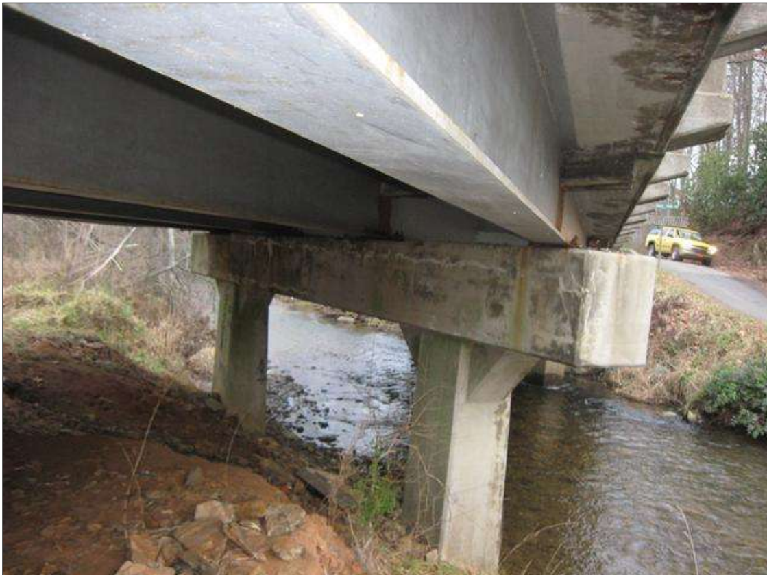
REP. OF INT. BENTS 1 AND 2. PHOTO WAS TAKEN OF INT. BENT 1.
