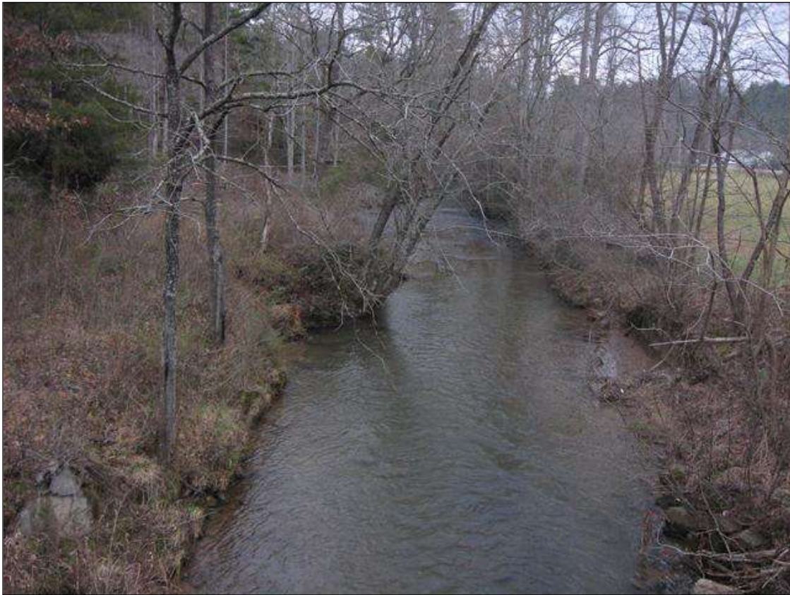
LOOKING DOWNSTREAM FROM TOP OF BRIDGE.
