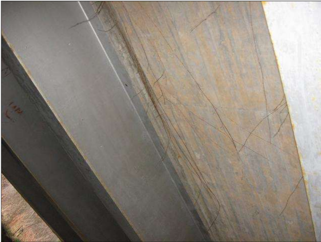
REP. OF UNDERSIDE FOR SPANS 1, 2, AND 3. PHOTO WAS TAKEN OF SPAN 1.
