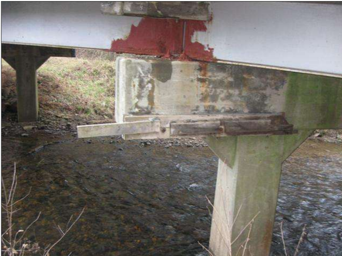
TEMP. REPAIR TO CAP INT. BENT 2.
