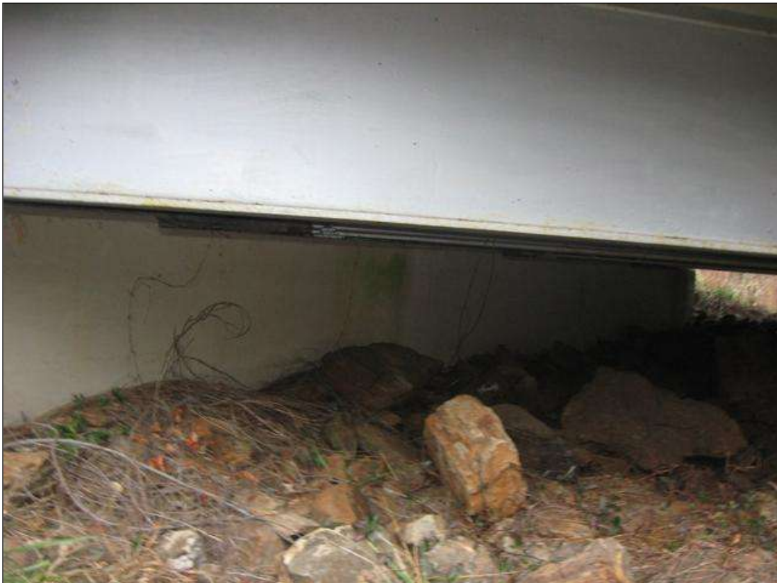
REP. OF END BENTS 1 AND 2. PHOTO WAS TAKEN OF END BENT 1.
