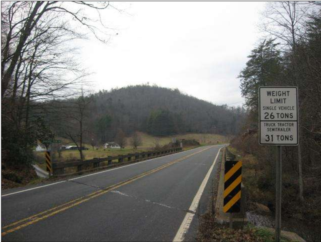
LOOKING SOUTH - BRIDGE IS POSTED SV 26 TTST 31 TONS.
