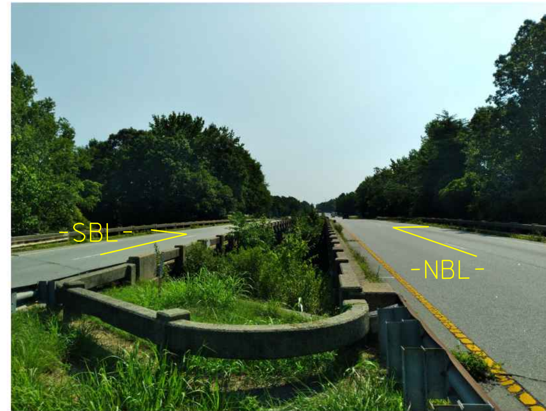
PHOTO #2: END BENT 1 OF EXISTING BRIDGES 164 AND 168 LOOKING EAST (UPSTATION)
