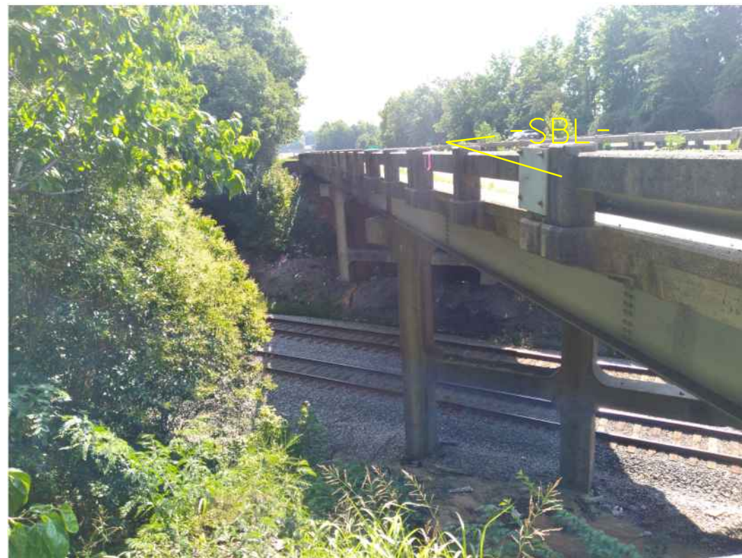
PHOTO #3: END BENT 1 OF EXISTING BRIDGE 168 LOOKING EAST (UPSTATION)
