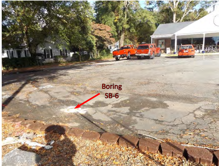
Photograph 8. GeoEnvironmental soil boring location U5873.2-SB-6.
