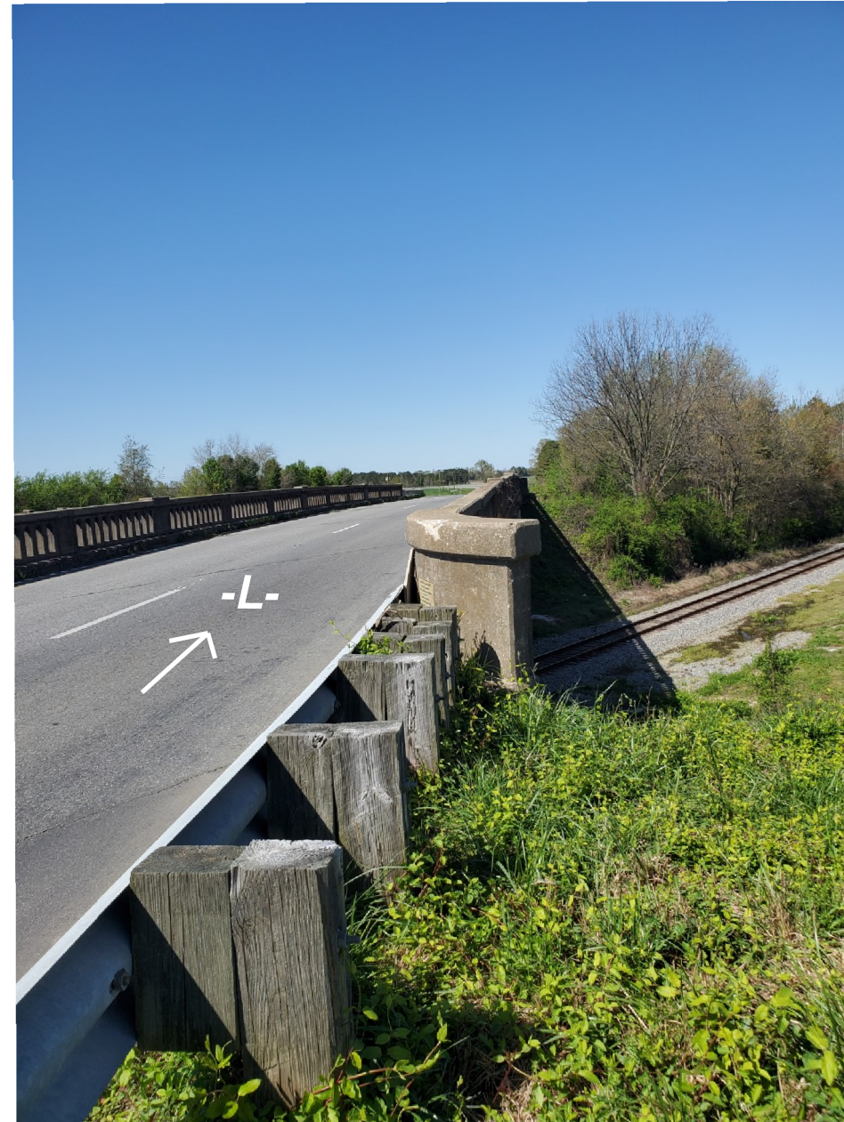
VIEW LOOKING NORTH
