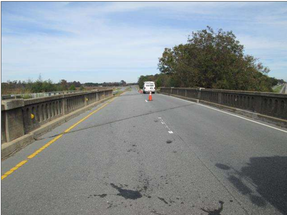
LOOKING NORTH FROM BRIDGE
