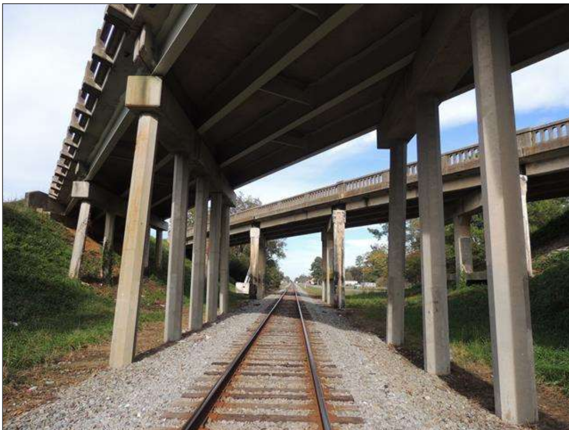
LOOKING EAST THROUGH SPAN 3
