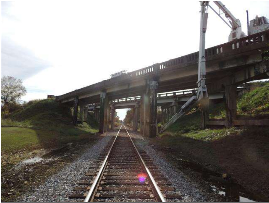
LOOKING WEST THROUGH SPAN 3
