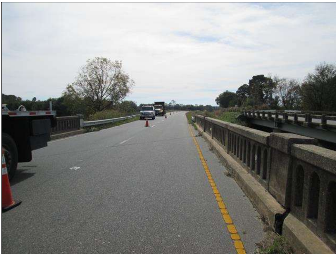
LOOKING SOUTH FROM BRIDGE
