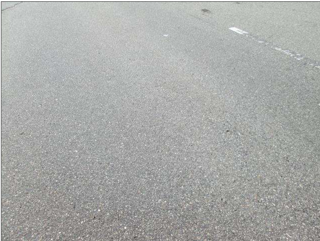
WEARING SURFACE SPAN 3 ( SIM. IN ALL SPANS )
