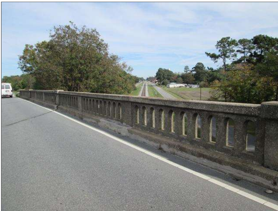
LOOKING EAST FROM BRIDGE
