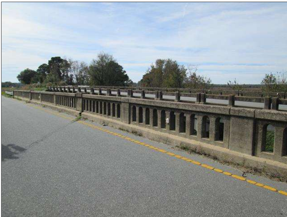
LOOKING WEST FROM BRIDGE
