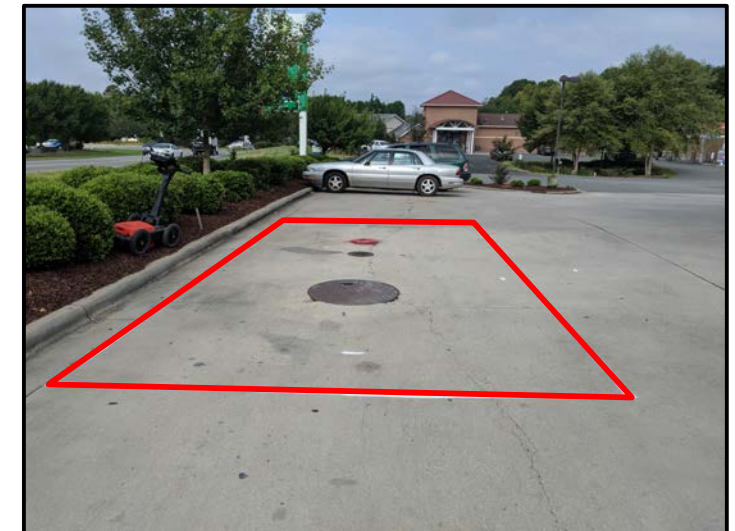
View of Known UST #1 Facing Approximately West
