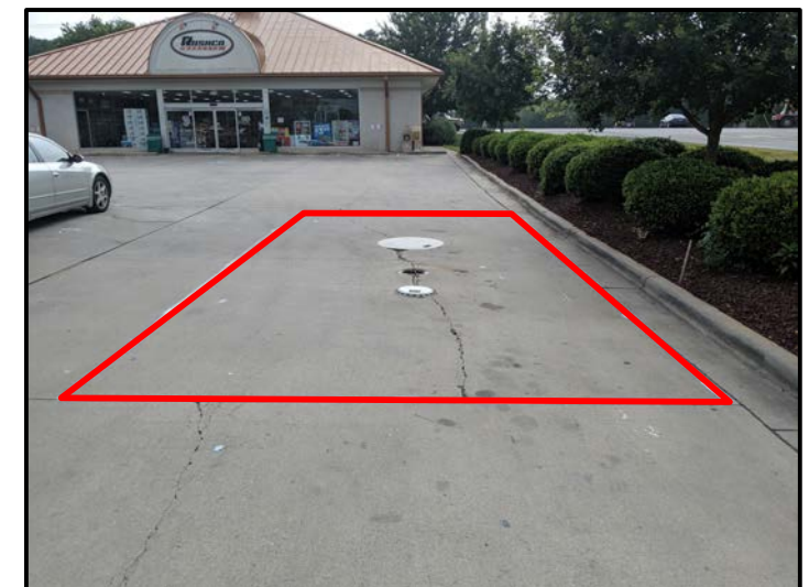
View of Known UST #2 Facing Approximately East
