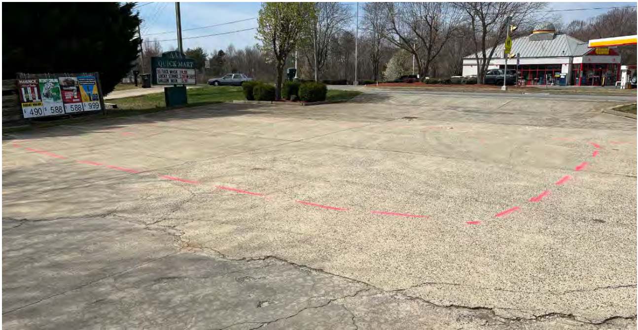
Photograph 2. Known abandoned UST Basin at the Quick Mart property.
