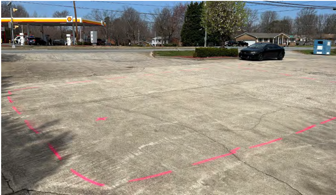
Photograph 3. Known abandoned UST Basin look toward former fuel dispensers at the Quick Mart property.
