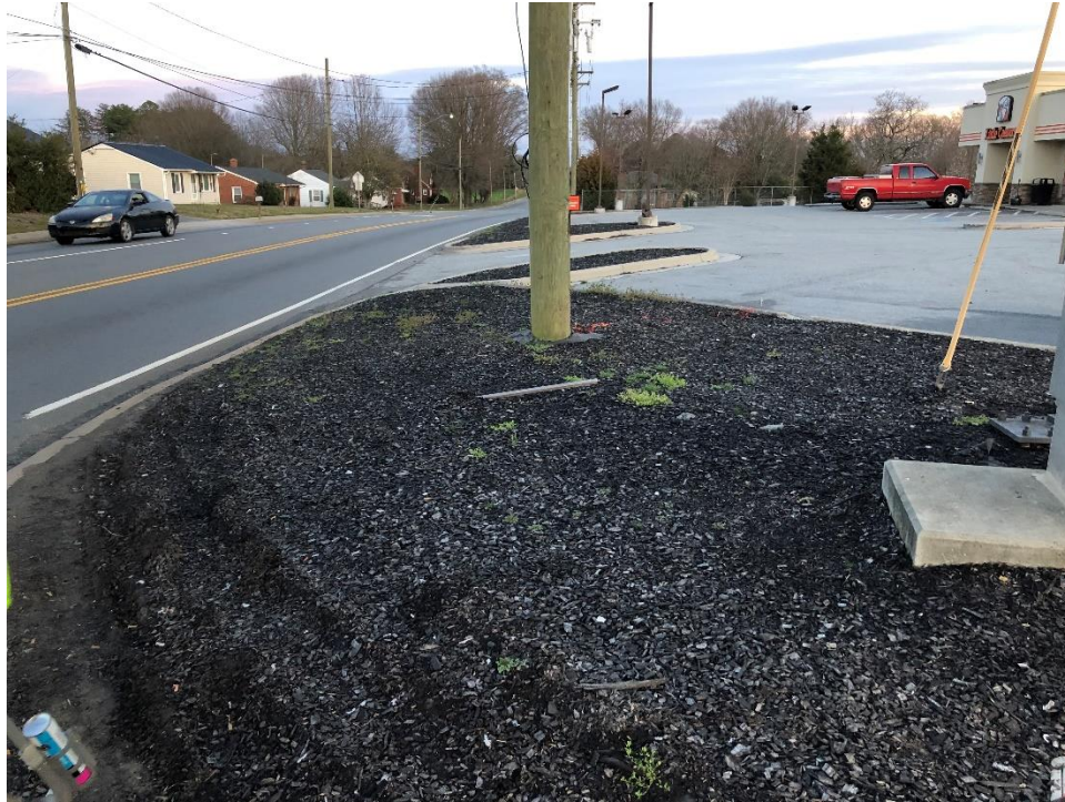
Photo 1: Looking southeast along Old Hollow Rd. project limits.
