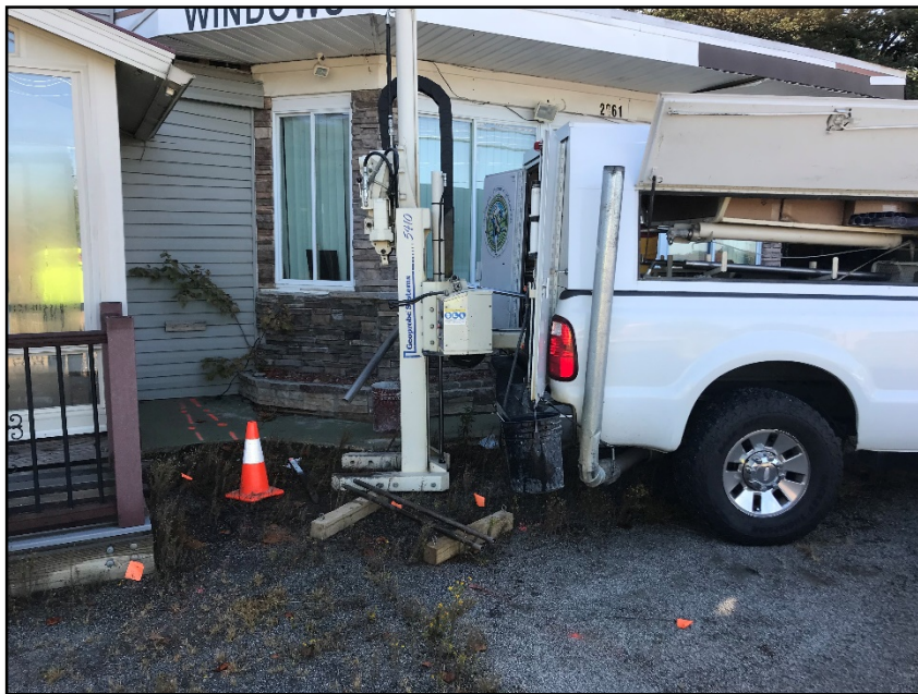
Photograph No. 2: General view of Boring B-16.
