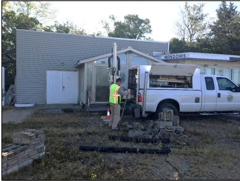
Photograph No. 1: General view of Boring B-15.
