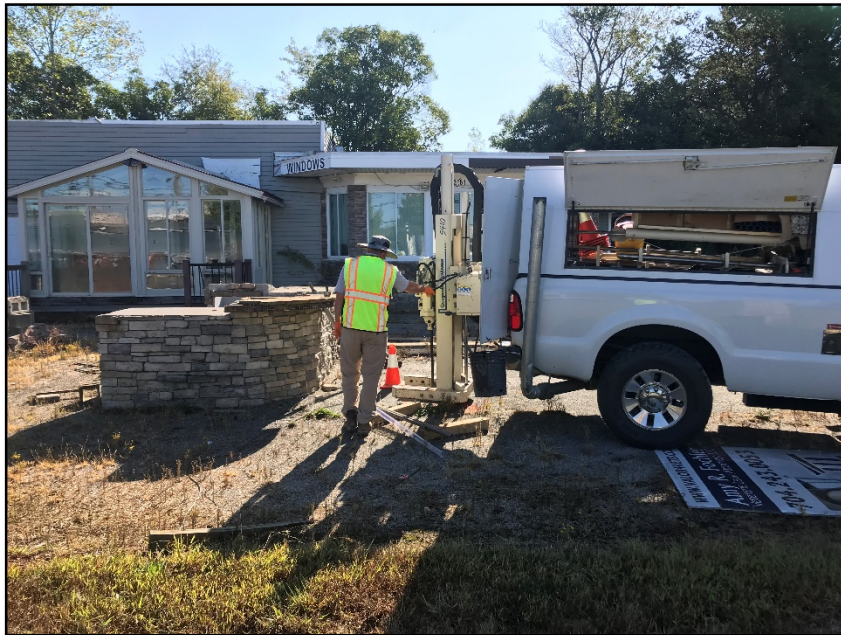
Photograph No. 4: General view of Boring B-18.
