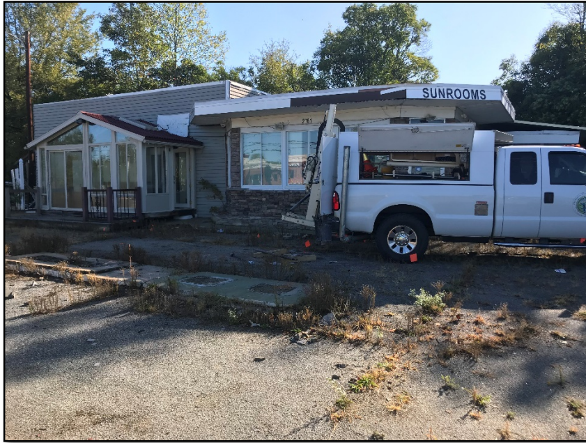
Photograph No. 3: General view of Boring B-17.
