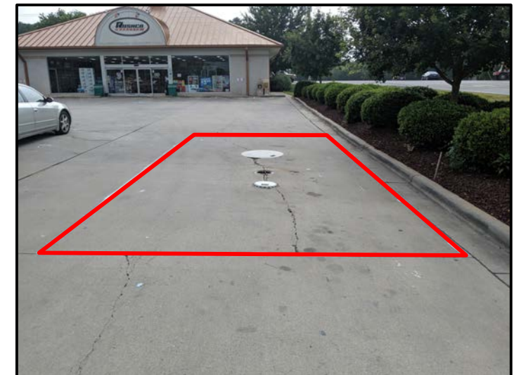
View of Known UST #2 Facing Approximately East
