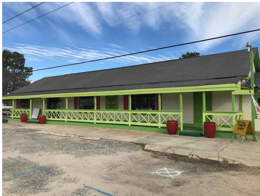
Photo #2 View of the on-site building (4798 NC-55); facing north.
