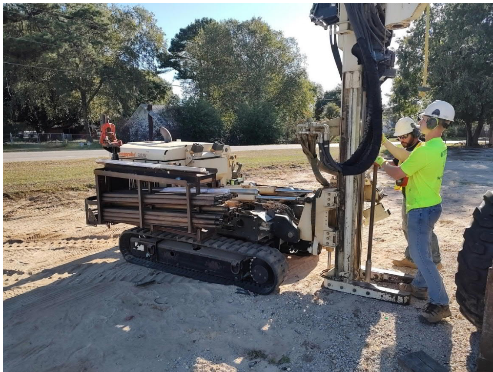
Photo 12 View of Quantex advancing soil boring; facing east.
