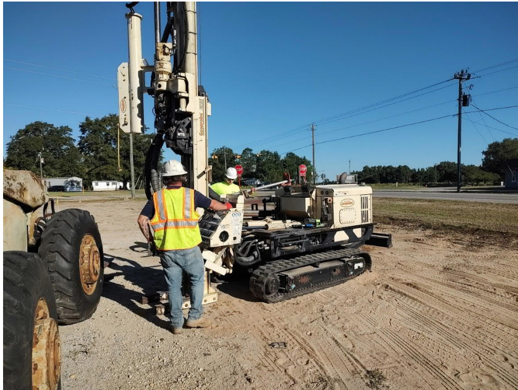
Photo 11 View of Quantex advancing soil boring; facing north.
