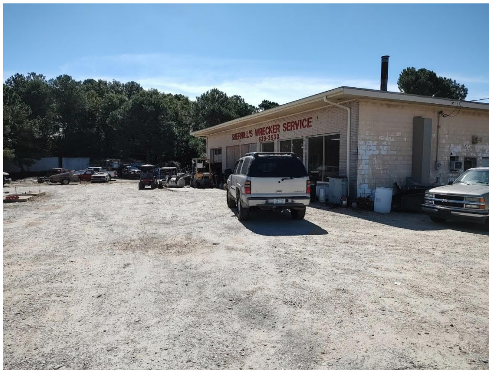
Photo 2 View of the site; facing south.
