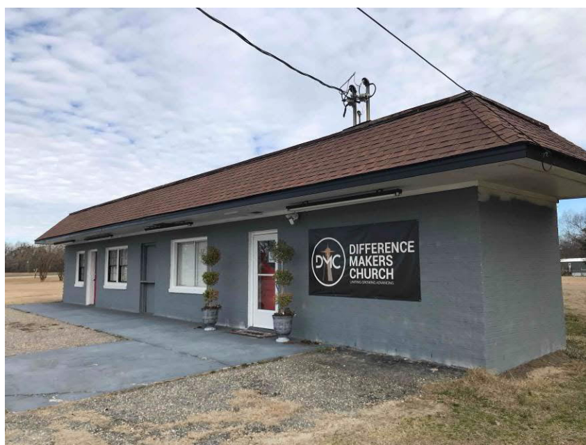
Photo #2 View of the on-site building; facing northeast.
