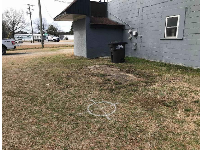
Photo #9 View of the confirmed grease trap and the apparent sanitary sewer line exit location from the building (in between the window and electricity meter) located on the south side of the on-site building; facing west.
