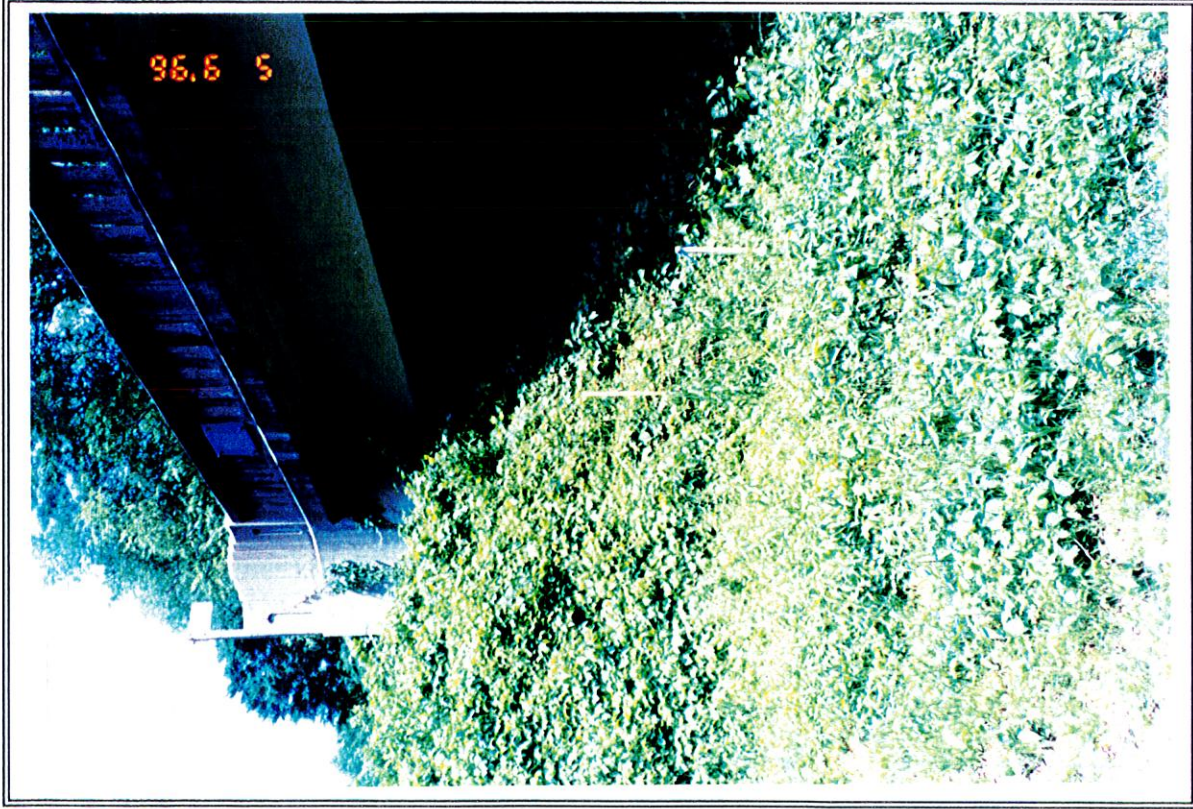
PHOTO NO. 9 - SBLEB2-A looking northeast toward End Bent Two. Stake at toe of slope indicates offset location of borehole
