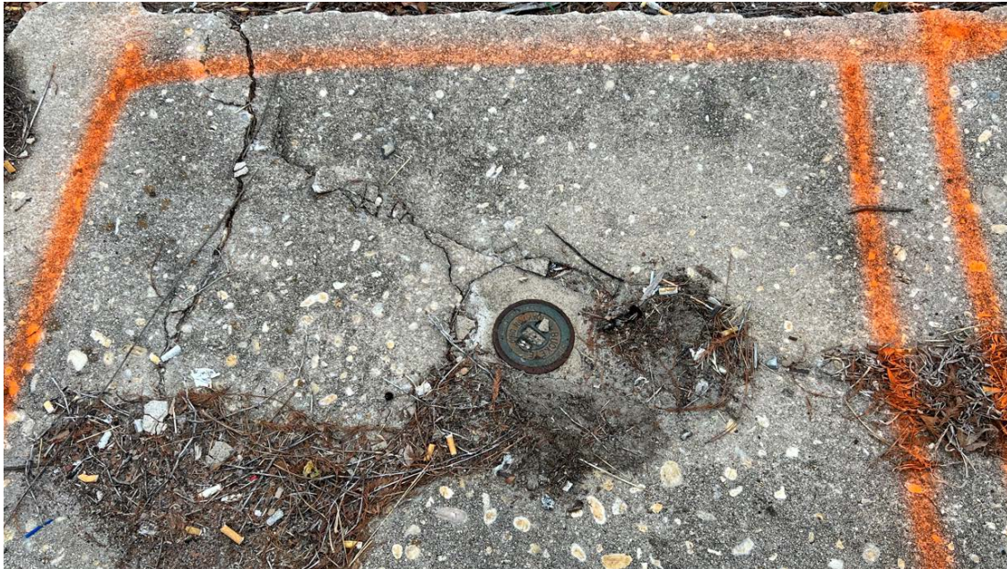
Photograph 2. Fill port visible at the surface.
