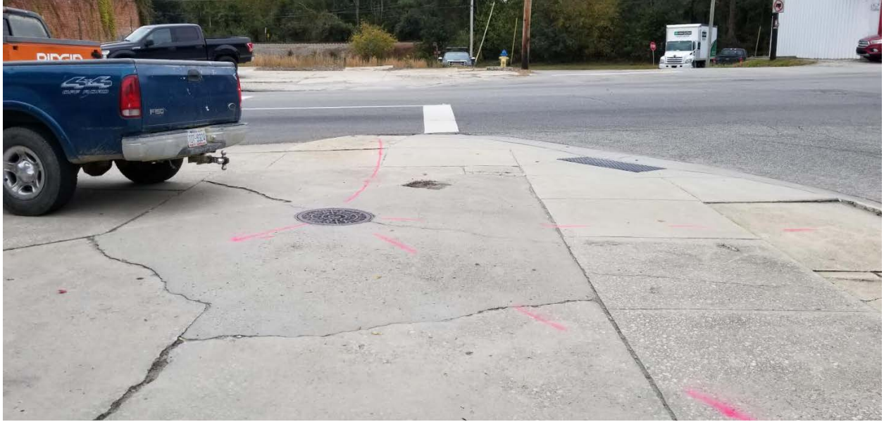
Photograph 5. Parcel 006 area of reinforced concrete, subsurface piping, storm drain, and manhole.
