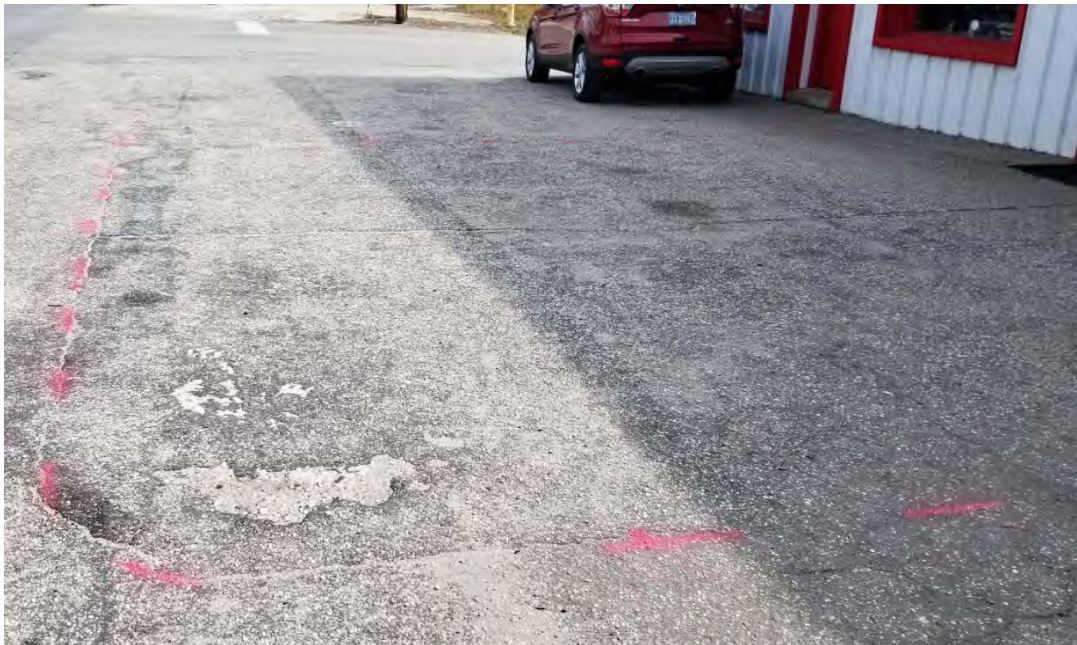
Photograph 2. Parcel 005 area of suspected reinforced concrete slab.
